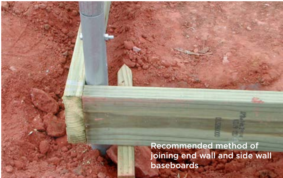
Installing baseboard to end wall posts using wood screws
