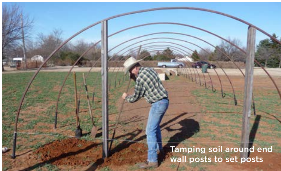
Anchoring end wall posts in concrete
