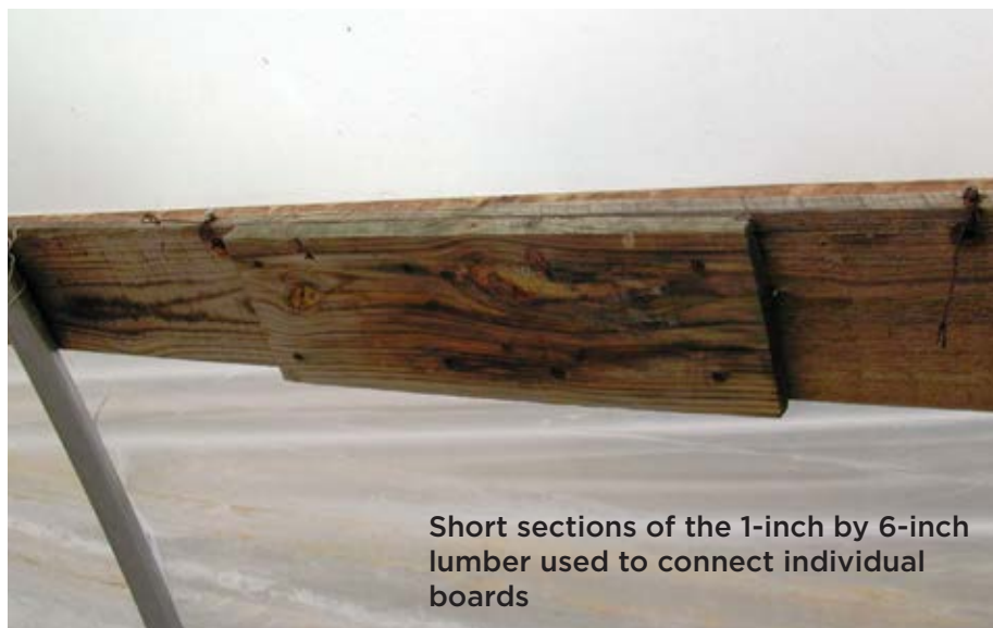
A hip-board fabricated using treated 1-inch by 6-inch lumber
