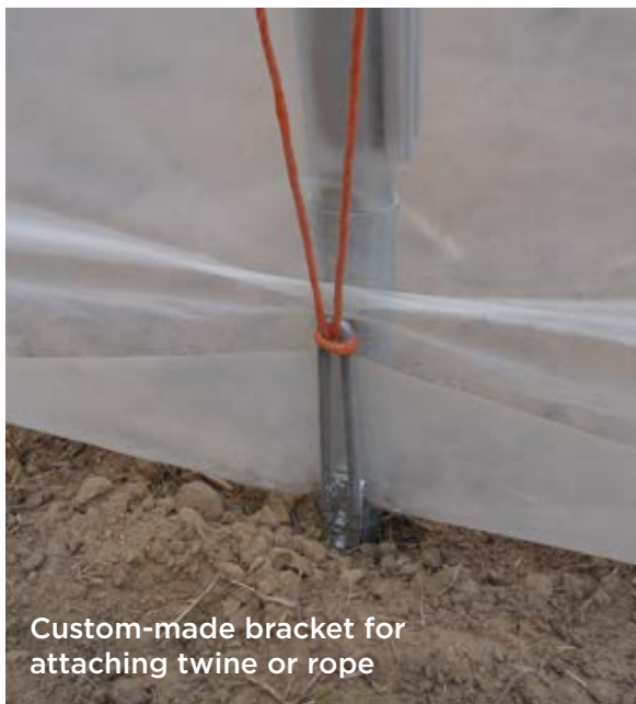
Use of heavyweight baling twine to fasten poly cover to frame. Notice the placement of the rope on either side of the hoop.
