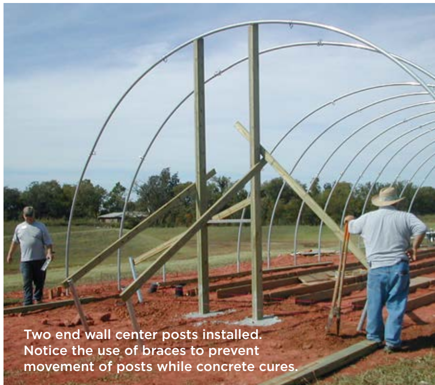
Use a string line attached to opposite ground posts to align end wall posts. A carpenter's level is needed when setting posts to ensure they are installed plumb.
