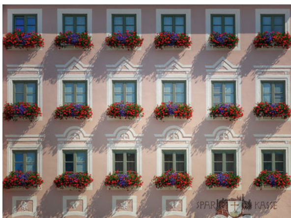
Fig. 2.9 This close-order setting has 3 rows and 6 windows per row (6 columns). (Photo by Albrecht Fietz from Pixabay, Landsberg am Lech (Germany) 2016; id 3240939)
