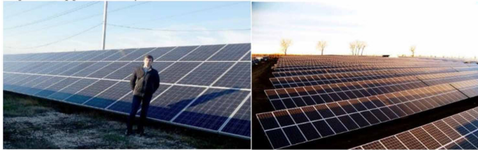
Figure 2. Shading of photovoltaic modules in solar power plants
