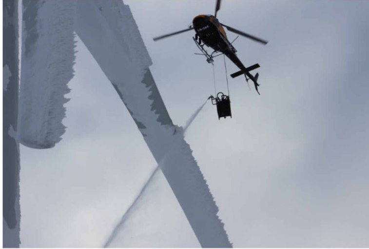
Figure 2. Fighting the icing of wind turbine blades with a helicopter (Nilsen, 2015)
