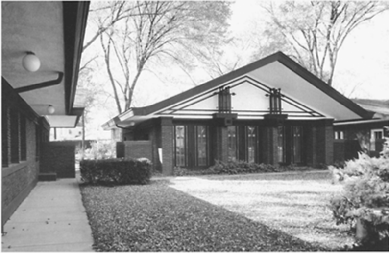
Babson Stable and Service building, inner court showing east elevation of garage Riverside, Illinois (c. 1916 additions and alterations to the 1908 original Babson House by Louis Sullivan)
