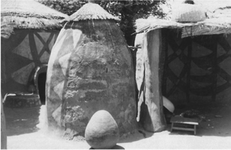
Earth-molded, nontrabeated structures, including granary, shade shelter, and living unit from Gurunsi culture, northern Ghana
