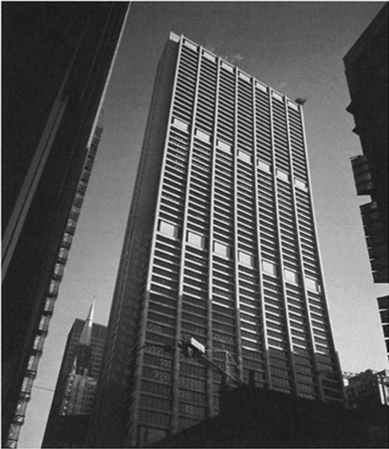
First National Bank of Chicago, designed by Perkins and Will (with C.F.Murphy Associates), 1966
