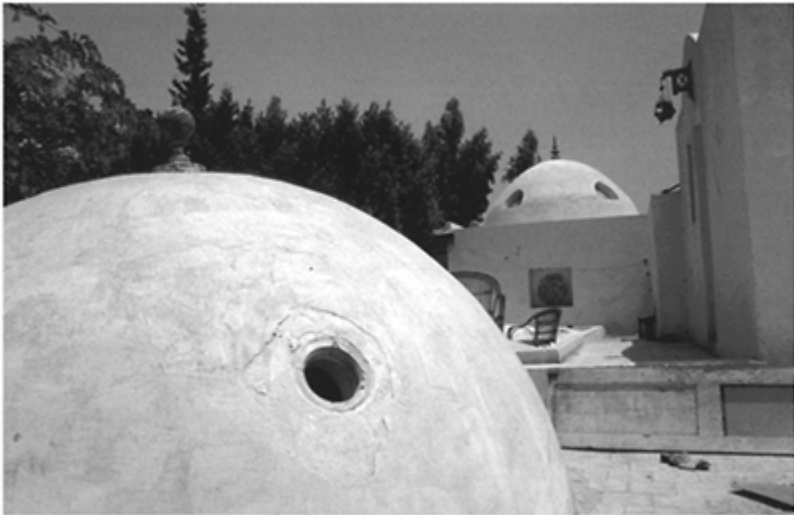
El-Dar Restaurant, view from the roof showing its mud-brick dome
