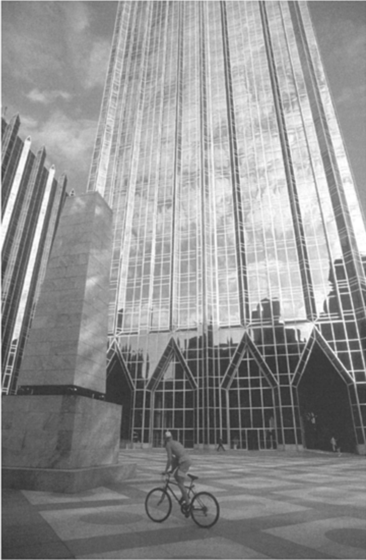
Plaza and PPG Place Skyscraper (formerly Pittsburgh Plate Glass Company, PPG Industries, Inc.), Philip Johnson and John Burgee (1979–84)
