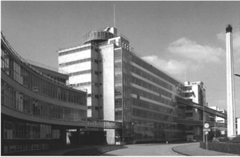
Van Nelle Factory, Rotterdam (1928), by Johannes A. Brinkman and L.C. van der Vlugt
