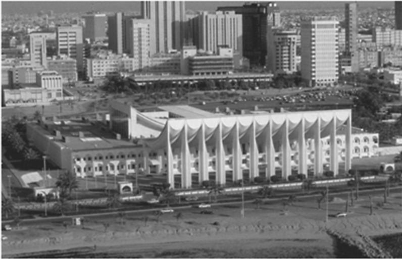
National Assembly Building (1983), Kuwait City, Kuwait
