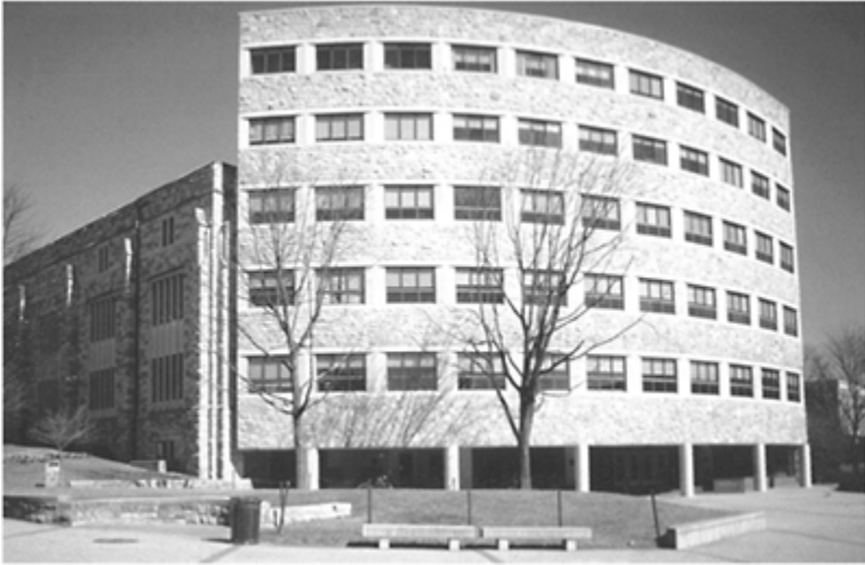
Carol M. Newman Library Renovation and Addition, Virginia Polytechnic Institute and State University (1971)
