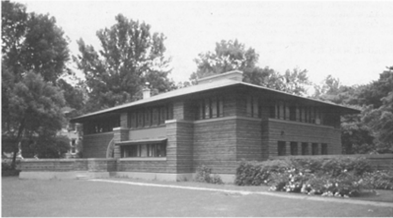
Arthur Heurtley House, Oak Park, Illinois, designed by Frank Lloyd Wright (1902)
