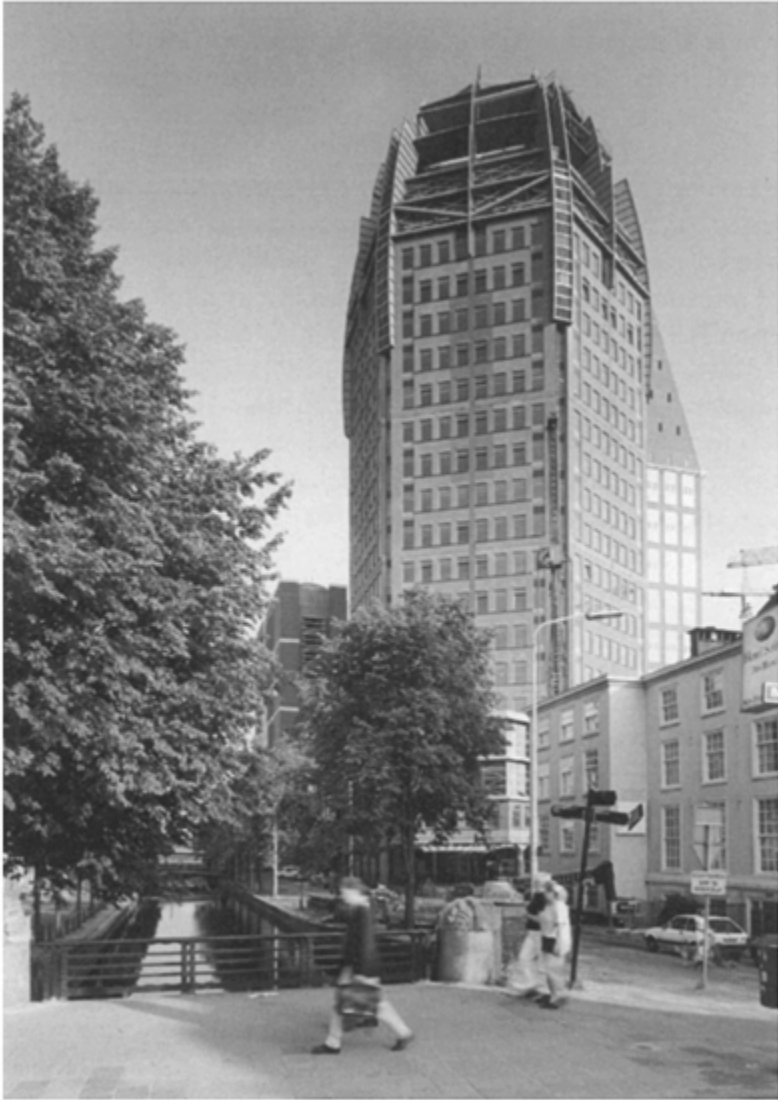
Zurich Tower, The Hague, the Netherlands (1999)
