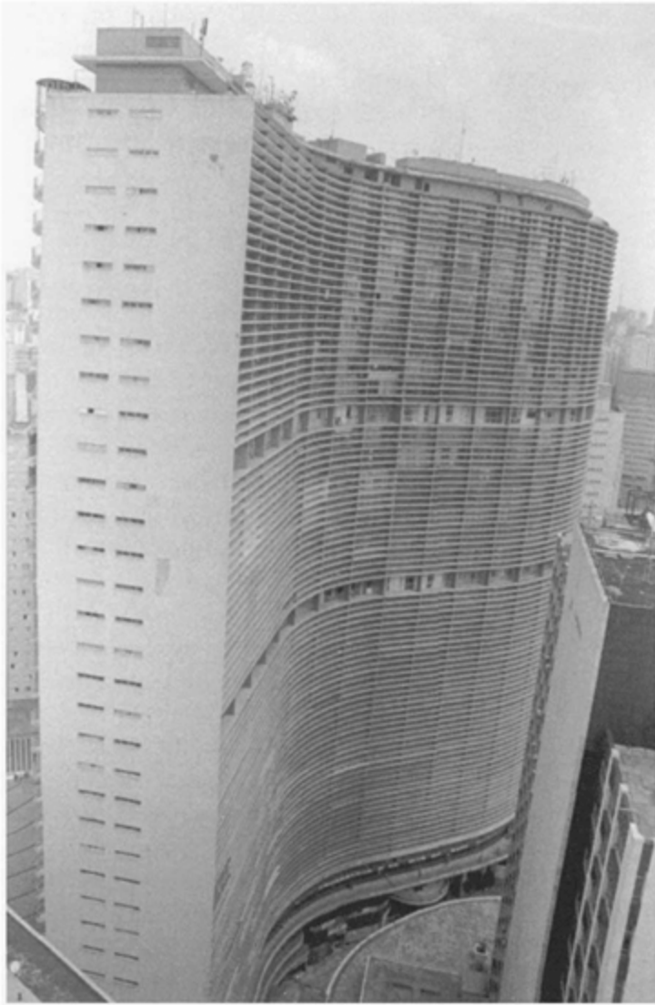
Copan Building (1957) designed by Oscar Niemeyer
