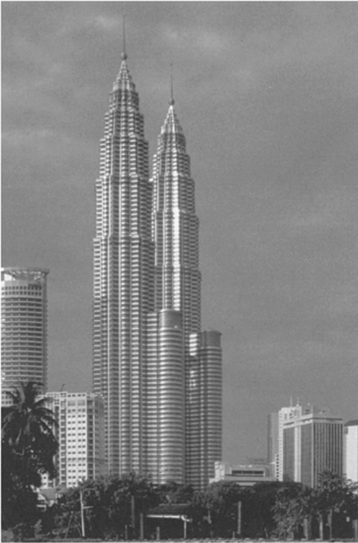
Petronas Office Towers, designed by Cesar Pelli
