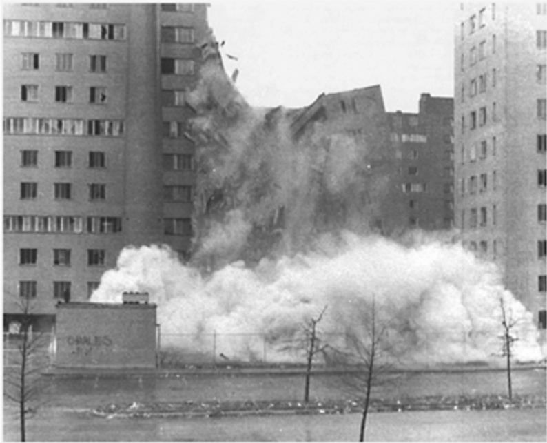
Pruitt Igoe Housing Project, designed by Minoru Yamasaki, April 21, 1972 demolition
