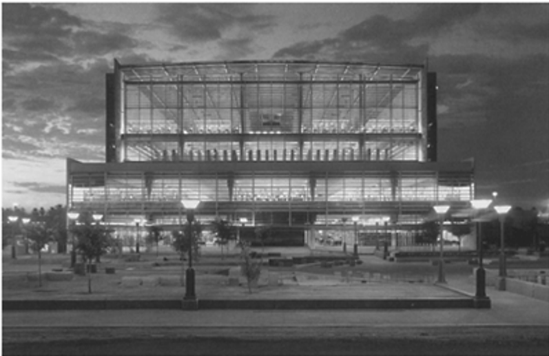
Phoenix Central Library (1995), South elevation
