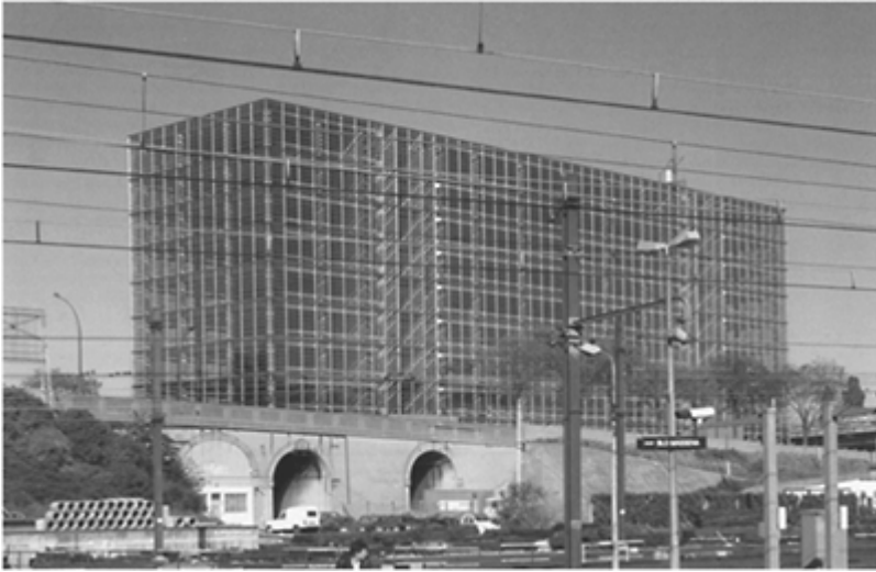
Hotel Industriel Berlier, Paris, designed by Dominique Perrault and Partners (1990)
