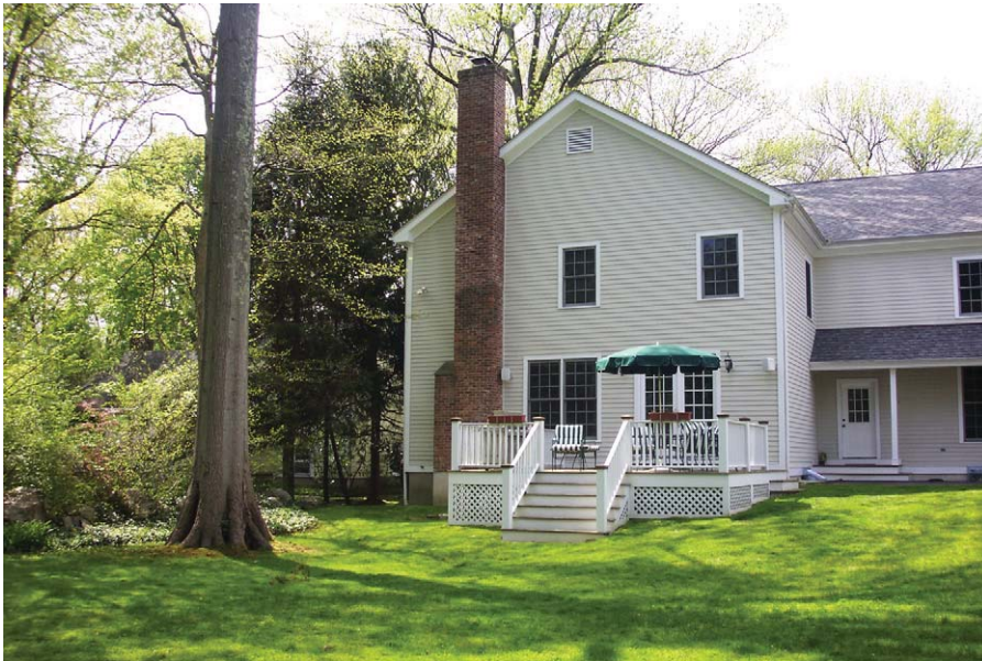
A typical North American home, built largely from wood (apart from the foundations and fireplaces/chimneys). Region of Greenwich, CT, USA (41 02 20.00 N 73 36 48.90 W).
