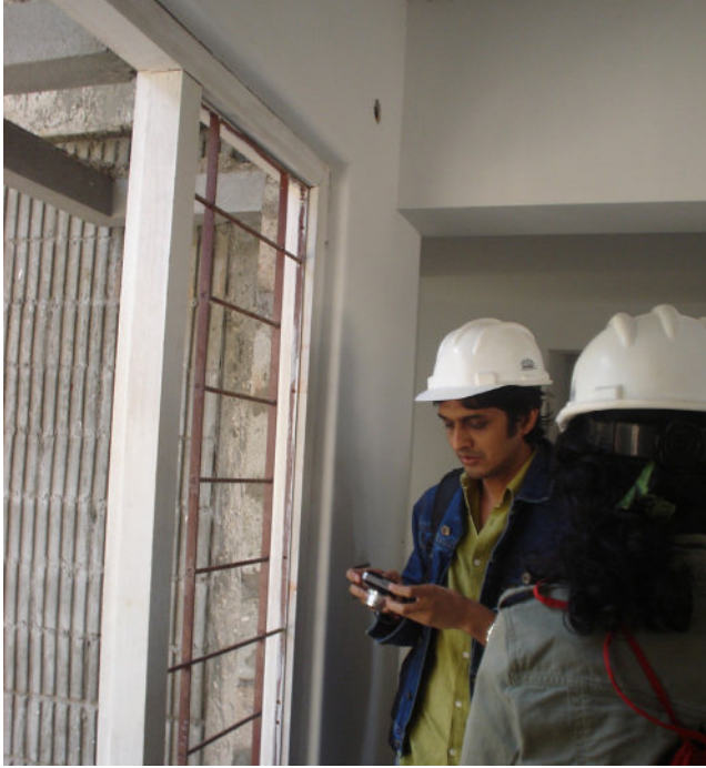
FIGURE 12. RSIEA students exploring new construction in one of BCIL's housing developments outside of Bangalore. Photo by the author.
