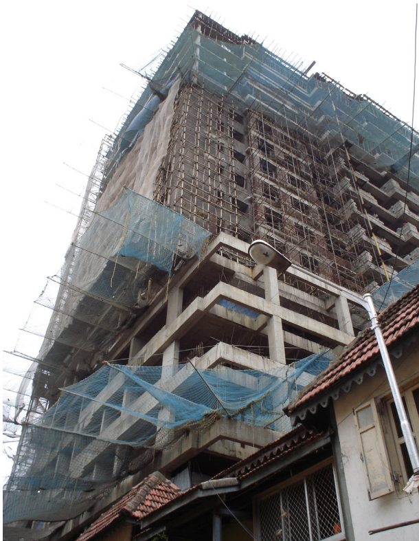
FIGURE 1. Construction in Mumbai, 2012. Photo by the author.
