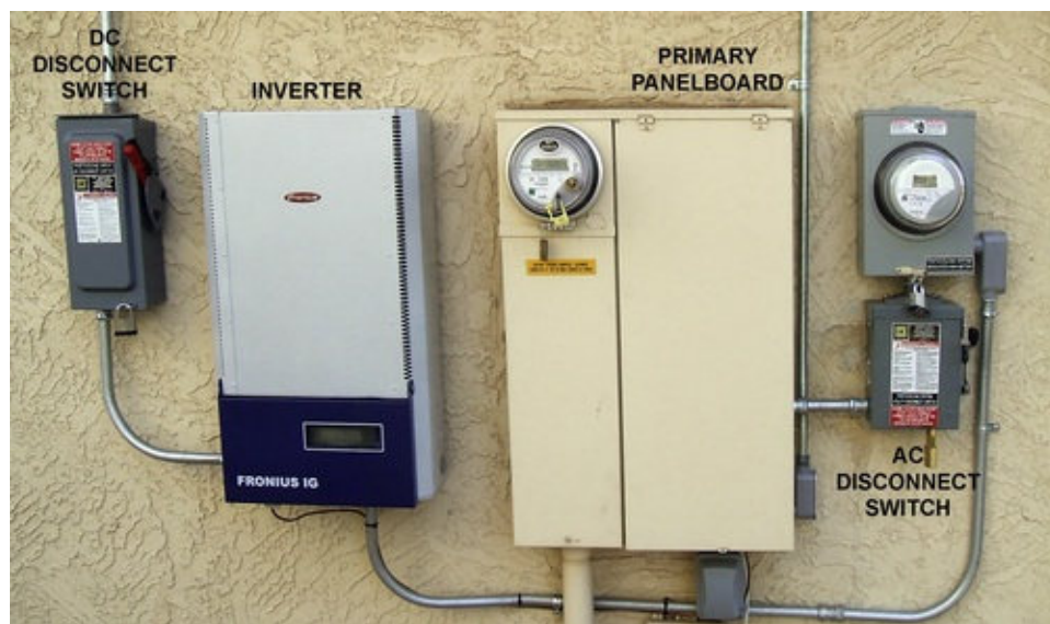
FIGURE 5.5 DC/AC Disconnect Arrangement. Courtesy of www.DreamHomeConsultants.com . (For color version of this figure, the reader is referred to the online version of this book.)
