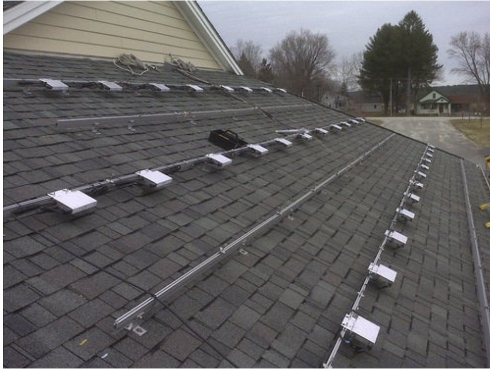
FIGURE 5.7 Microinverters and mounting system for PV modules. Photo courtesy of ReVision Energy Corp. (For color version of this figure, the reader is referred to the online version of this book.)
