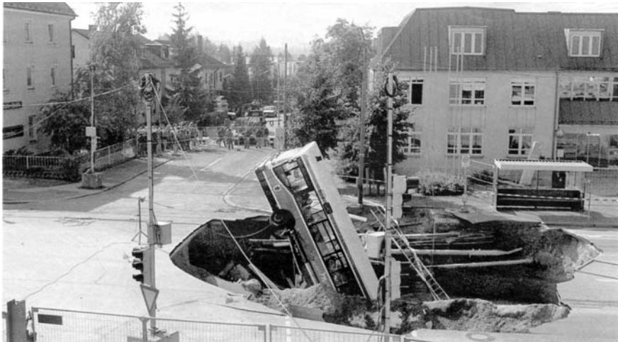
Fig. 1. Munich Trudering collapse, Subway line 2 - East Section 2 [9]
