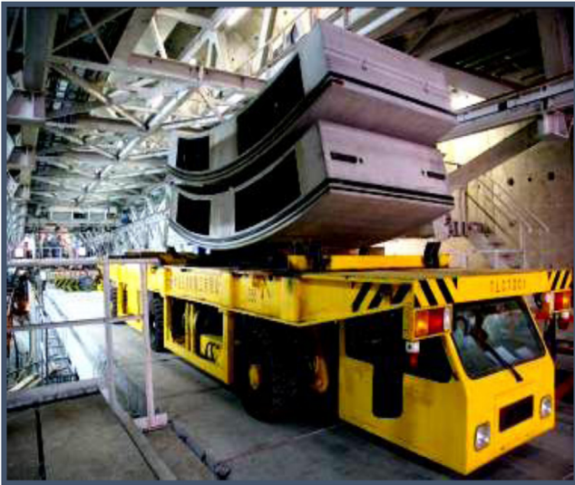
Figure 4.58 Transportation of segments within the tunnel.
