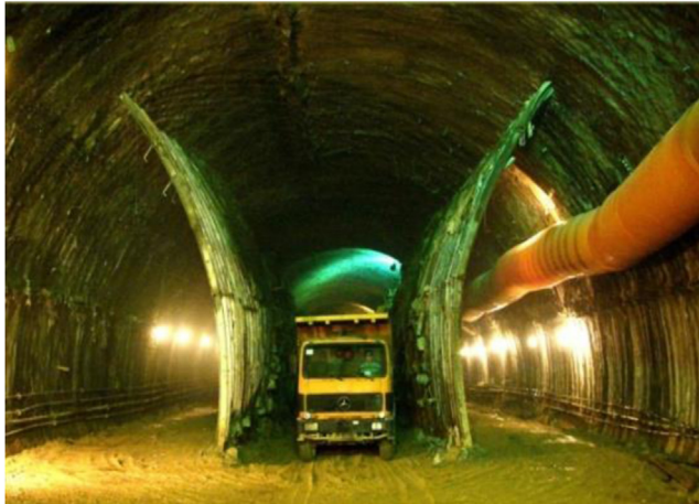
Figure 4.34 Xiangnan tunnel under construction.
