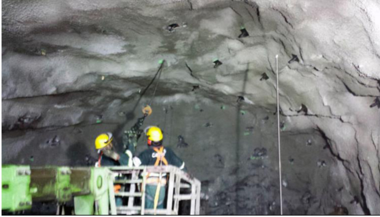
Figure 4.35 Rock bolt installation (Dywidag-Systems International, 2014).
