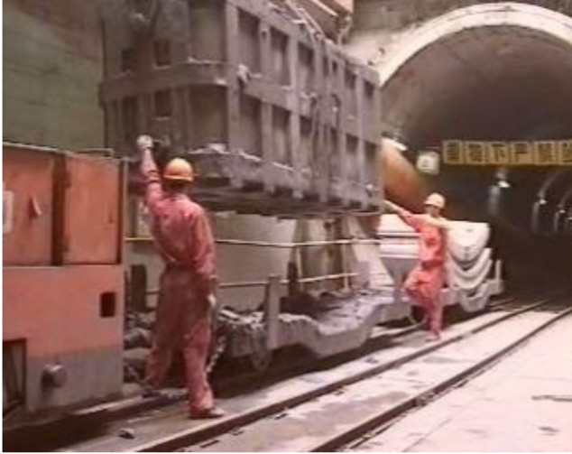
Figure 4.55 Vertical hoisting box.
