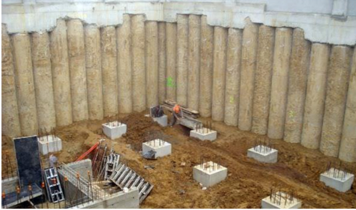
Figure 4.8 Tangent bored piles.
