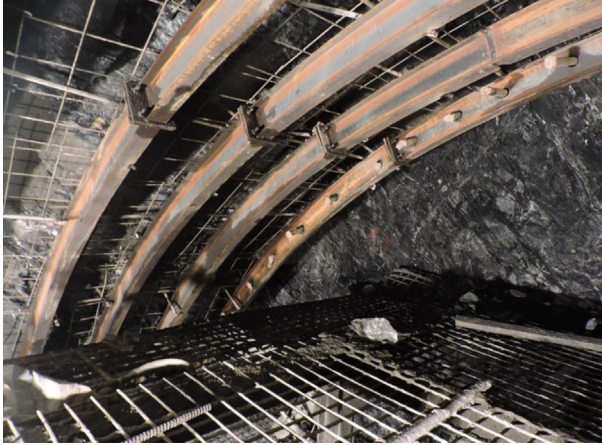
Figure 4.37 Tunnel lattice girders.
