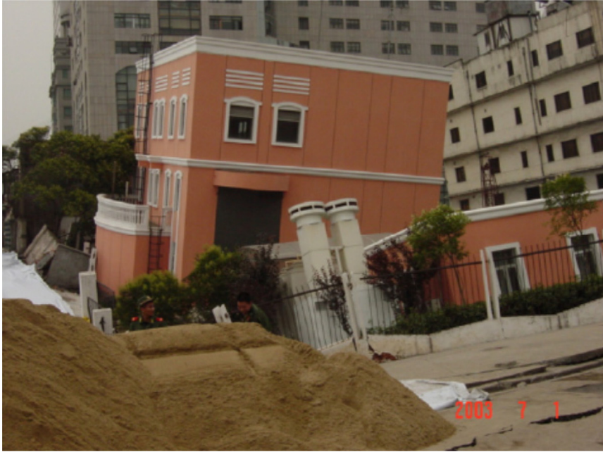
Figure 5.16 Tilting of a building above the collapsed area.
