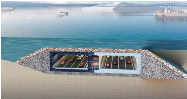
Figure 4.65 Image of an immersed tunnel.
