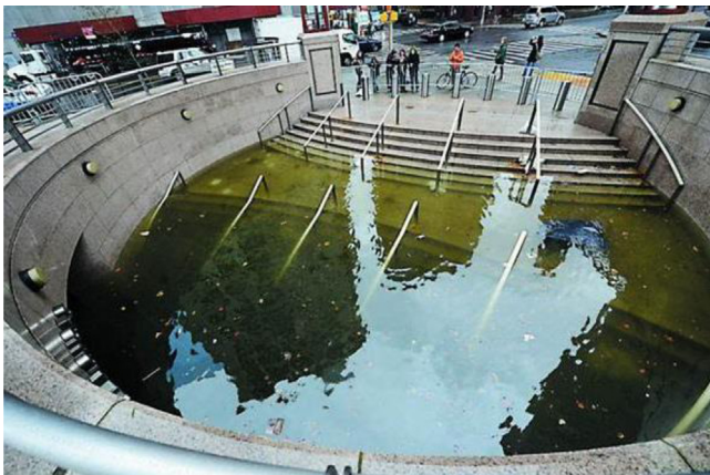
Figure 6.4 A surveillance camera image of water engulfing an underground station (AP, 2012).
