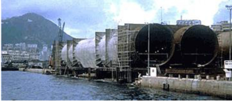
Figure 4.67 Hong Kong cross-harbor tunnel elements nearly ready for side launching (FHWA, 2009).
