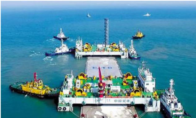
Figure 4.75 Tunnel elements in transportation.
