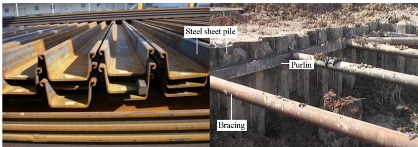
Figure 4.6 Steel sheet piles.
