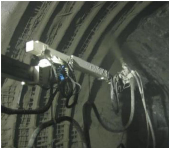
Figure 4.39 Sprayed concrete system.
