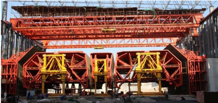
Figure 4.71 Full section of the hydraulic automated formwork system HMZB tunnel.
