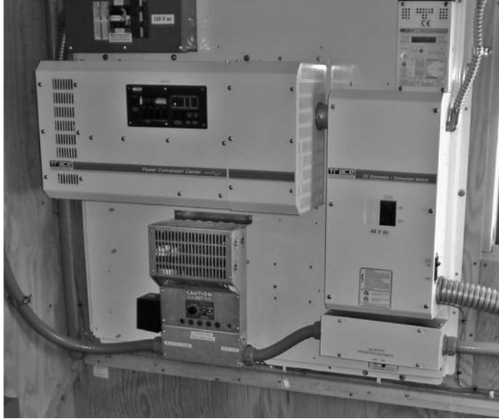
FIGURE 6.11 Example of a stand-alone inverter setup (Xantrex/Trace) as part of DC load center.
