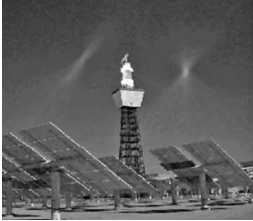
FIGURE 4.19 Primary and secondary focal points seen in the air at the Barstow power tower in California (Courtesy DOE).
