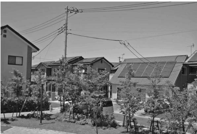
FIGURE 8.1 Ohta City has the highest concentration of grid-tie PV homes, with over 500 homes installed in this neighborhood.
