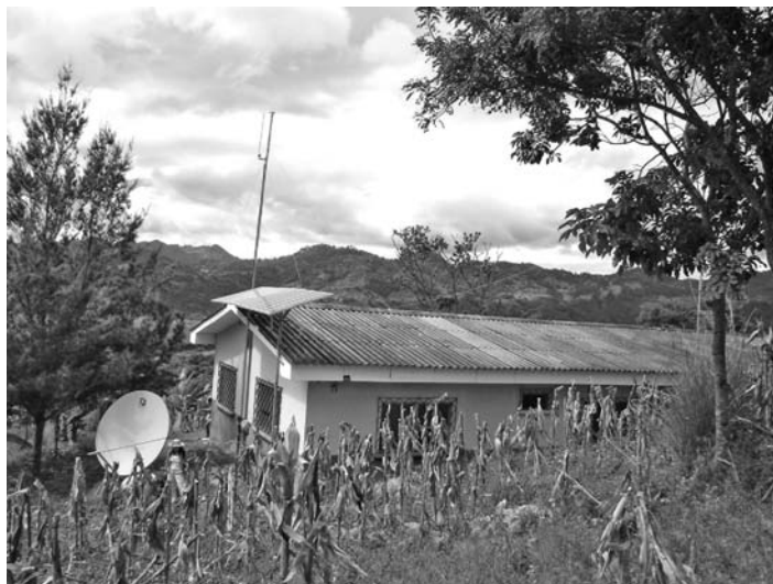
FIGURE 1.1 Remote PV-powered school for satellite-assisted education in the Lempira Province of Honduras.
