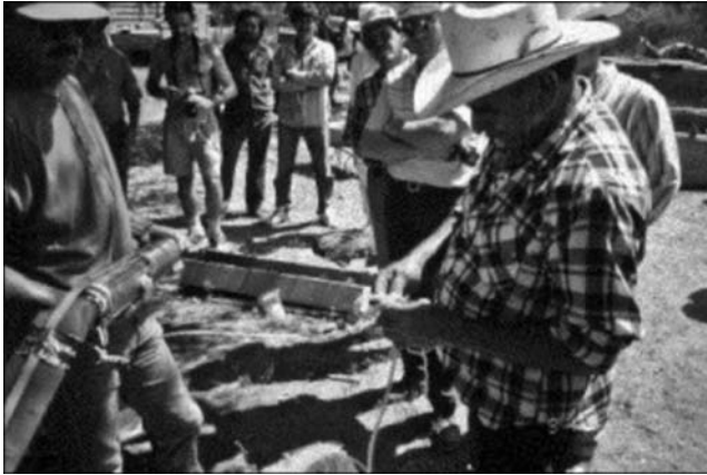
FIGURE 8.42 Installation of a PV submersible pump in Sonora, Mexico.
