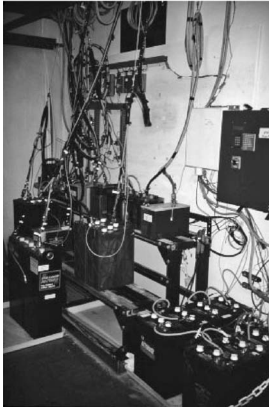
FIGURE 11.5 Battery testing at Sandia National Laboratories' PV systems lab.
