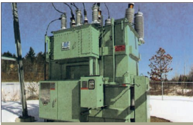
FIGURE 18-36 Three-phase autotransformer.
