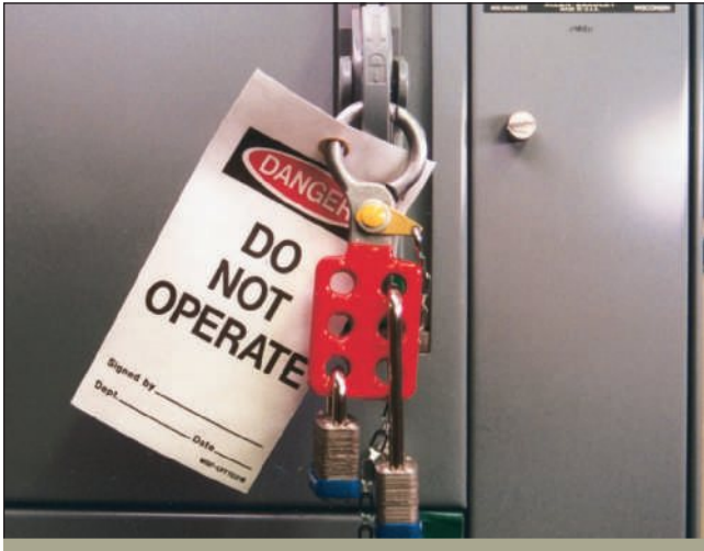
FIGURE 1-5 The equipment can be locked out by several different people.
