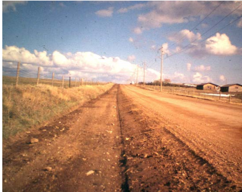
Excellent roadway reshape done with only motor graders, a roller and water truck.
