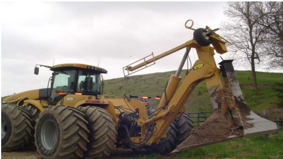
This large tile plow was brought in which is commonly used in some regions to install polyethylene pipe into farm fields for drainage purposes. This type of machine has also been used to plow drain tile into gravel roads with great success.
