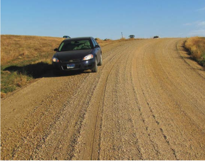
Wrong shape on curve which increases risk of crashes.
