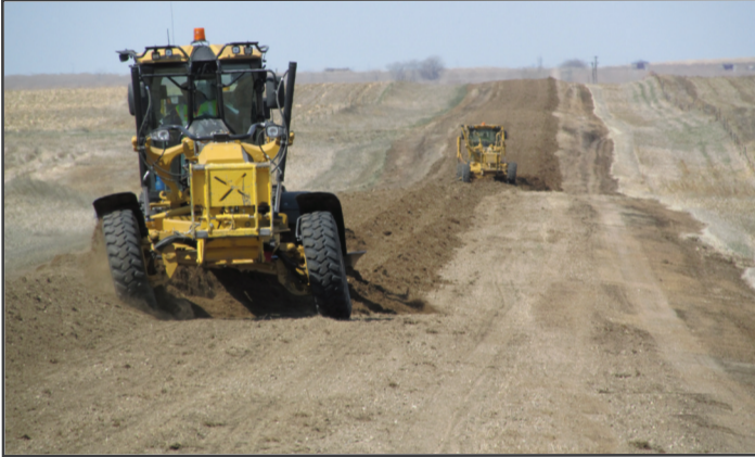
Reconstruction work space. (Source: Greg Vavra, SDLTAP).
