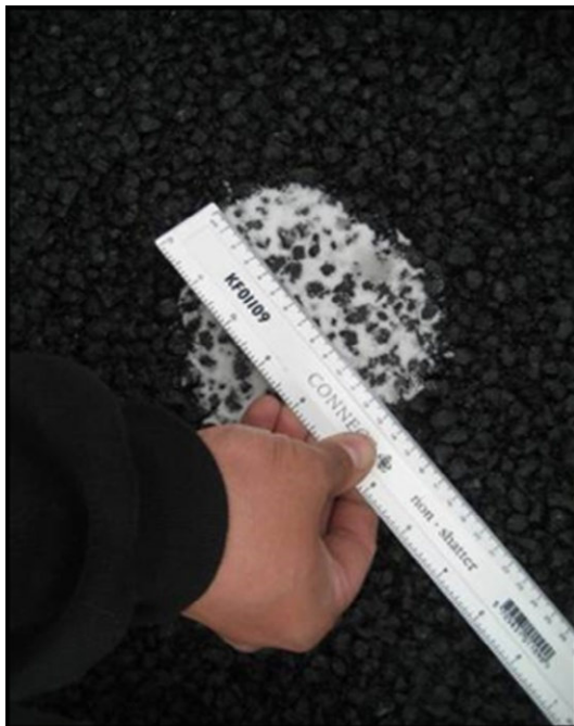
Fig. 14.4 In situ testing of macrotexture depth.
