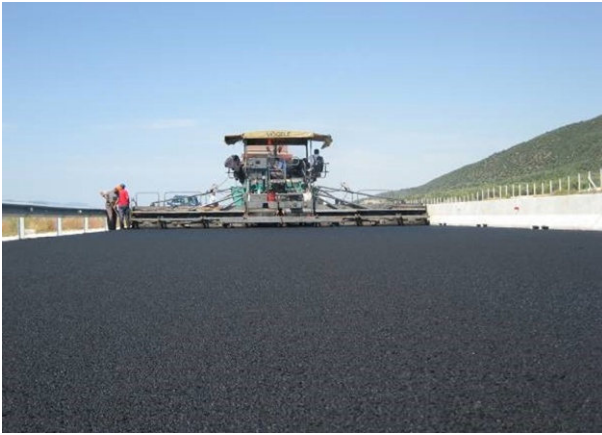
Fig.14.2 Asphalt paving.
