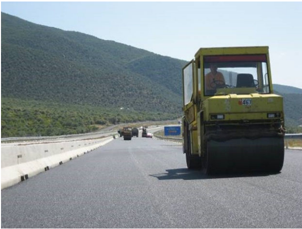
Fig. 14.3 Mix compaction.
