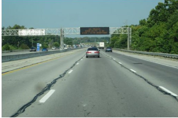
Fig. 10.7 Thin 4.75 mm dense-graded HMA overlay.
