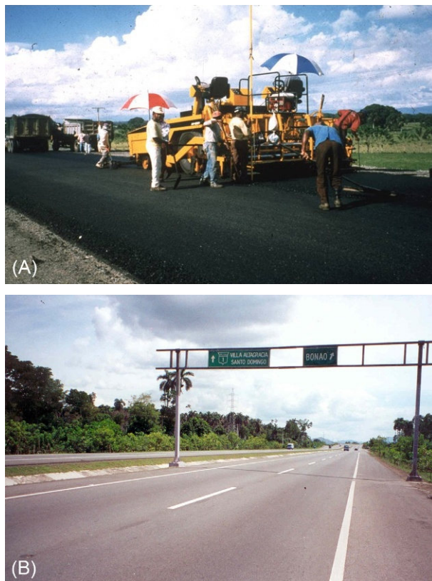
Fig. 14.14 Duarte Highway near Bonao, Dominican Republic: (A) Paving of HMA contains nickel slag aggregate (B) 5 years after construction.
