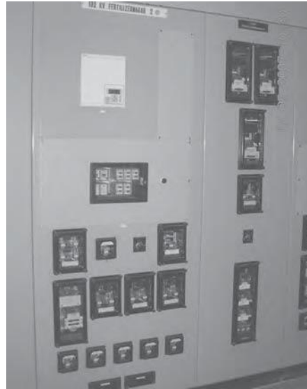
Fig. 4.1(b) Numerical distance relay scheme
