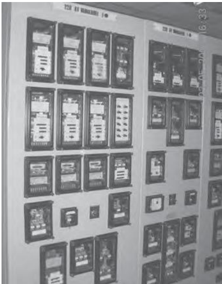
Fig. 4.1(a) Old distance relay scheme
