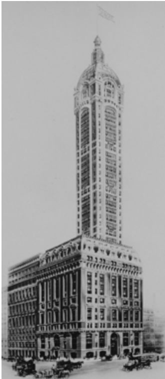
FIGURE 1.4 Singer Building, New York, USA, 1908
