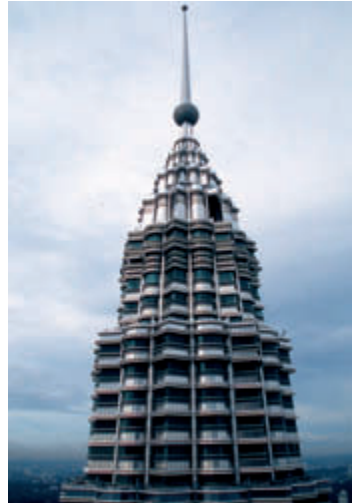
FIGURE 6.10 The Petronas Twin Towers, aerodynamic top (courtesy of Antony Wood/CTBUH)
