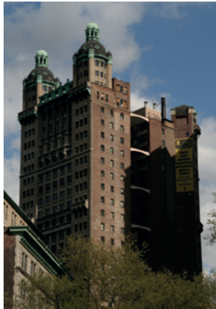
FIGURE 1.3 Park Row Building, New York, USA, 1899 (courtesy of Antony Wood/CTBUH)
