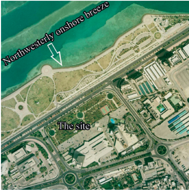
FIGURE 4.2 Site of BWTC (credit for photo: WS Atkins & Partners, Middle East)
