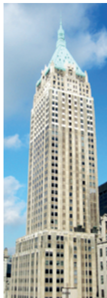
FIGURE 1.6 The Trump Building, New York, USA, 1930
