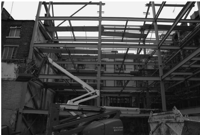
Photograph 13.2 Rear view of façade to row of terraces; shows new steel frame inserted behind façade
