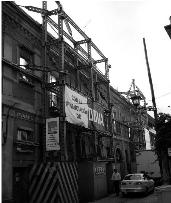
Photograph 13.7 Temporary external façade support – proprietary system
