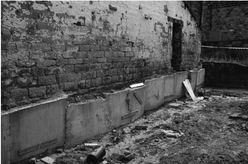
Photograph 11.3 Mass concrete underpinning
