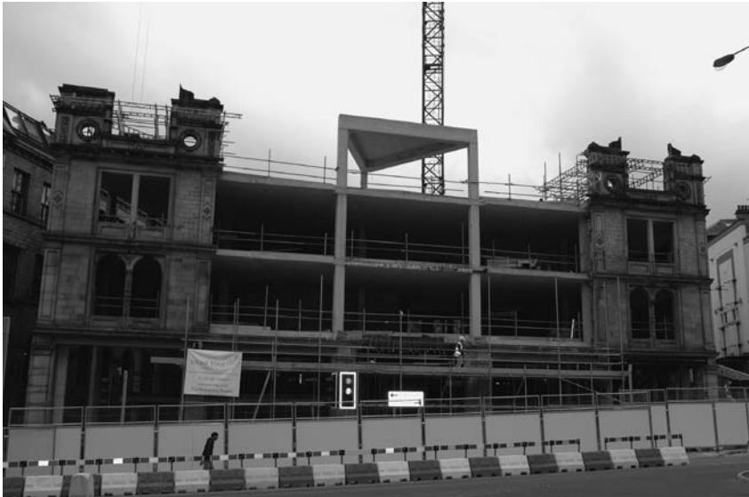
Photograph 13.34 Façade removed brick by brick
