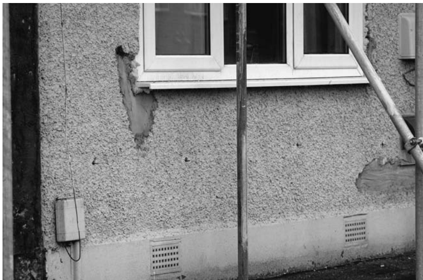
Photograph 12.1 Remedial cavity ties inserted: cracks in the render and structure have been filled and sealed with epoxy resin, ready to receive insulation and render
