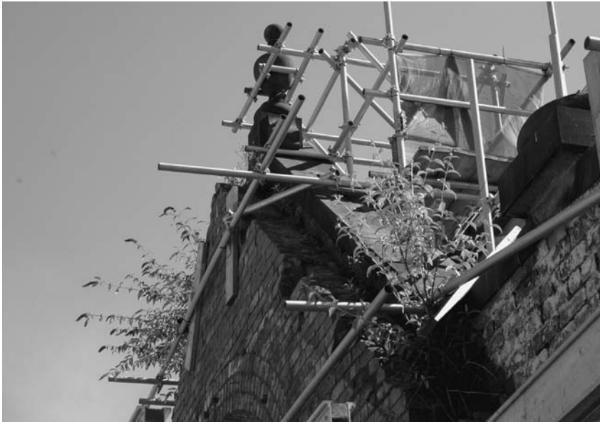
Photograph 13.31 East Brook Hall, Bradford: each ornamental feature may need to be individually supported and braced
