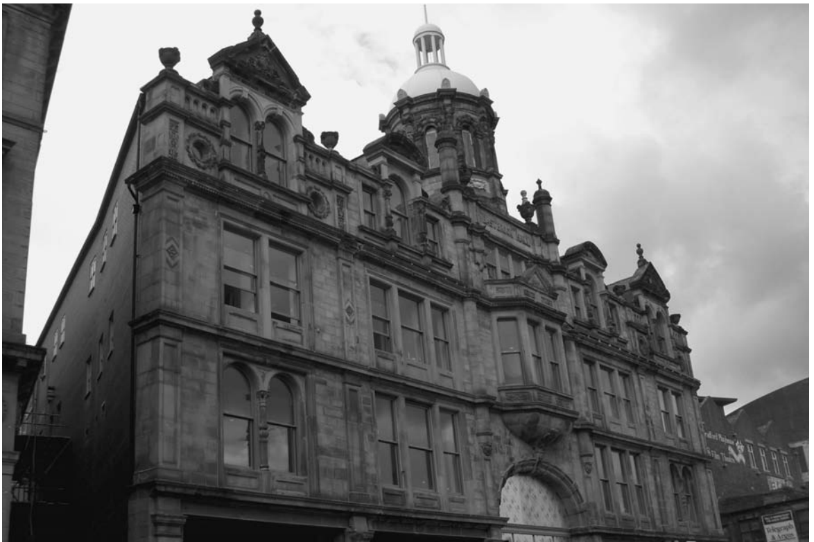
Photograph 13.35 Completed façade after rebuild
