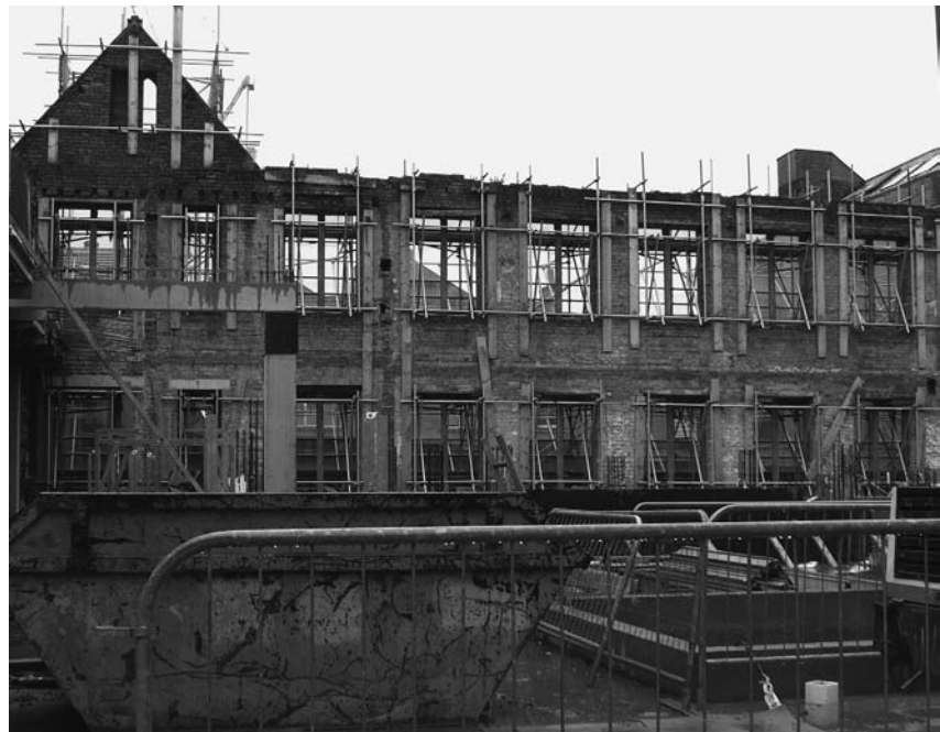
Photograph 13.6 Internal view of façade retention scheme at East Brook Hall, Bradford (cropped)
