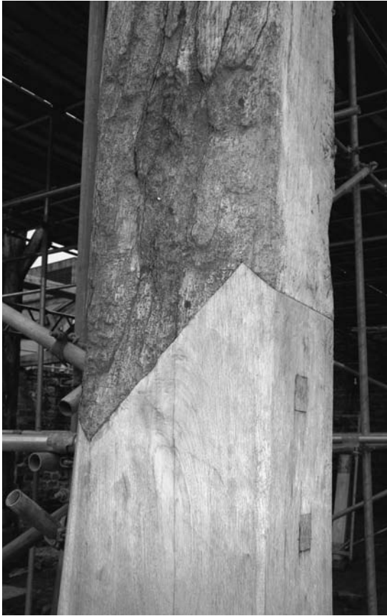
Photograph 8.15 Pinned mortise and tenon joint
