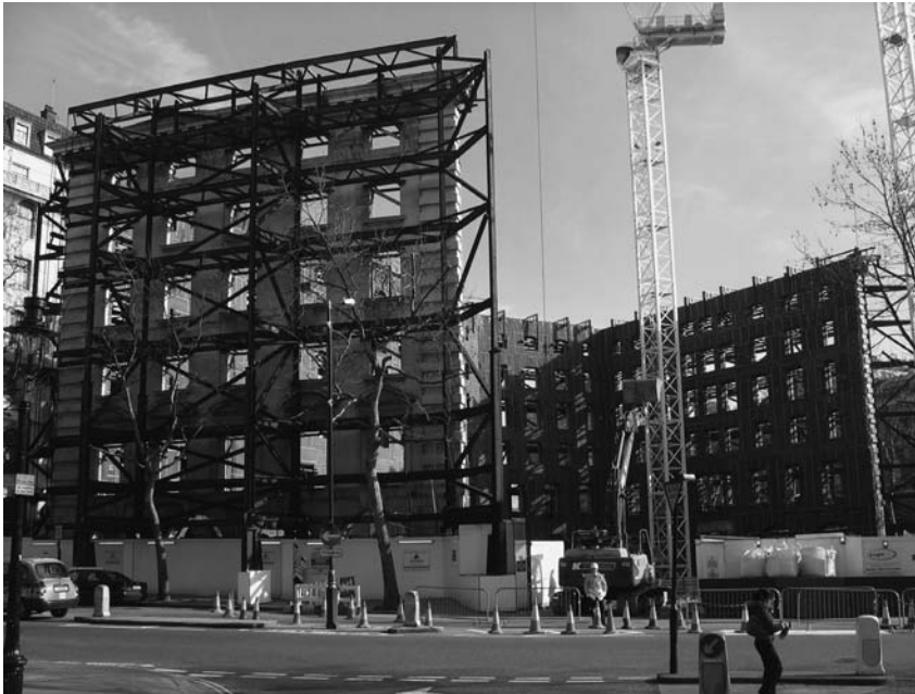
Photograph 13.38 External rolled steel façade retention system
