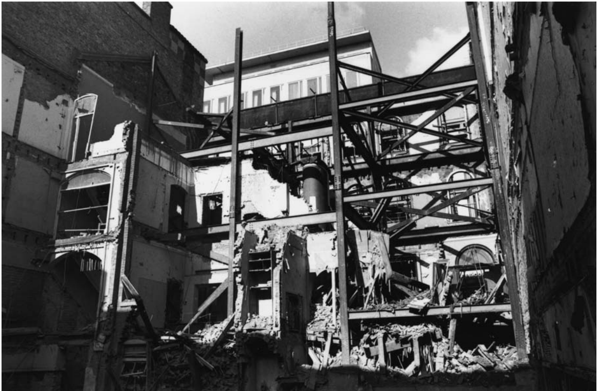
Photograph 13.13 Use of new steel frame to provide support; wholly internal façade support system
