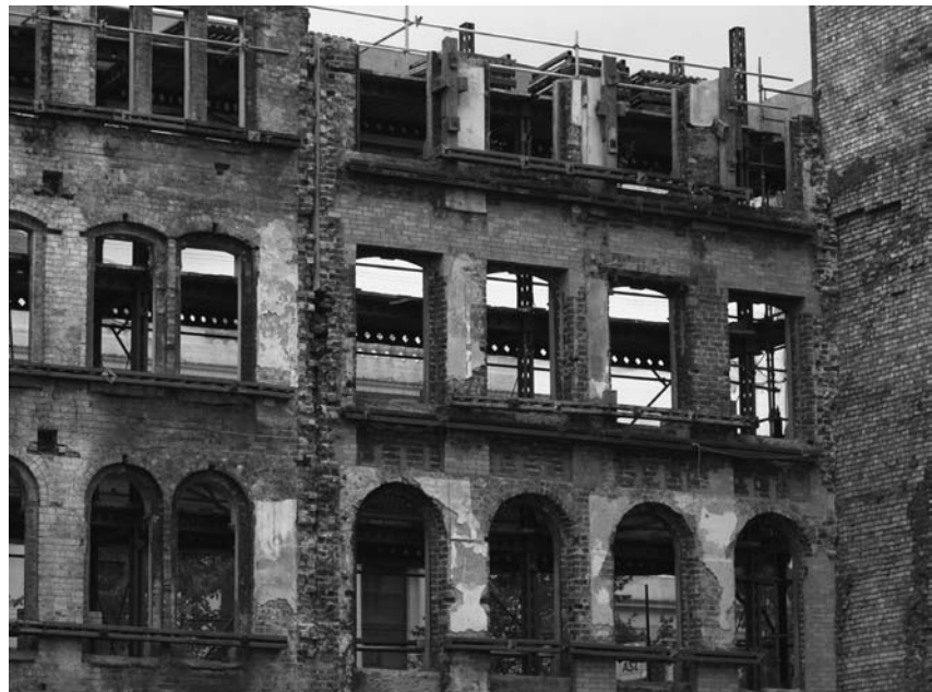
Photograph 13.23 Proprietary external façade support system, showing through-ties and straps across the internal face of the building, Belfast
