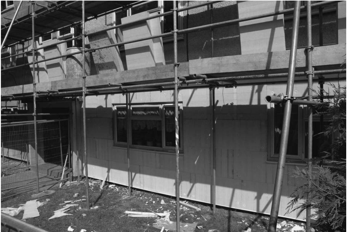
Photograph 4.9 External insulation bonded to existing wall
