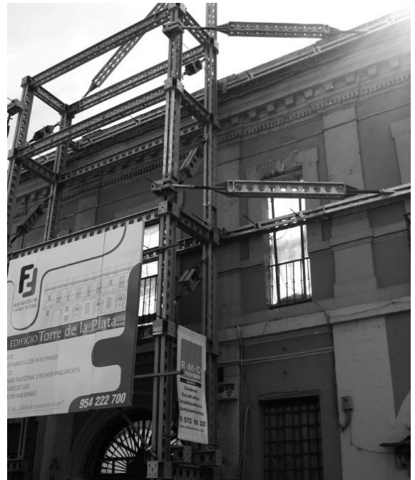
Photograph 13.8 Adjustable façade retention system
