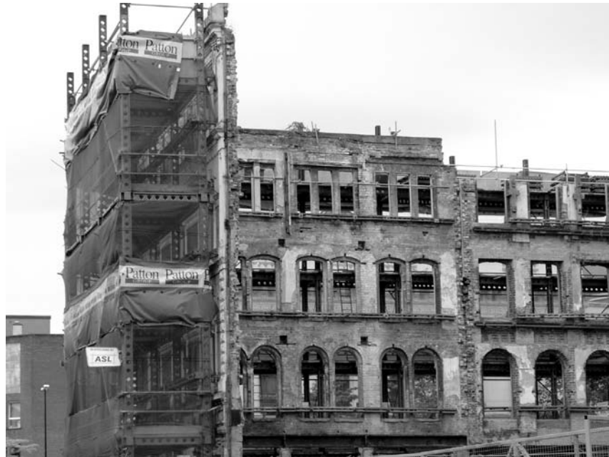
Photograph 13.22 Proprietary external façade support system, Belfast
