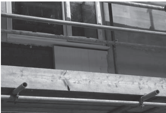
Photograph 4.10 First coat of render applied directly to the external insulation
