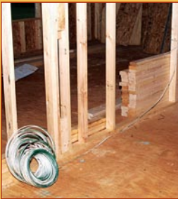
147 | Pulling Cable in New Construction
