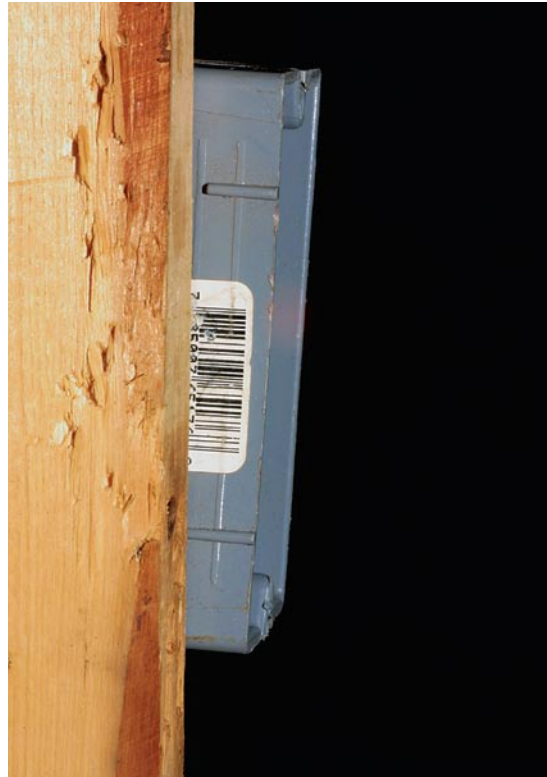
The front edge of the box must be parallel with the stud—not angled like the one shown here—extending just far enough to make it flush with the finished wall.
