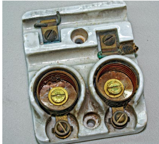
An early one-circuit main or branch circuit panel that fused both the hot wire and the neutral. It used common screw-in fuses so you could change your main breaker to what you wanted regardless of the consequences.
