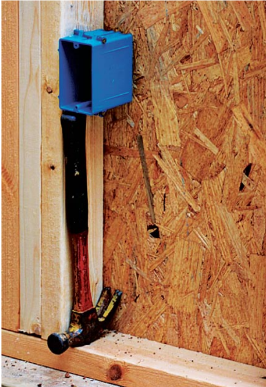
Using a hammer as a height gauge keeps all receptacle boxes at the same level and allows for quick installation.
