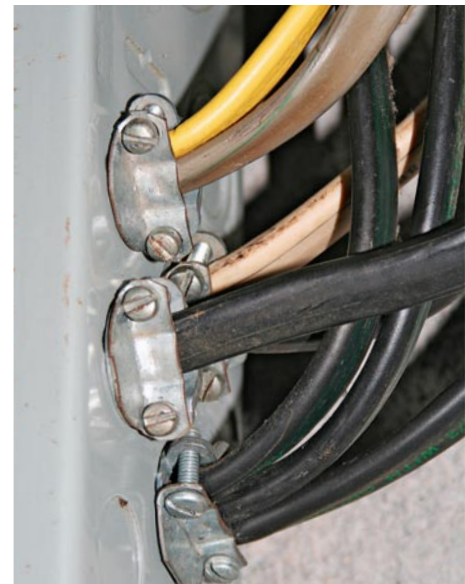
NM clamps tightening on the side of cable can damage the cable (top). A singular clamp if overtightened can damage cable (extremely common) (middle). Three cables (against code) in a NM clamp almost guarantees a damaged cable (bottom).
