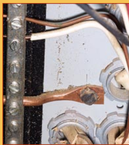
96 | Bringing Cables into the Panel
