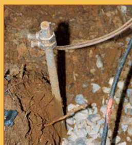
118 | A Low- Resistance Panel-to-Earth Ground
