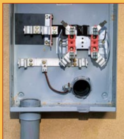
78 | Connecting Meter Base to Panel
