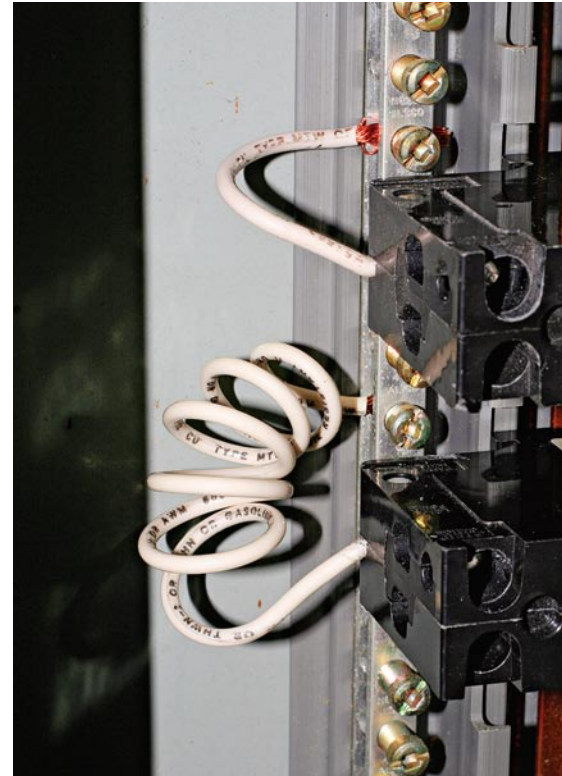
An AFCI works the same whether a white pigtail is left long and coiled (as it comes out of the box) or cut short.
