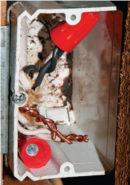
A wire connector has fallen off the neutral splice and the ground wire is pressing against bare neutral.
