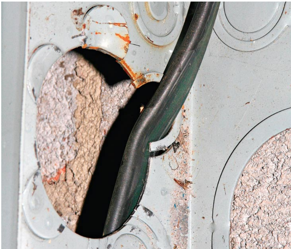
A panel entry without an NM clamp can cut or puncture a cable.
