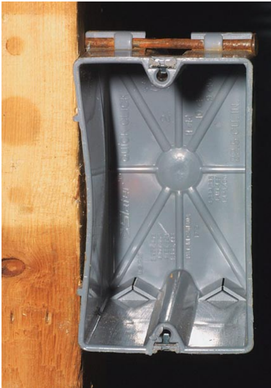
One too many hammer hits will warp a thin plastic box.
