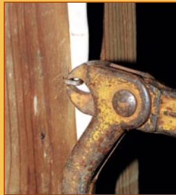
157 | Routing Wires in Renovation Work
