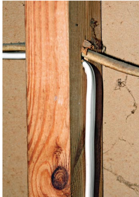
Pinch point. Never pull an immediate turn with a cable. It can heat up and arc.
