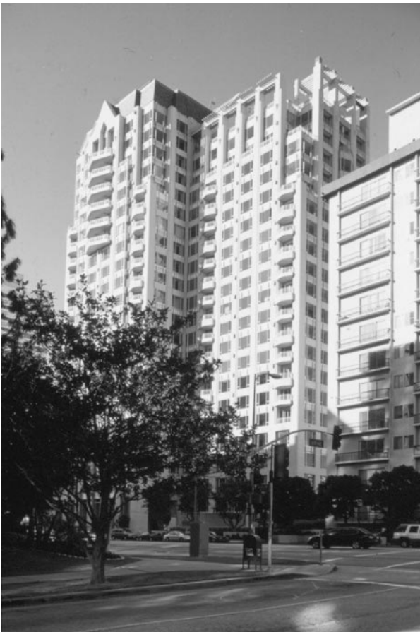
Photo 4.2 Precast concrete clad poured-in-place concrete ductile frame braced condominium, The Remington, Los Angeles, CA, 2002. (Courtesy of Magee Architects, Inc.)
