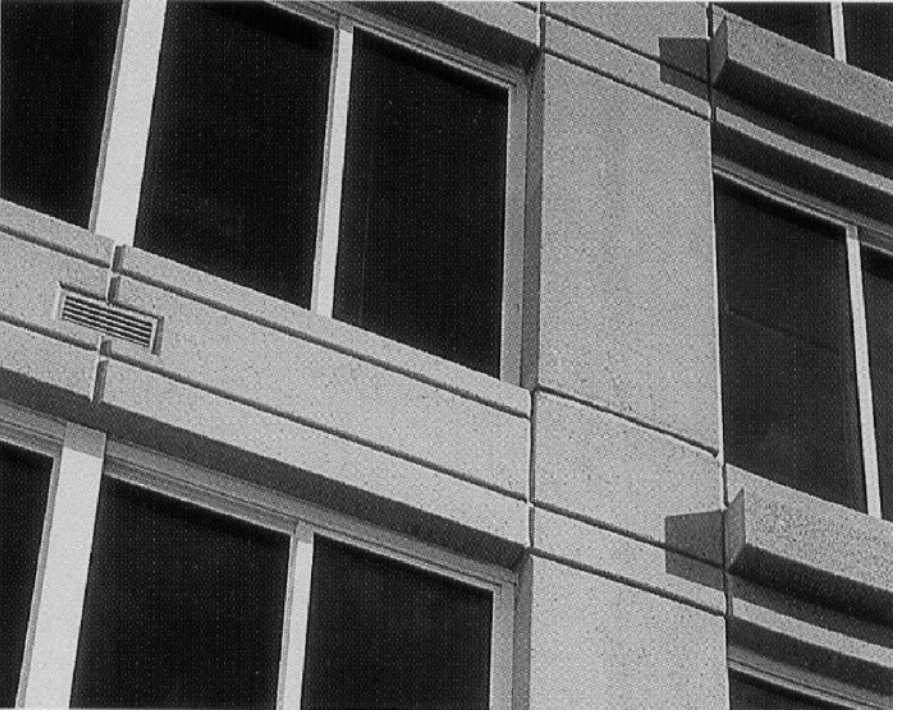
Figure 3.1.16 Concrete finishes. Precast concrete tames. (Courtesy of Pankow Builders.)
