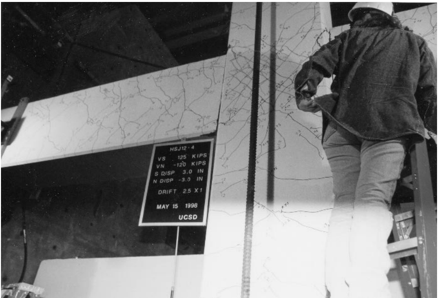
Photo 2.8 Beam-column joint at 2.5% drift, University of California San Diego.
