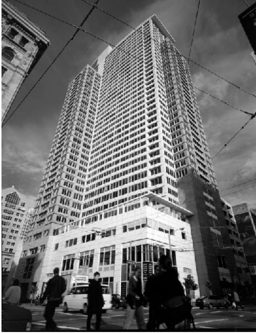
Photo 2.4 Paramount Apartments, San Francisco, CA. (Courtesy of Charles Pankow Builders.)
