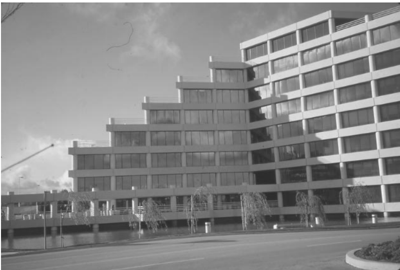
Photo 4.1 Precast clad concrete frame, Mariners Island, San Mateo, CA. (Courtesy of Englekirk Partners, Inc.)
