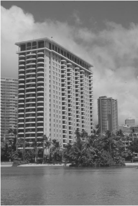
Photo 1.2 Exposed cast-in-place concrete, Lagoon Towers, Honolulu, HI, 1965. (Photo by Robert E. Englekirk.)
