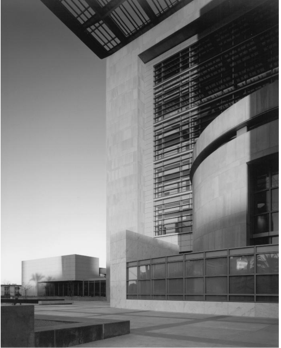
Figure 3.1.16 (Continued) Concrete finishes. Limestone on precast concrete panels. (Courtesy of Clark-Pacific.)
