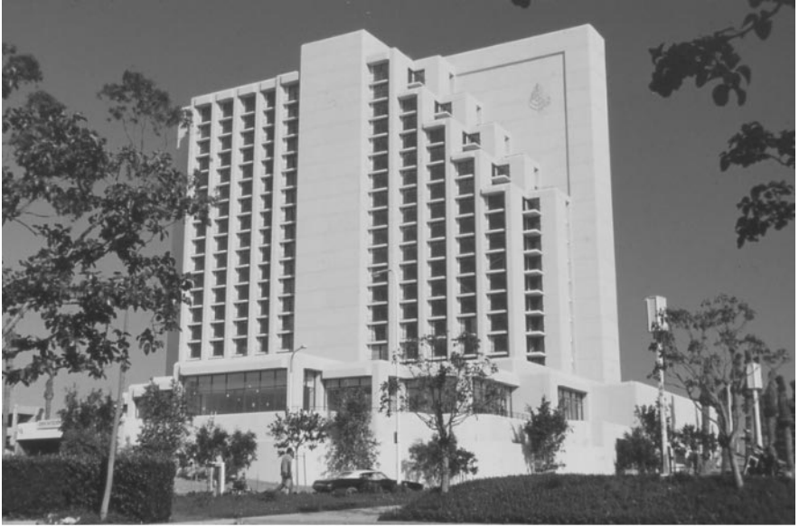
Photo 1.3 Precast clad concrete frame, Four Seasons, Newport Beach, CA. (Courtesy of Englekirk Partners, Inc.)
