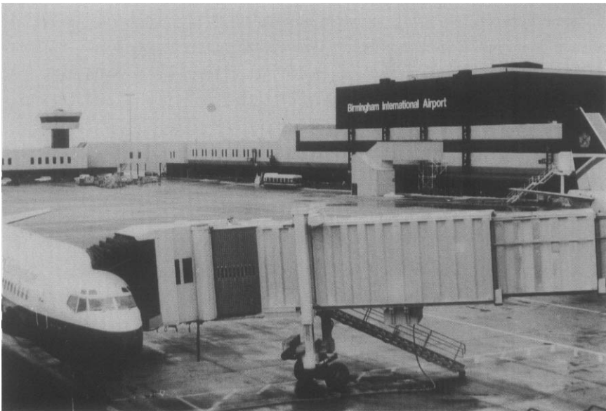
Figure 8-5 A passenger boarding bridge with a wide range of adjustment (photo A. Kazda)
