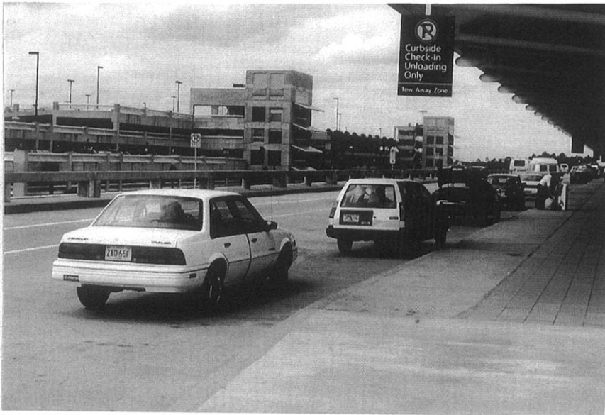
Figure 16-1 Kerb in front of the departure concourse for passenger drop-off (photo A. Kazda)
