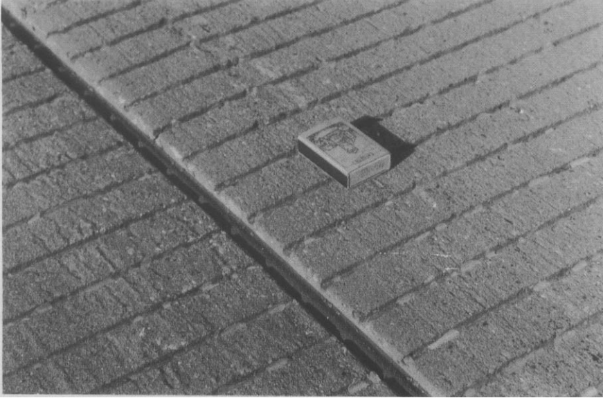
Figure 5-18 Pavement transversal grooving (photo A. Kazda)
