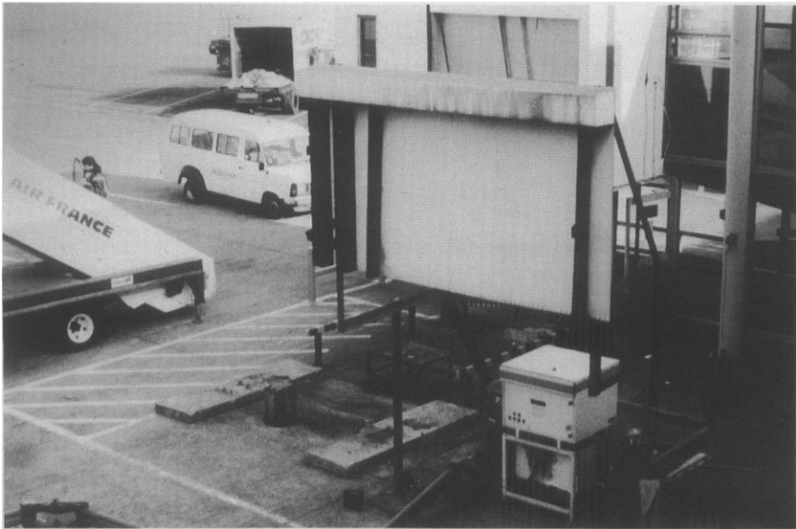
Figure 8-13 Side marker board (photo A. Kazda)
