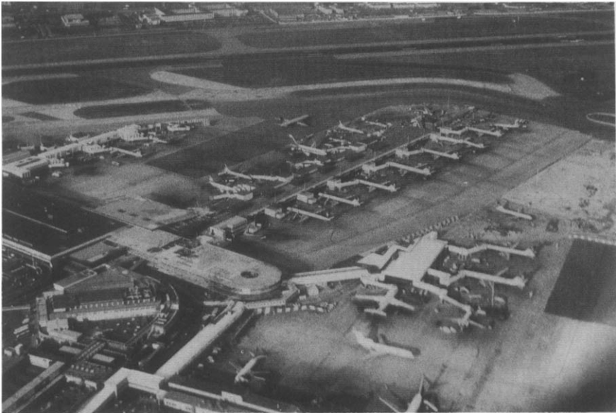
Figure 7-5 Pier system at London Heathrow Airport (photo A. Kazda)
