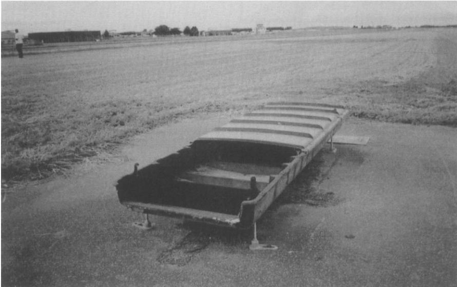
Figure 10-18 T-VASIS light unit, Hamilton Airport, New Zealand (photo A. Kazda)
