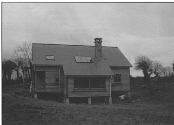
Plate 10. House in Sligo, Republic of Ireland
