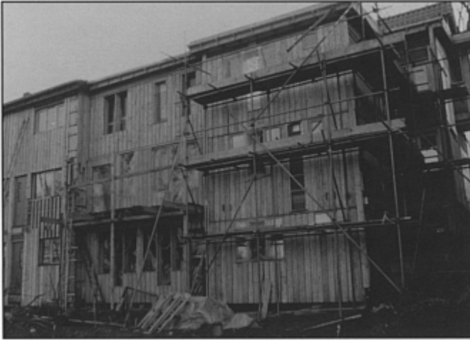
Plate 7. Housing at Chapel Allerton (Rear elevation)
