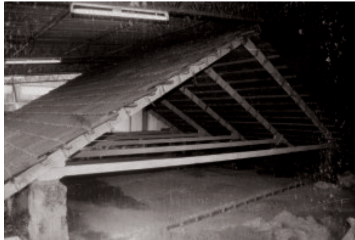
Fig. 6.5. Prefabricated roof truss and rafters for Mangalore tiled roof
