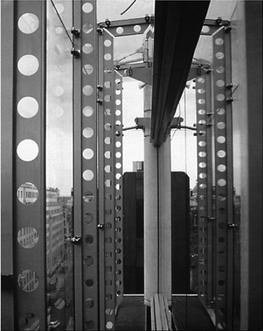
4.1 Detail of triple-glazed facades. Helicon Building, London. Architects: Sheppard Robson,
