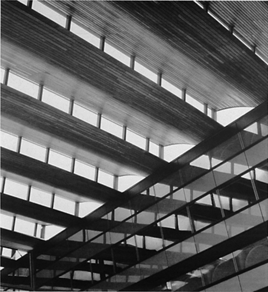
7.10 Use of sustainable hardwood, Mistral Building, Reading. Architects: Foster and Partners.
