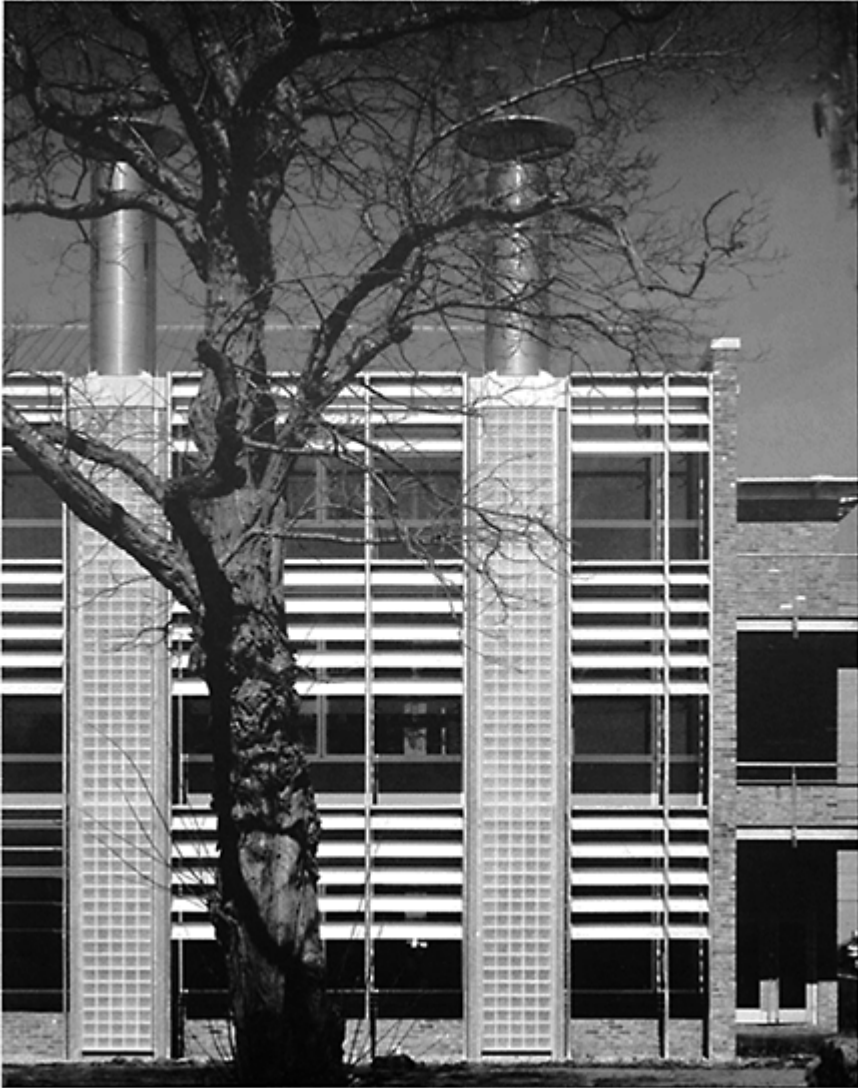
11.1 Detail of south facade showing relationship between ventilation stacks and solar shading. The Environmental Building, BRE, Garston. Architects: Feilden Clegg.
