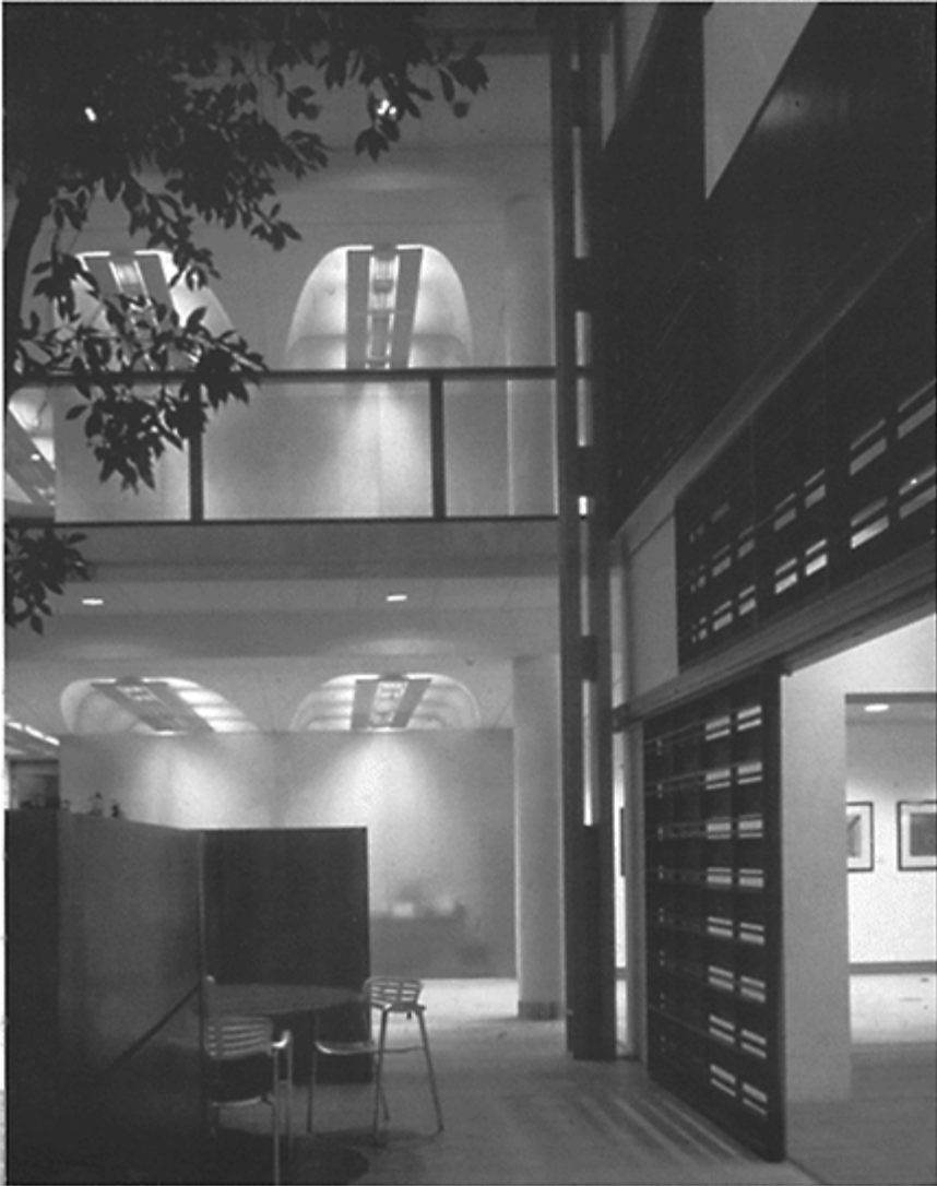
8.5 View of atrium (left) and office area (right): note the timber solar screen. Architects: Bennetts Associates.
