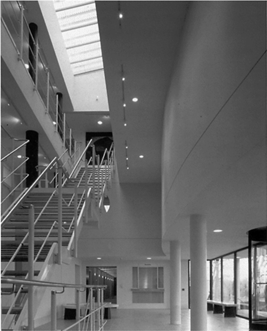
13.6 Entrance hall at Elizabeth Fry Building, University of East Anglia. Note heavyweight construction and recessed windows. Architects: John Miller and Partners.
