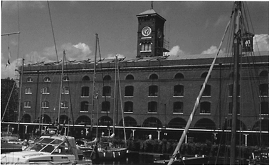
1 Ivory House in London's Docklands has changed uses several times over the past 200 years.
