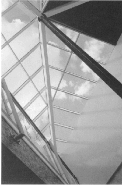
1.10 Central atrium and solar chimney, Groundwork Trust Office, Jarrow, near Newcastle. Architect Carol Townsend of EarthSense.
