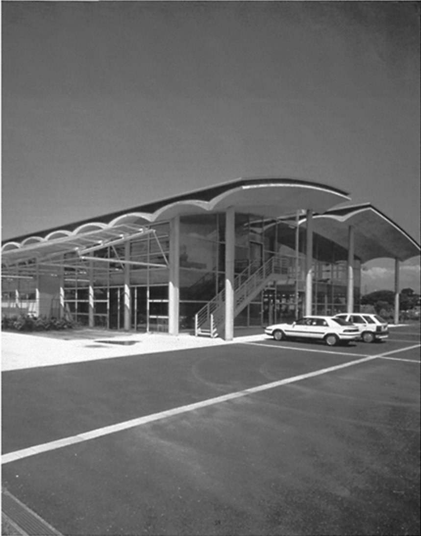
7.1 Lycée Albert Camus, Fréjus, France. Architects: Foster and Partners.
