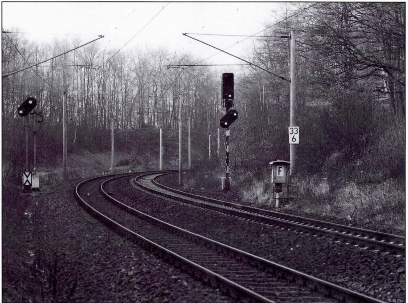
Fig. 6.7 Intermediate block signal, combined with a distant signal on the right (DB AG)
