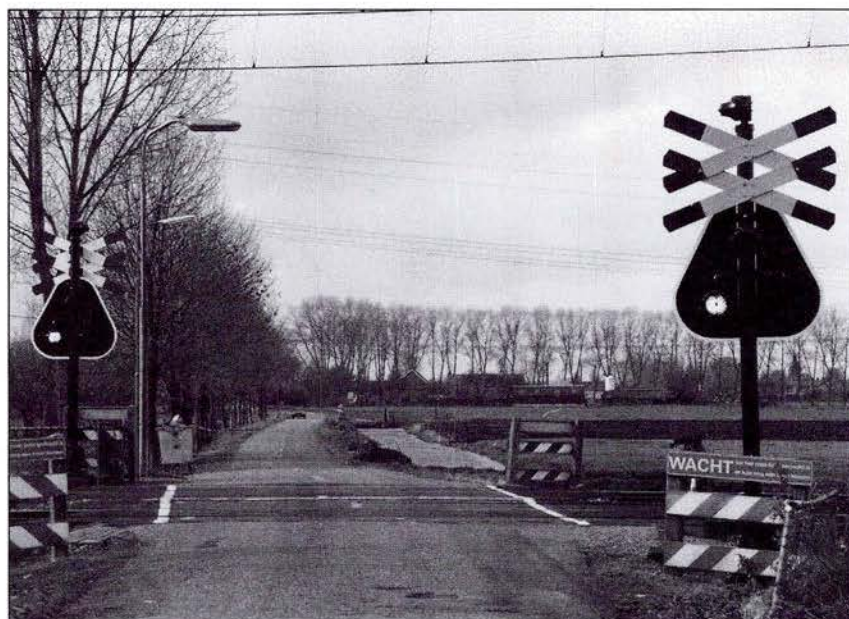
Fig. 12.1 Automatic level crossing on NS
