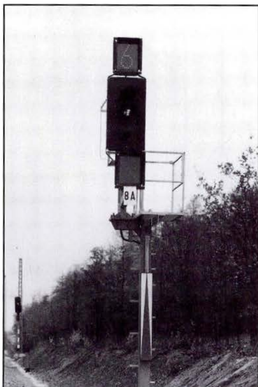
Fig. 4.16 The new German running signal 'KS' type in situ
