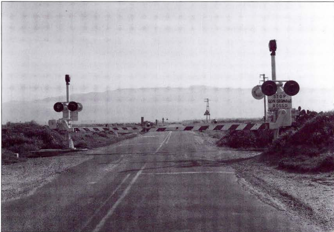
Fig. 12.4 Automatic half barrier crossing on FS
