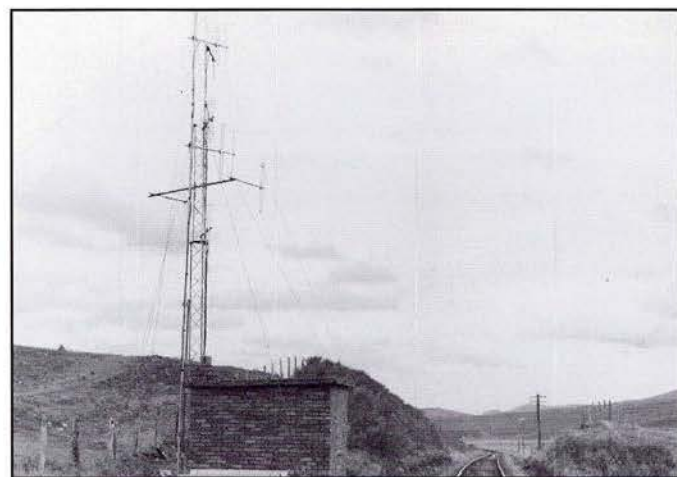
Fig. 6.2 Radio electronic token block (RETB), in use in Scotland
