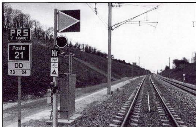
Fig. 10.4 Marker on TGV line
