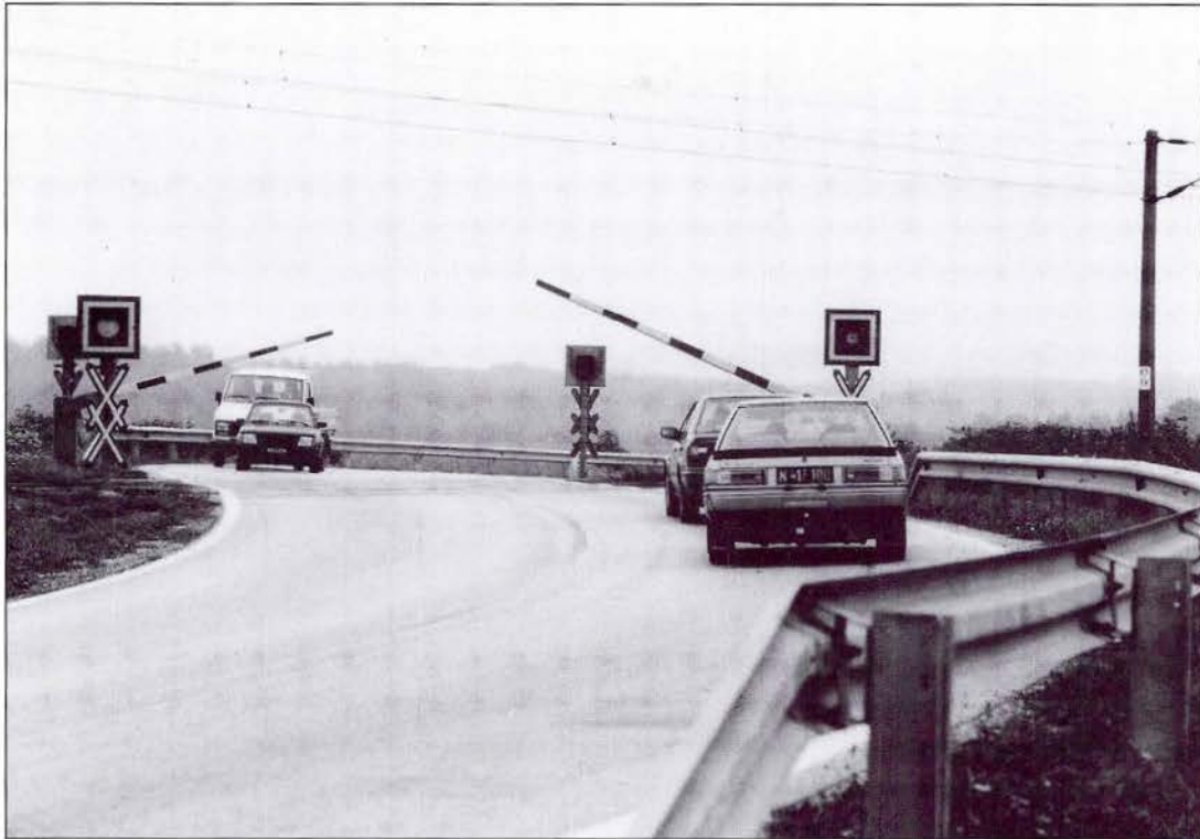
Fig. 12.3 Automatic half barrier level crossing on ÖBB
