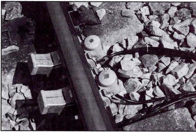
Fig. 2.10 Axle counter AZL70 type
