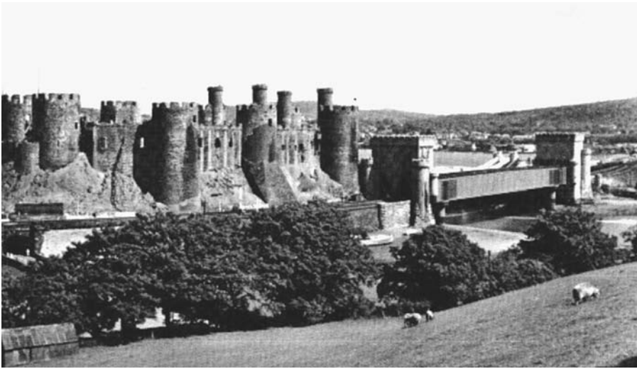
Fig. 13.11 The box-girder bridge at Conway, 25 kilometers east of the Menai Straits.
