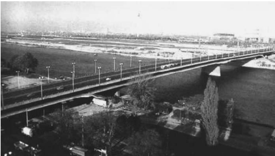
Fig. 18.15 A concrete twin-box-girder bridge was opened in November 1980. This bridge is also called the Reichsbrücke. ( www.reichsbruecke.net/geschichte_e.php )
