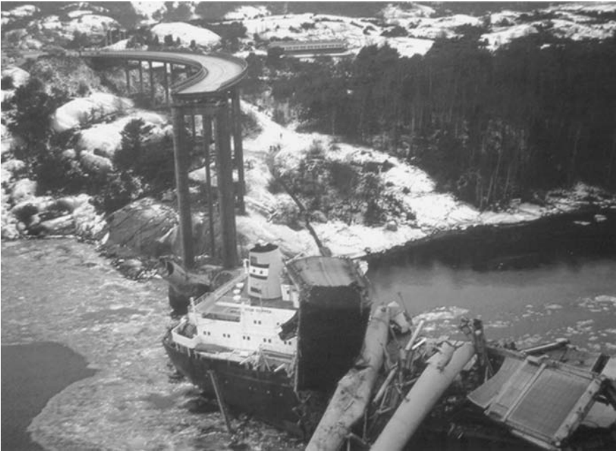
Fig. 19.8 The collapse of the Almö Bridge. (Tjörnbron. The Swedish National Road Administration. With kind permission of Lennart Lindblad)
