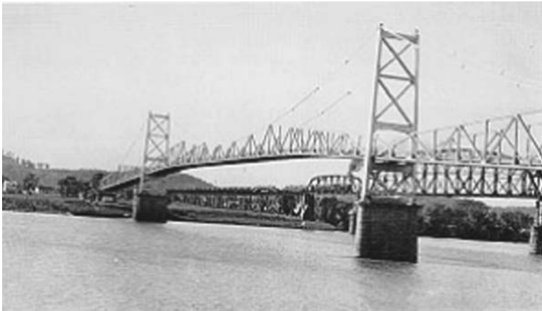
Fig. 11.3 The Point Pleasant Bridge (in the foreground). ( http://wikipedia.org/wiki/Silver Bridge )
