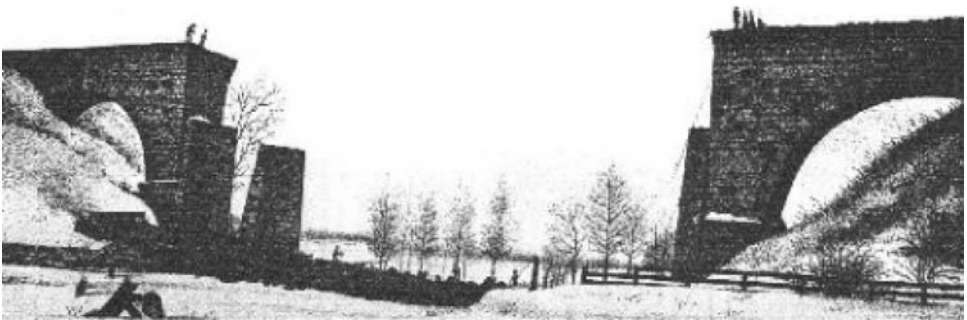
Fig. 2.4 The day after the collapse. The extra brick pier that is seen close to the left-hand abutment is from the earlier wooden bridge at this site. ( http://home.alltel.net/arhf/bridge.htm )
