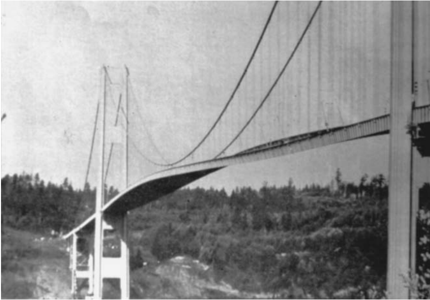
Fig. 7.4 The twisting motion of the main span. (University of Washington Libraries, Special Collections, UW 21413)
