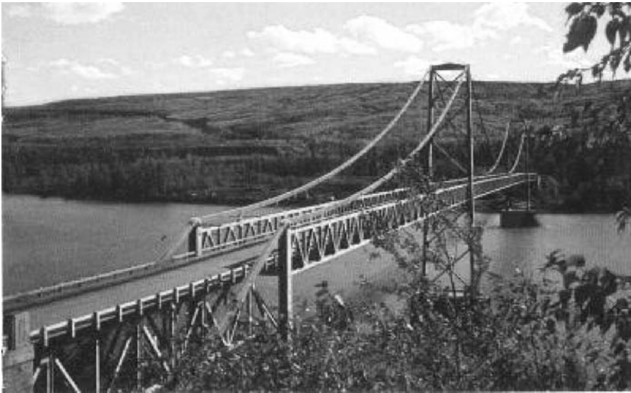
Fig. 8.4 A scenic view of the Peace River Bridge (photo taken 1950). Note the upstream sloping side of the tower piers, not only built because of increased stability in the rapid-flowing waters, but – most probably – primarily for the reduction of ice loads during winter. A nearby temporary timber bridge had in fact been damaged by ice pressure in 1942. ( www.explorenorth.com/library/akhwy/peacerverbridge.html )
