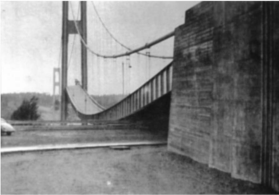
Fig. 7.7 The deflected side span on the east side, at the time of the collapse of the main span. (University of Washington Libraries, Special Collections, UW 27459z)
