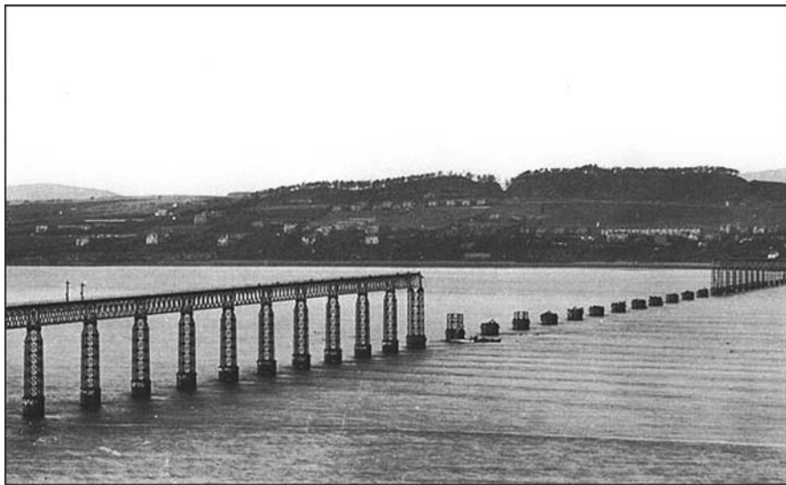
Fig. 3.7 All thirteen high girders of the Tay Bridge had collapsed into the river. (Wolcott: The breaks of progress. Mechanical Engineering)
