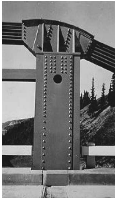
Fig. 8.7 The splay saddle on top of the cable bent. ( www.inventionfactory.com/history/RHAbriD/term/ )
