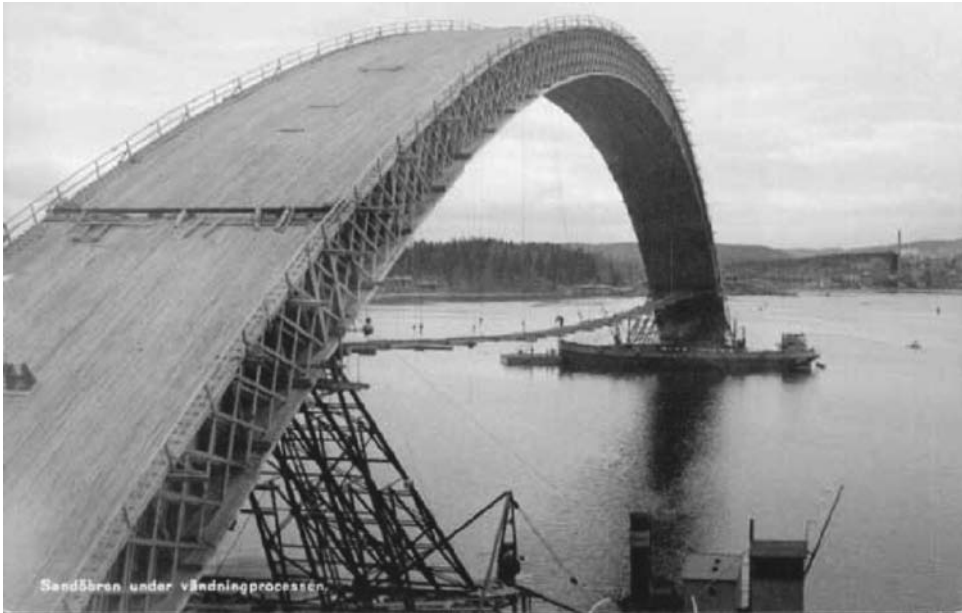
Fig. 6.2 The timber arch falsework being shipped into position. ( www.famgus.se/Gudmund/Gudm-Sandobron.htm , with kind permission of Leif Gustafsson)
