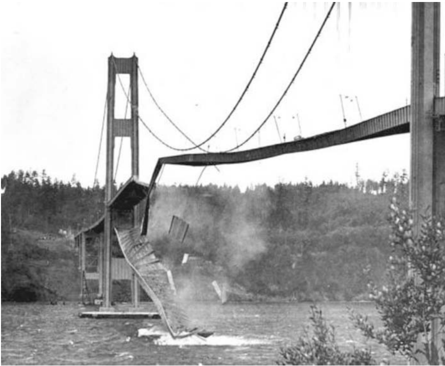
Fig. 7.6 The first part of the collapse, where 183 metres of the main span tore away from the vertical hangers (suspenders) and fell into the waters below. (University of Washington Libraries, Special Collections, UW 21422)
