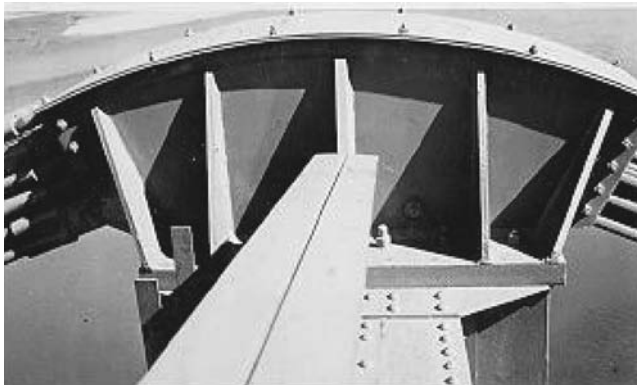
Fig. 8.6 The top of the towers, where the main cable passes over the saddle, transferring the load down vertically into the tower leg. ( www.inventionfactory.com/history/RHAbbridg/term/ )
