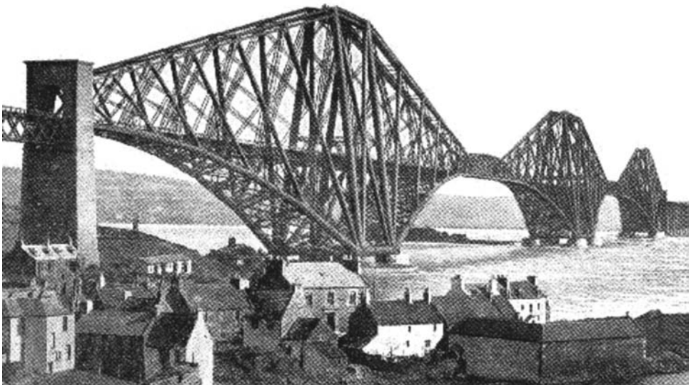
Fig. 3.23 The huge cantilever truss bridge over the Firth of Forth in Scotland, which replaced the suspension bridge proposed by Bouch. This bridge surpassed the Brooklyn Suspension Bridge from 1883 (486 m) as the longest span in the world (521 m).
