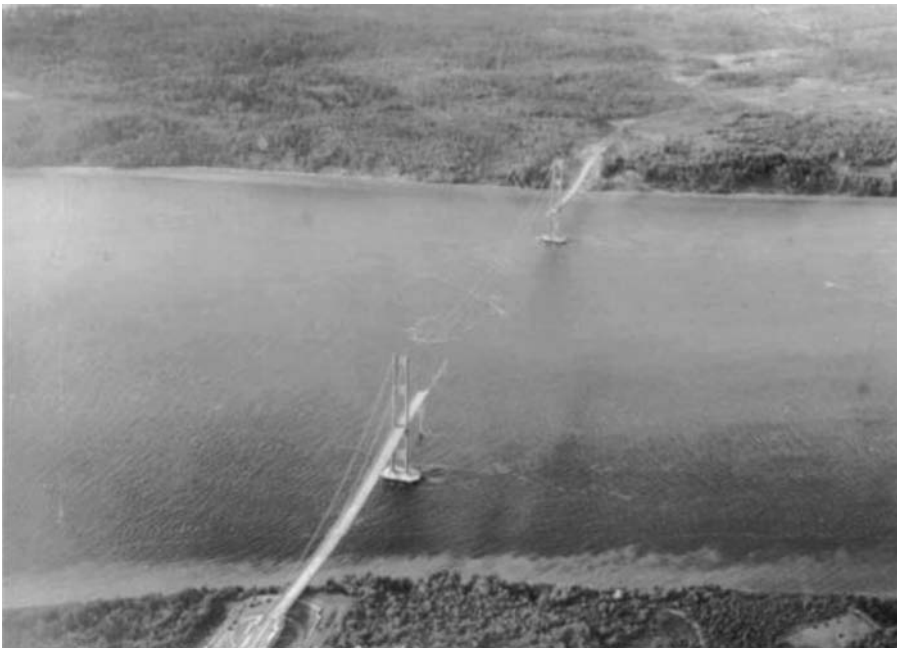
Fig. 7.8 The collapsed Tacoma Narrows Bridge – aerial view looking west, a rather sad and dreary sight. (University of Washington Libraries, Special Collections, UW 26818z)
