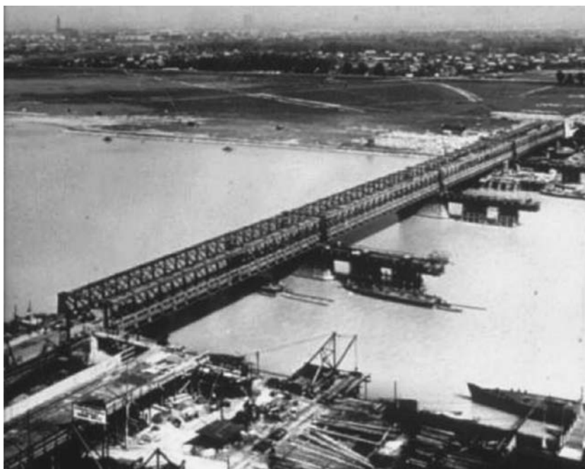
Fig. 18.1 The old truss bridge over the River Danube in Vienna – Kronprinz-Rudolph-Brücke – which was constructed in 1876. ( www.reichsbruecke.net/geschichte_e.php )
