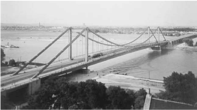
Fig. 18.2 The new bridge was opened in 1937, and replaced the old truss bridge. ( www.reichsbruecke.net/geschichte_e.php )
