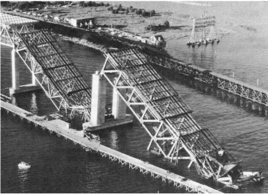
Fig. 9.4 The collapse of the Second Narrows Bridge. (McGuire: Steel Structures. With kind permission of Pearson Education Publications).
