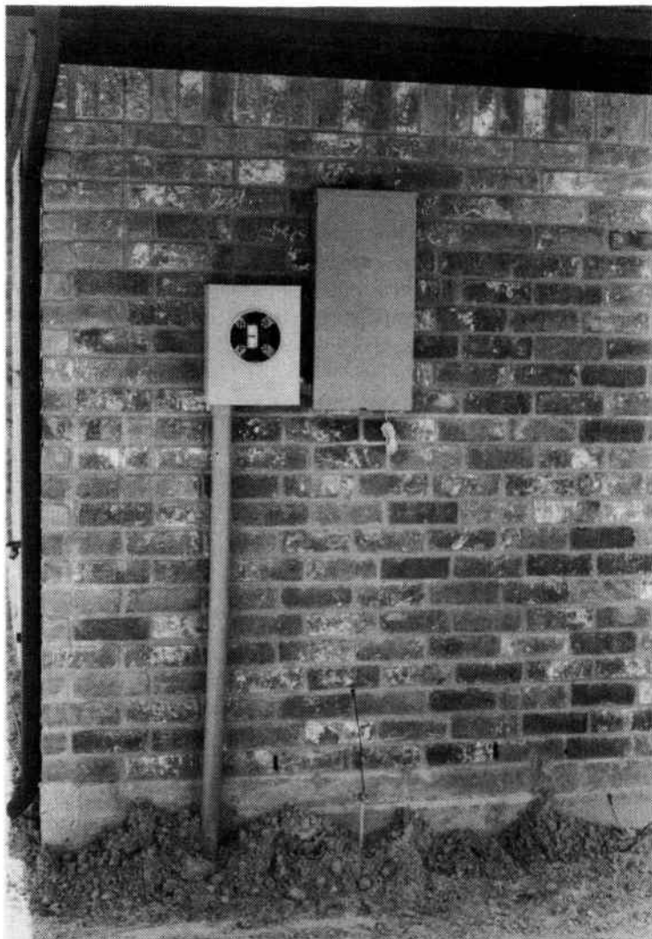
Fig. 6-71. The meter socket is now installed.
