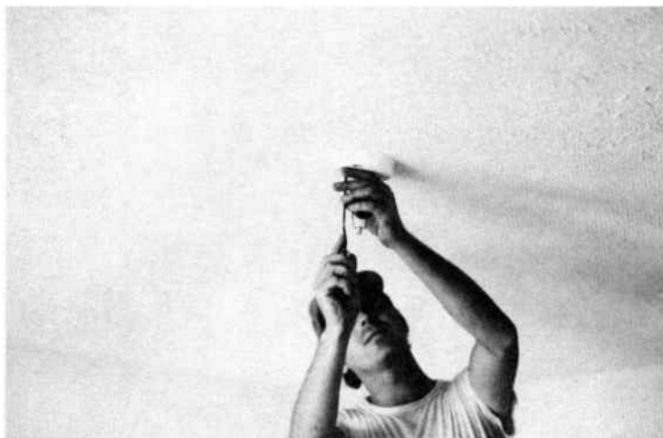
Fig. 6-58. Installation of the light fixture completes the job.
