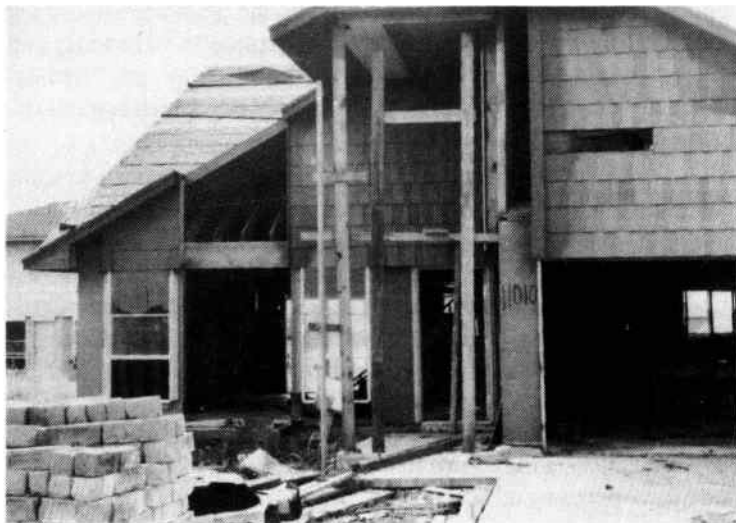
Fig. 3-11. A new home is under construction.
