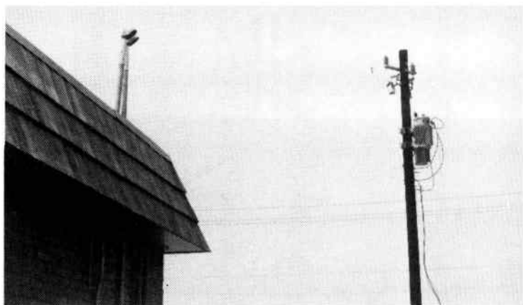
Fig. 3-7. A temporary electrical service for construction personnel comes down from the pole transformer.
