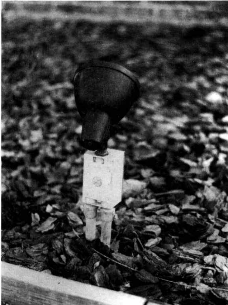
Fig. 7-13. A light with a metal hood for protection.
