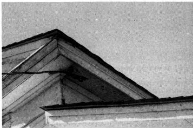
Fig. 8-2. An old service connection to an older home.
