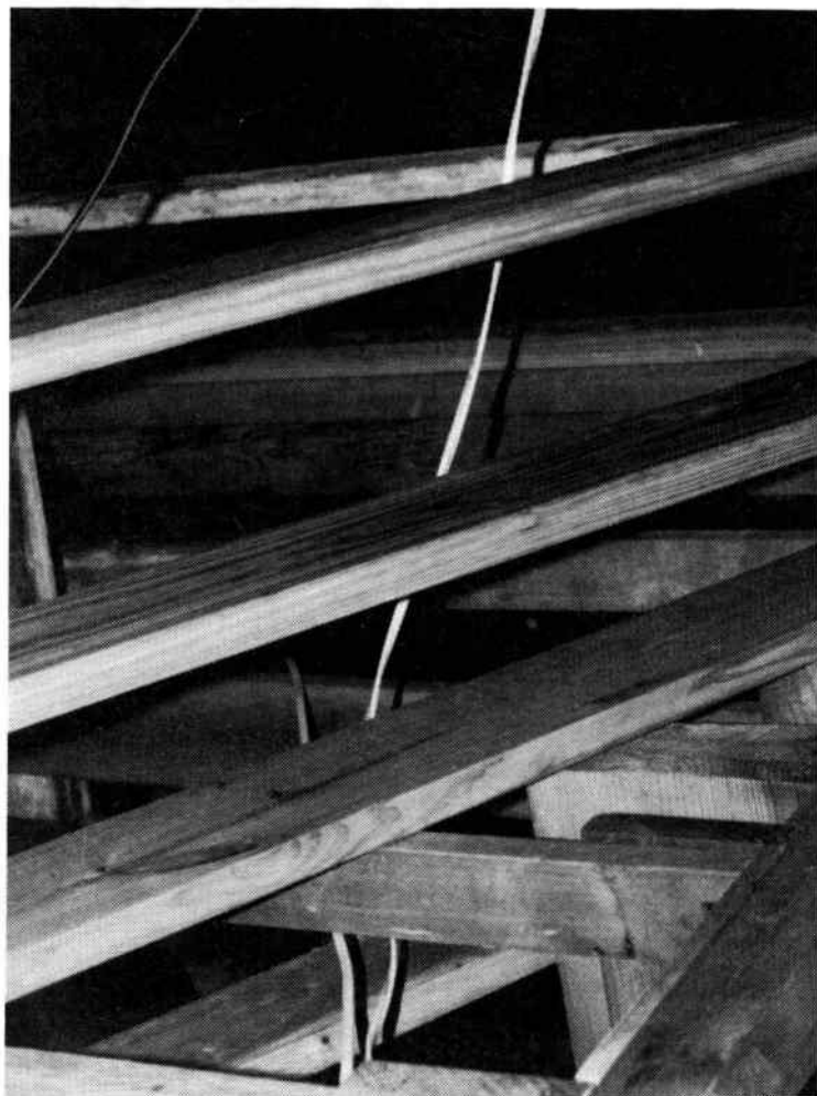
Fig. 6-20. A multi-wire cable is looped and tied to take up slack.
