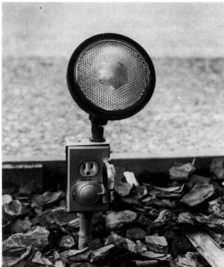
Fig. 7-12. An outside light with a receptacle.
