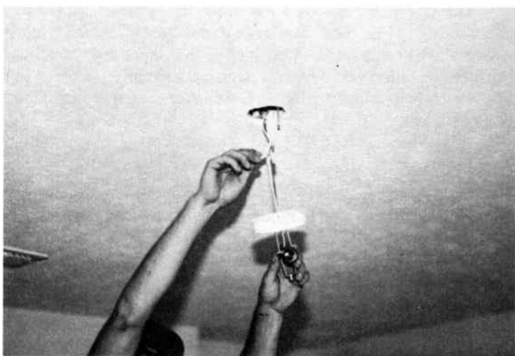
Fig. 6-57. Connecting a light fixture in the finished bedroom.
