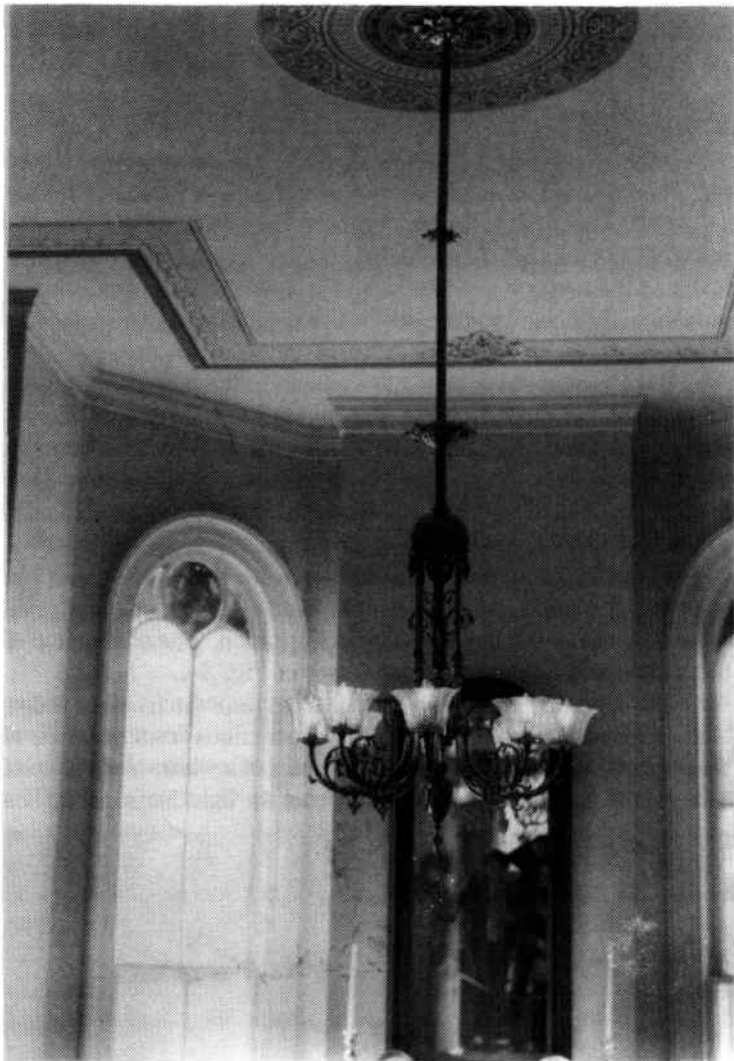
Fig. 8-3. An electrically wired gas light fixture.
