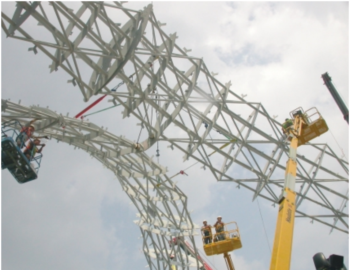
Category J Steelwork - The Whittle Arch, Coventry – Westbury Structures Ltd
