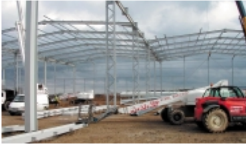
Multi-span portal frame during erection
