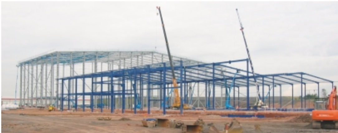
Screwfix Direct project, Stoke-on-Trent – Atlas Ward Structures Ltd
