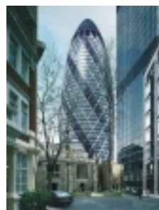
Swiss Re Building. Fire Engineers Arup Fire.
