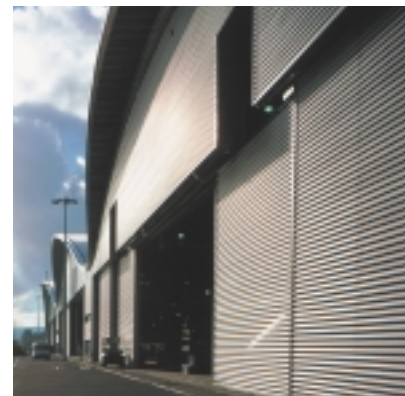
New Hangars for TAG Farnborough Airport - Rowecord Engineering Ltd
