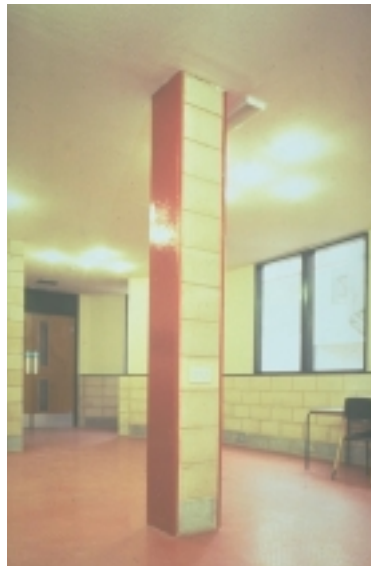
Block-filled column providing 30 minutes fire resistance
