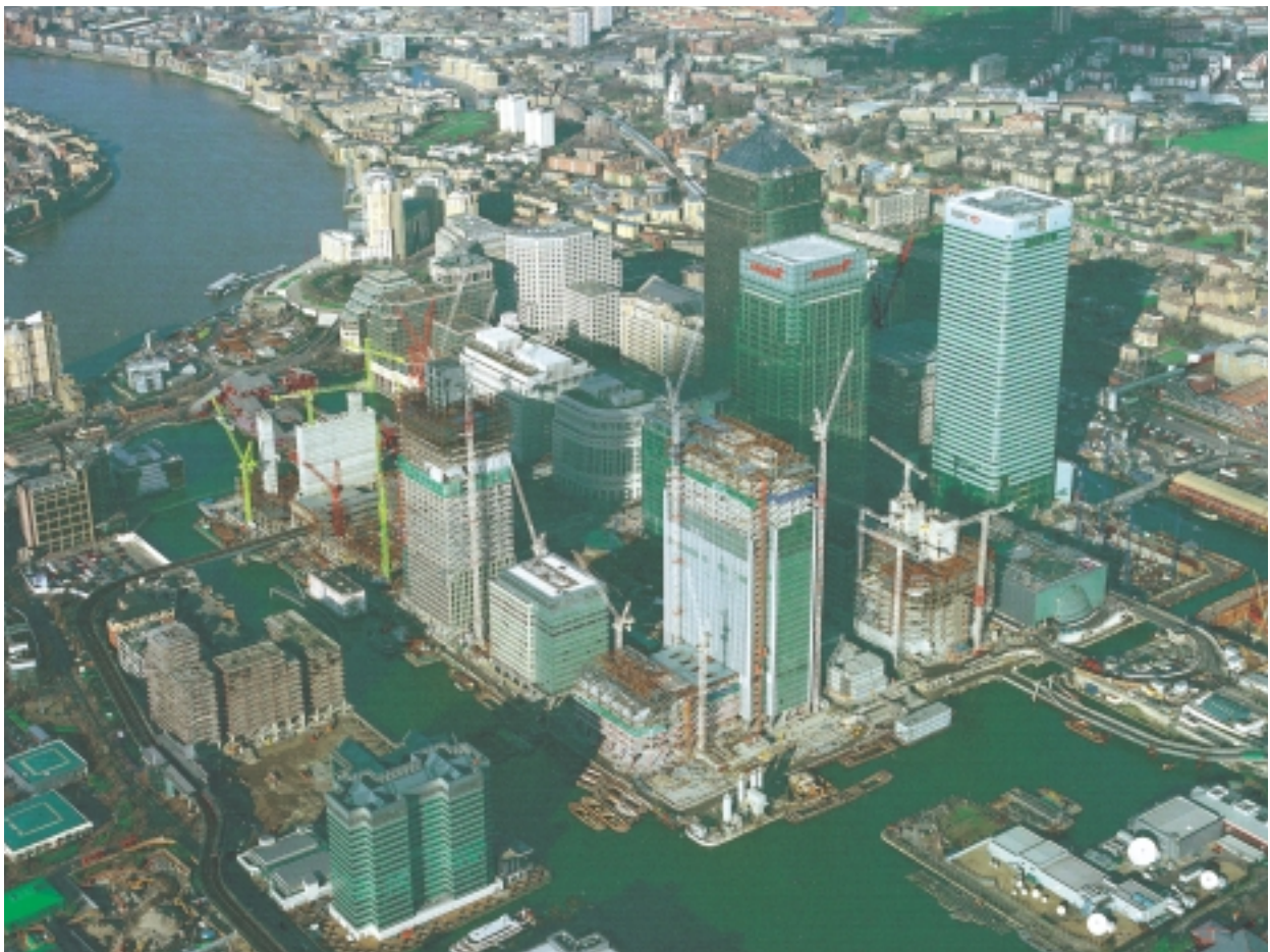
Canary Wharf, London – 72,300 tonnes of steelwork supplied by Cleveland Bridge UK Ltd
