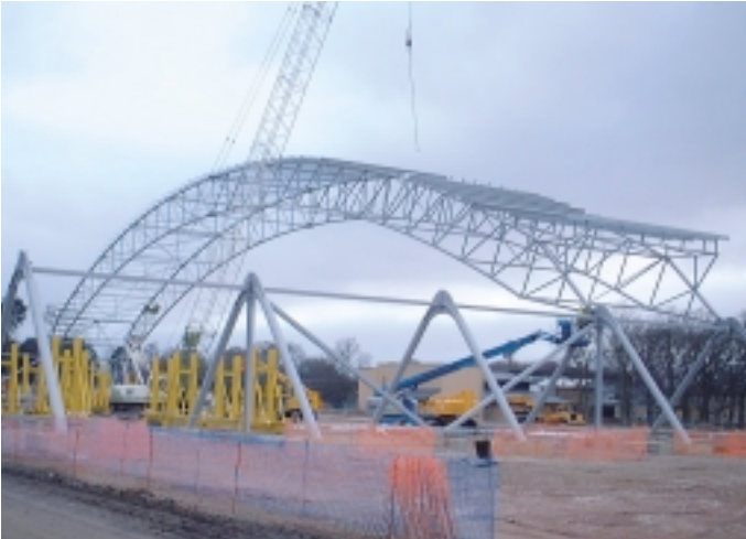
Category H Steelwork - TAG Aviation Hangar, Farnborough – Rowecord Engineering Ltd
