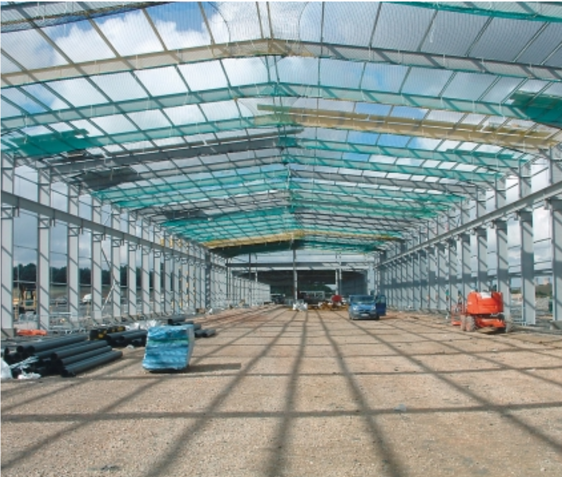
Category F Steelwork - Factory, Swadlincote – Bison Structures Ltd
