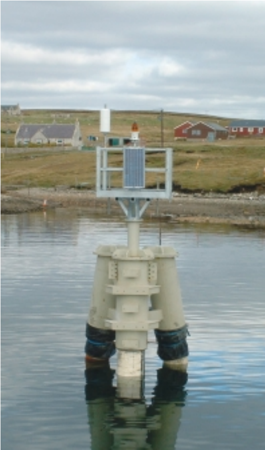
Category K Steelwork - Ulsta Navigation Tower, Shetland Isles - Dew Construction Ltd
