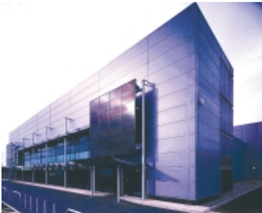
Baglan Energy Park was built on reclaimed industrial land, this air-tight, steel-framed and steel-clad building was constructed using local steelwork contractors.
