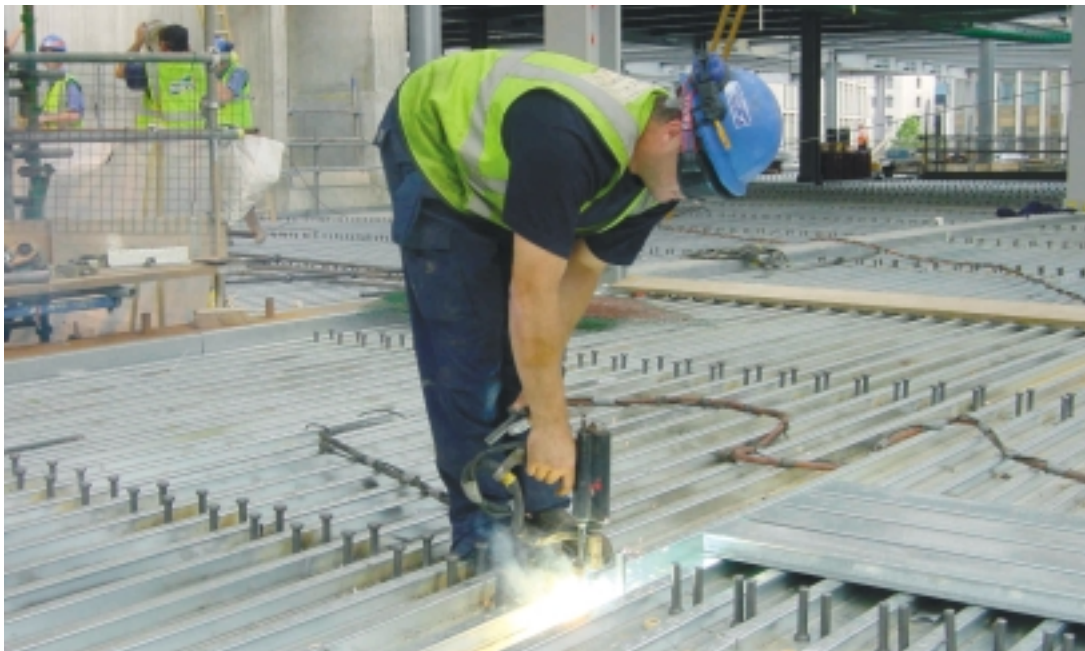
Baltic Quay, Gateshead – decking supplied by Structural Metal Decks Ltd
