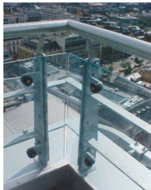
Category L Steelwork - Terrace Balustrading – Glentworth Fabrications Ltd
