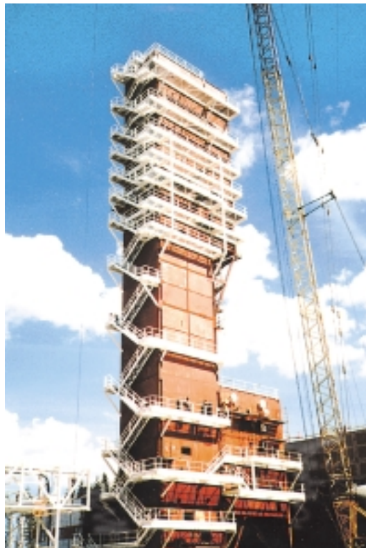
Category M Steelwork - BOC Plant - Bourne Steel Ltd
