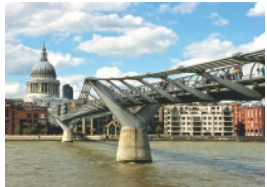
Figure 6.2 The crowd of pedestrians who had gathered for the opening of the Millennium Bridge in London caused a pronounced side-to-side vibration when they began to walk across
