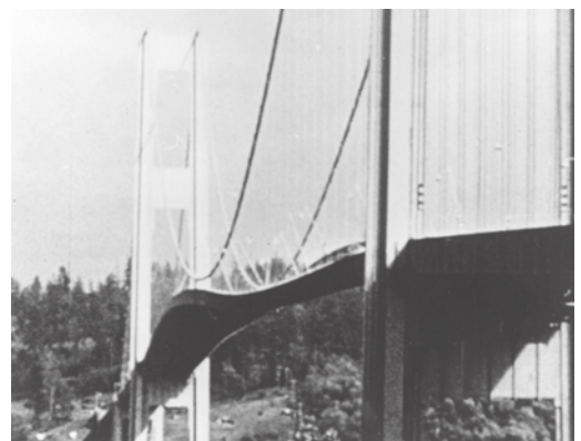
Figure 6.1 Wind-induced torsional vibration of the Tacoma Narrows bridge shortly before it collapsed
