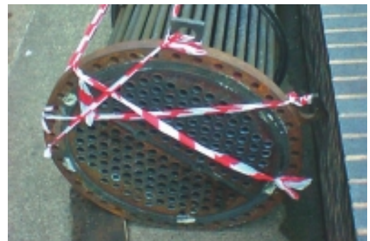
Figure 2.57 A typical shell-and-tube heat exchanger used in the hot water system at the University of Nottingham
