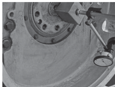
P3-8 Record the indicator reading at the SE location. Once again, make sure you note whether this reading occurs on the plus or minus side of the indicator zero point. Bar the engine to the NE reference point.
