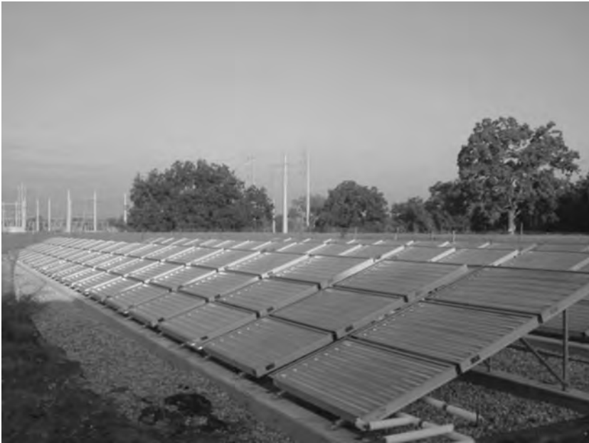
Figure 10.11 Parabolic solar heating system installation.
