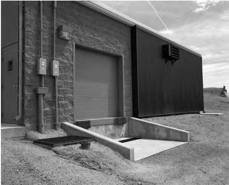
Figure 10.4 Passive solar power water heater in industrial use.
