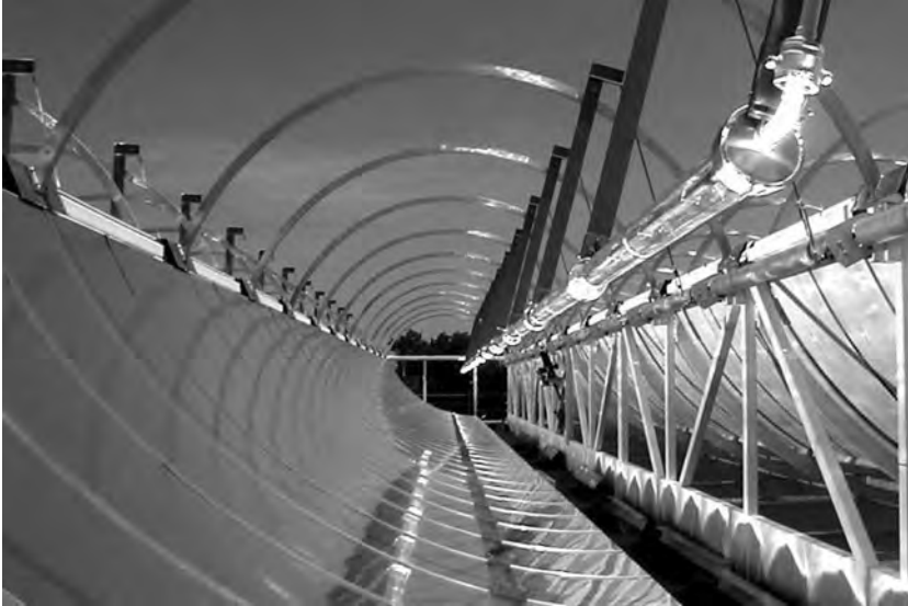
Figure 10.10 Solar parabolic heater installation. Photo courtesy of Solargenix.
