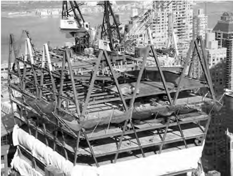
Figure 7.13 Digital structural members of new Hearst tower, New York, NY. Photo courtesy of Hearst Corporation.
