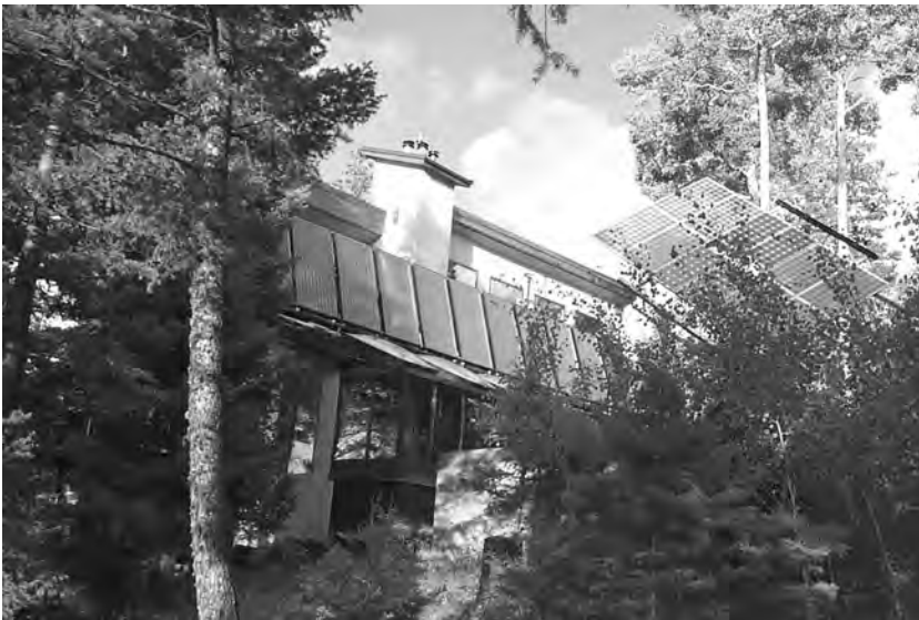
Figure 5.3 The Heavenly Retreat project (exterior view). Photo courtesy of Mr. Joel Goldblatt, New Mexico, United States.
