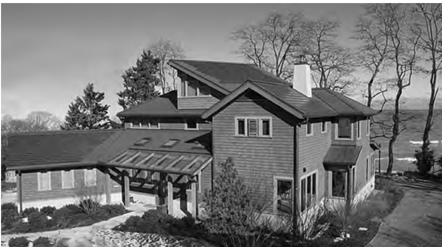
Figure 2.20 Application of SunSlate as roofing tile. Photo courtesy of Atlantis Energy Systems.
