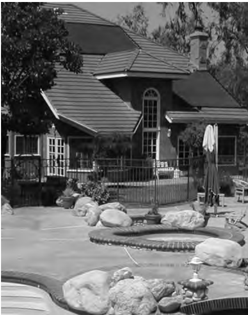
Figure 10.5 Rubber mat roof-mount solar water heater.
