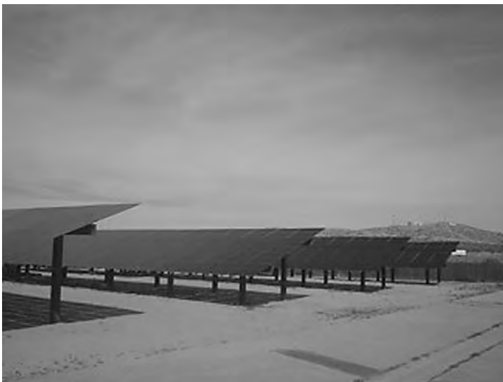
Figure 5.7 Boron solar photovoltaic farm. Photo courtesy of Grant Electric.
