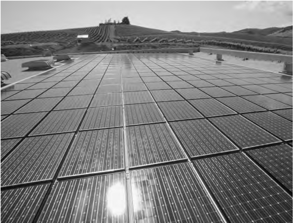
Figure B.33 Roof-mount non penetrating platform solar power system. Photo courtesy of Sun Power.
