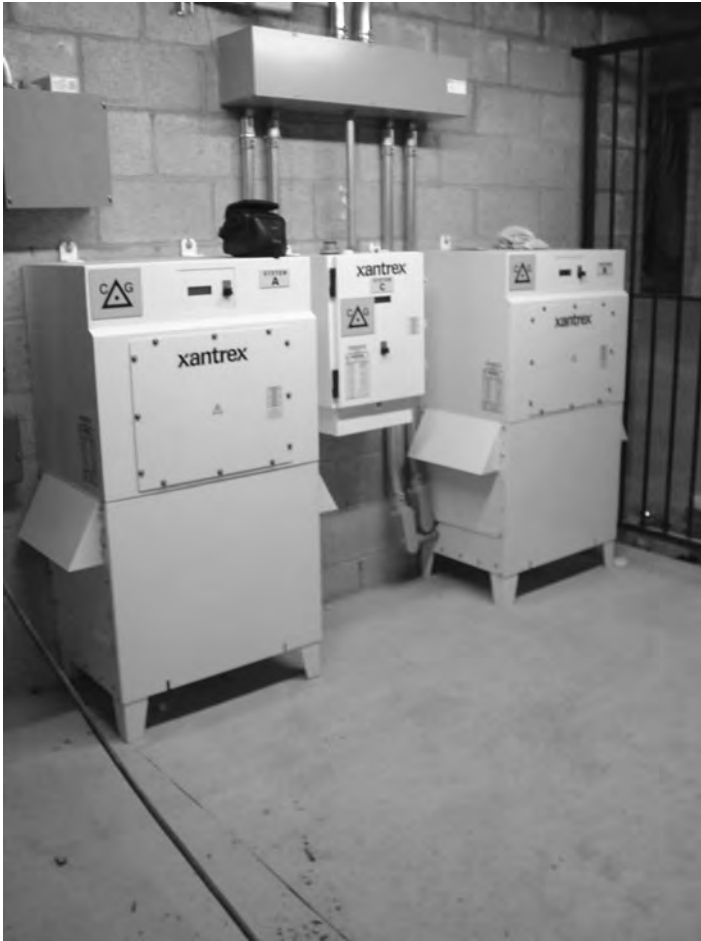
Figure 5.6 Inverter system, Arshag Dickranian School, Hollywood, California. Photo courtesy of Vector Delta Design Group, Inc.
