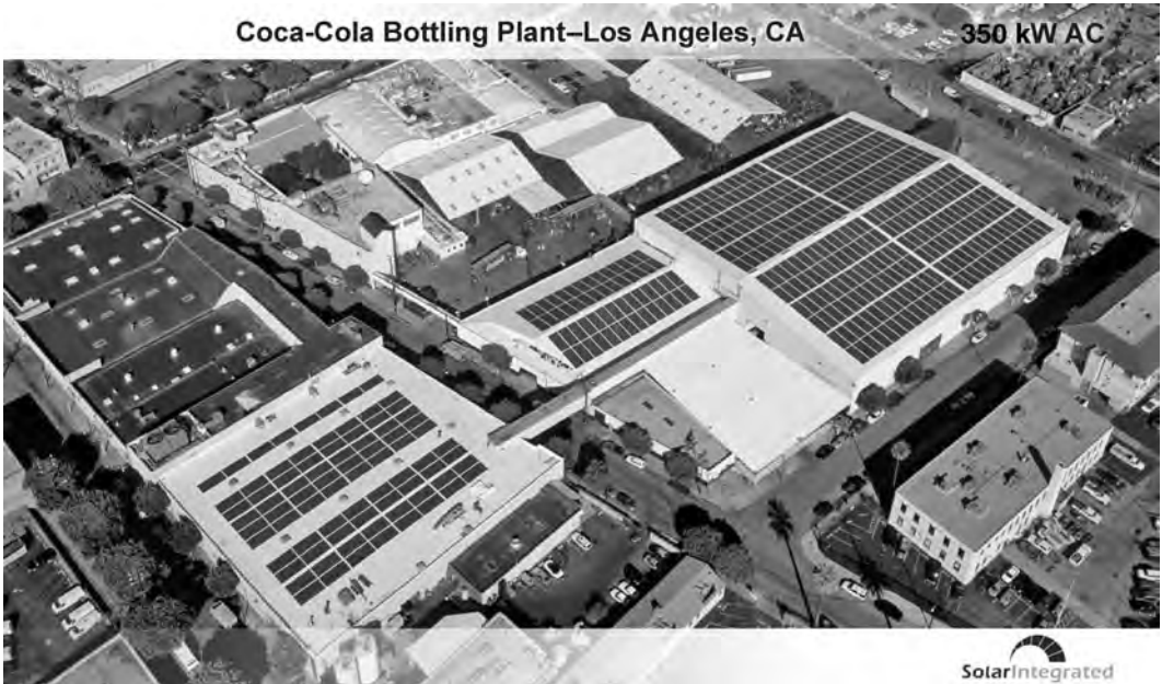
Figure 2.15 Coca-Cola Bottling Plant, Los Angeles, California. Photo courtesy of Solar Integrated Technologies.
