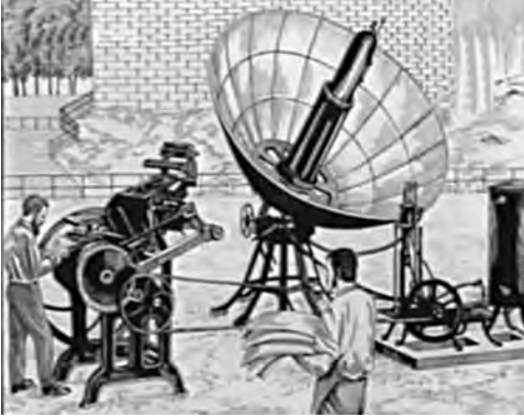
Figure 10.1 Historical use of passive solar energy to power a printing press.
