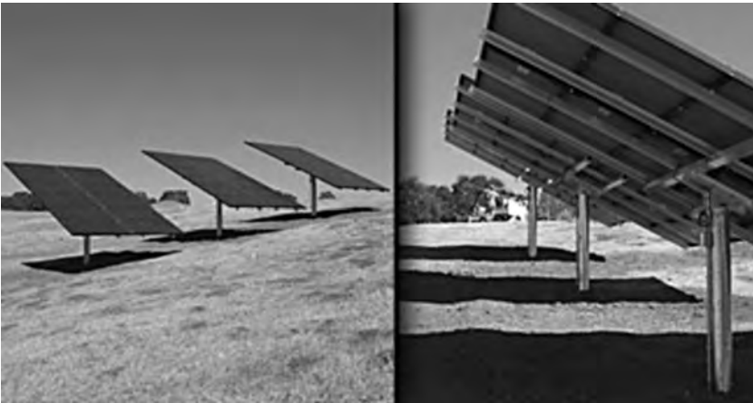
Figure B.5 Pipe-mounted semiadjustable tilt PV support structure.
