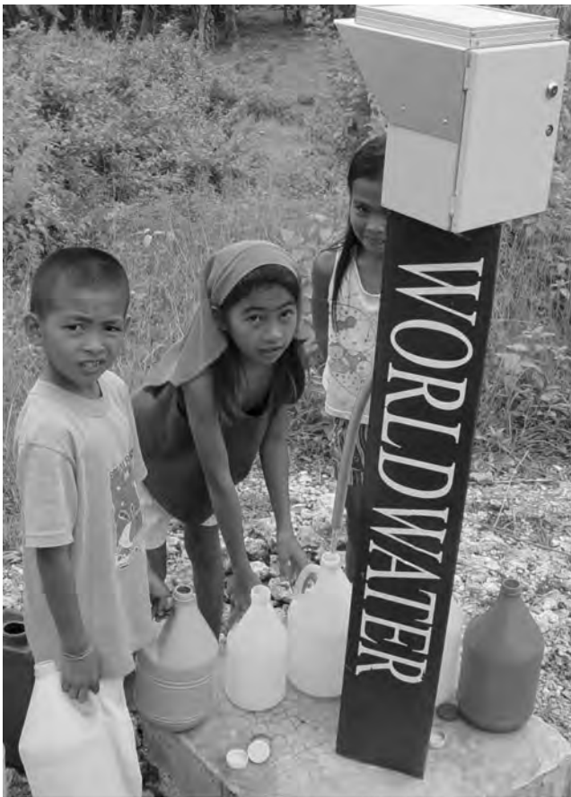
Figure 5.13 Submersible solar water pump in a rural Philippine village. Photo courtesy of WaterWorld & Power Corp.
