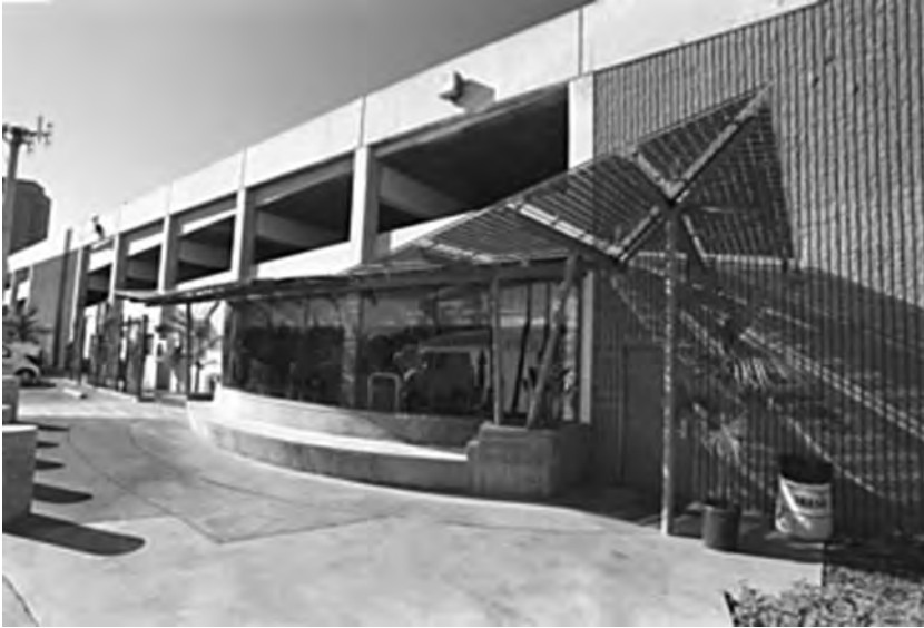
Figure B.29 Laminated glass BIPV solar power installation in commercial building entrance. Photo courtesy of Golden Solar Energy.
