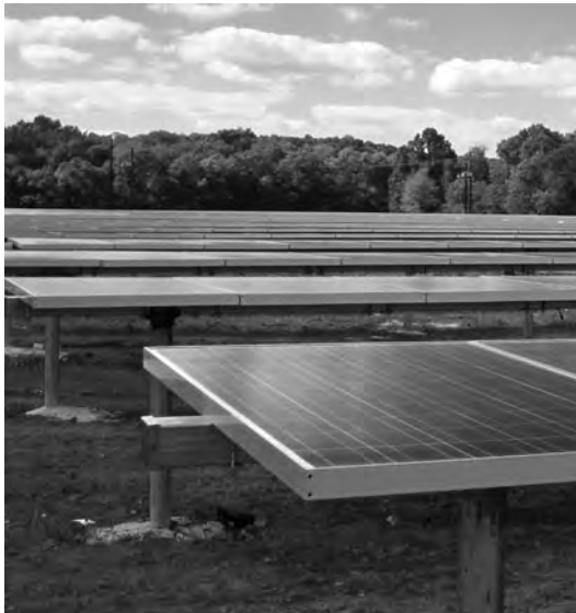
Figure B.35 Close-up of ground-mount single axis tracker solar power system. Photo
