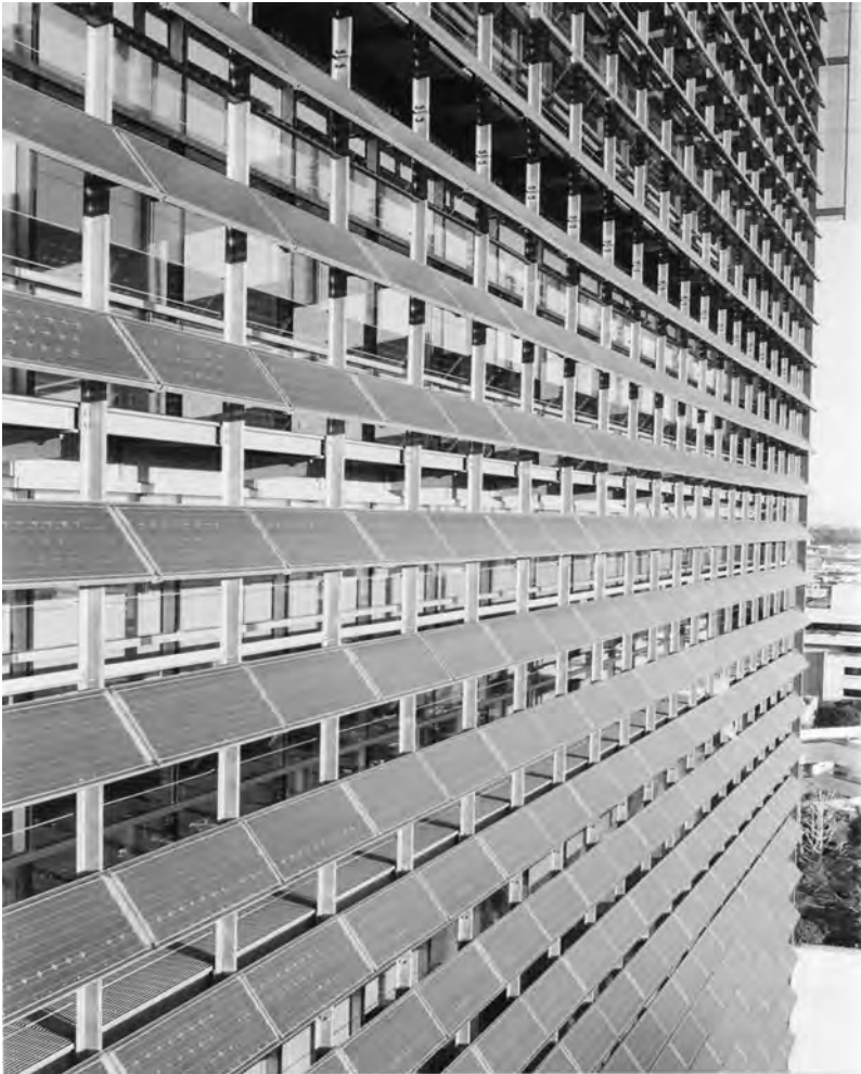
Figure 2.18 Application of BIPV as window canopy in CalTrans building, Los Angeles, California. Photo courtesy of Atlantis Energy Systems.
