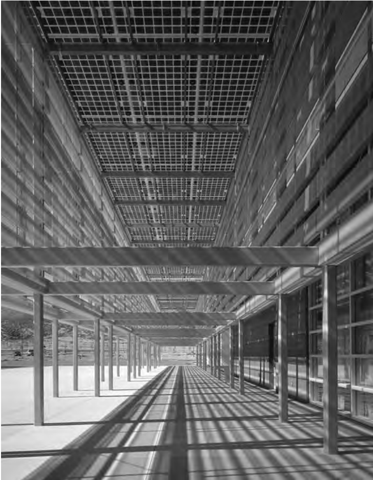
Figure 7.10 Water and Life Museum building-integrated (BIPV) solar power system. Engineered by Vector Delta Design Group, Inc. Photo courtesy of Fotoworks.
