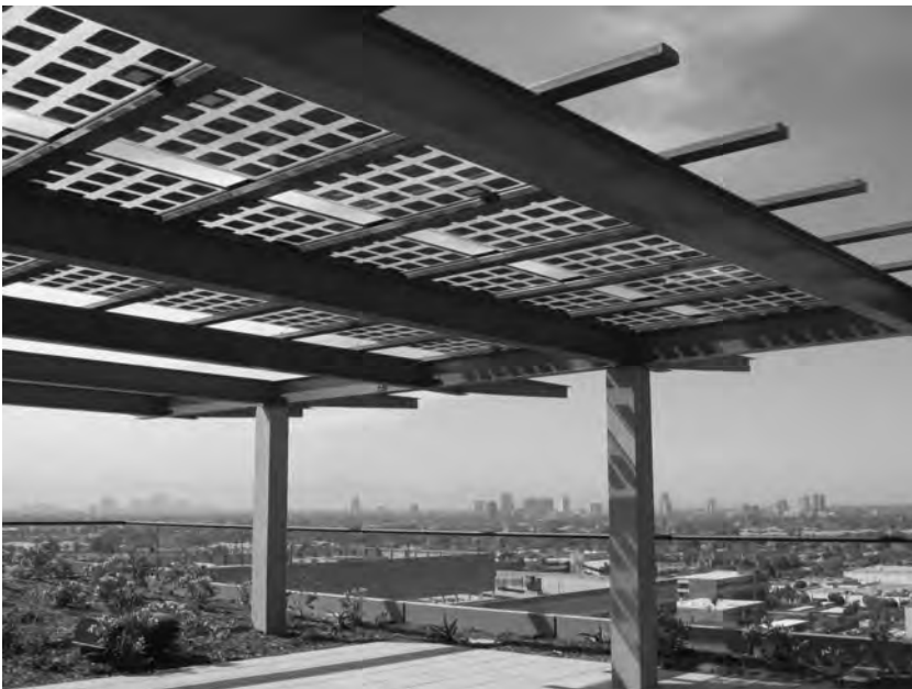
Figure B.30 BIPV solar power canopy installation. Photo courtesy of Atlantis Energy Systems.
