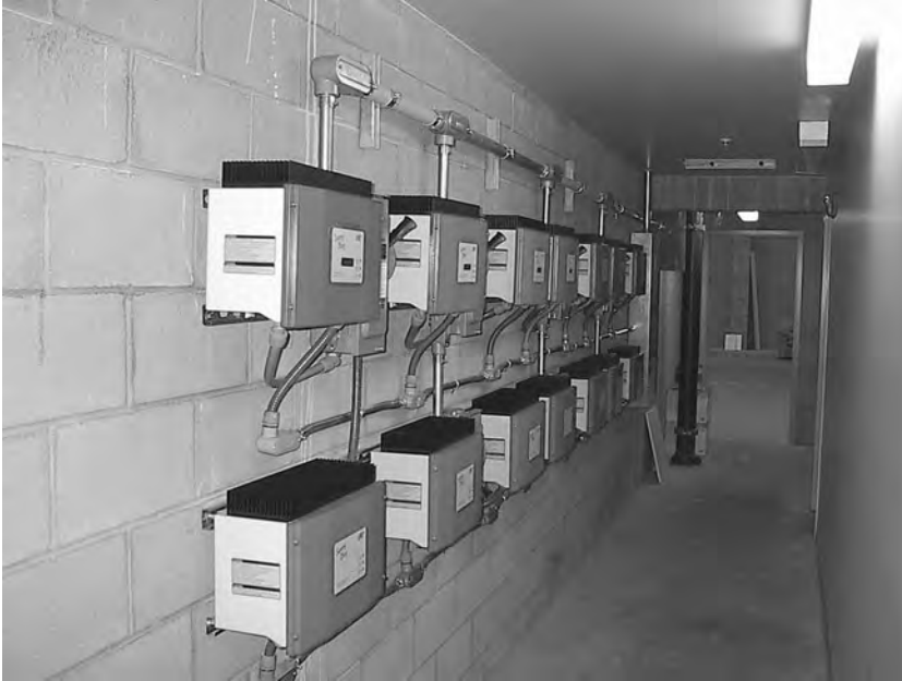
Figure 7.5 TriCom inverter system assemblies. Photograph courtesy of Solar Integrated Technologies, Los Angeles, CA.
