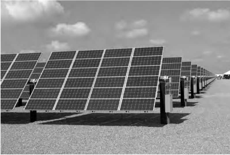
Figure 5.18 Large-scale single-axis solar farming system, Semitropic Water District, Wasco, California. Photo courtesy of SolarWorld.
