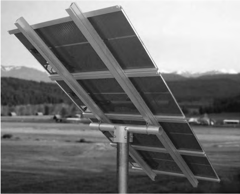
Figure B.11 Ground-mount fixed tilt PV support system hardware detail.
