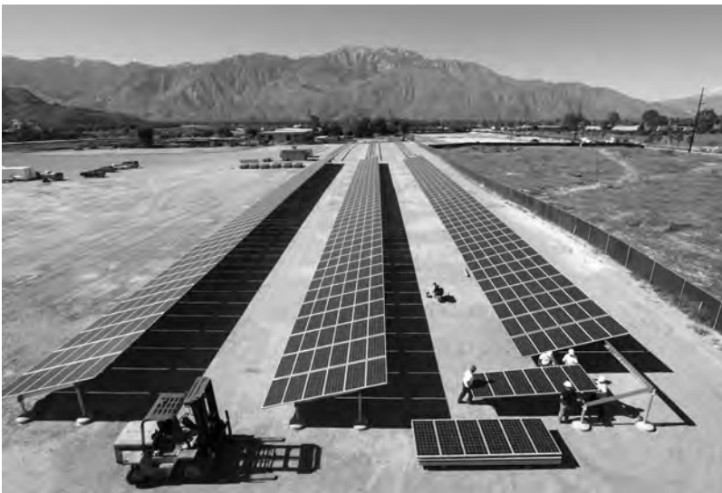
Figure 5.16 Large-scale solar pumping system in Imperial Valley California. Photo courtesy of WorldWater & Power Corporation.
