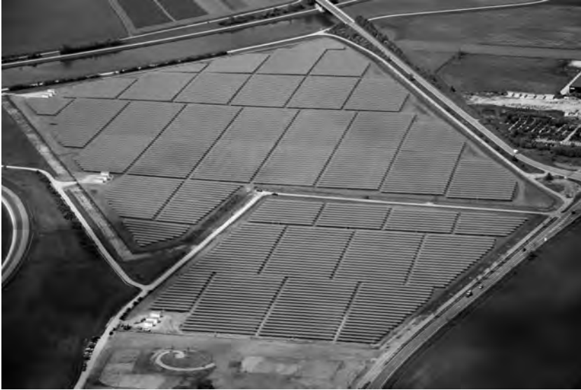
Figure B.32 10 single axis tracker Bavaria Solar Park. Photo courtesy of Sun Power.
