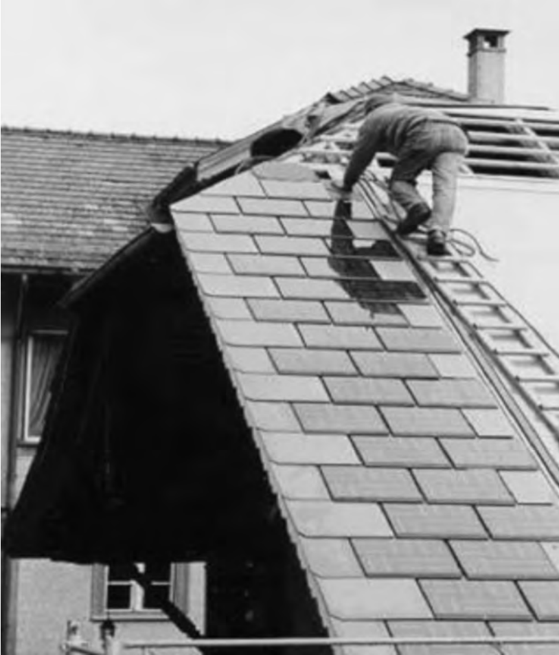
Figure B.26 Solar power roof slate installation in residential building roof structure. Photo courtesy of Atlantis Energy Systems.
