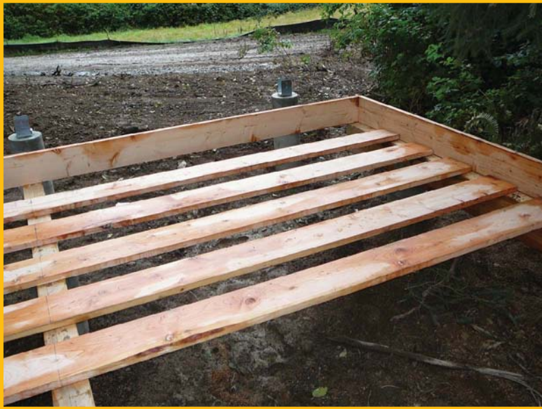
Joist spread and marked, ready to cut
