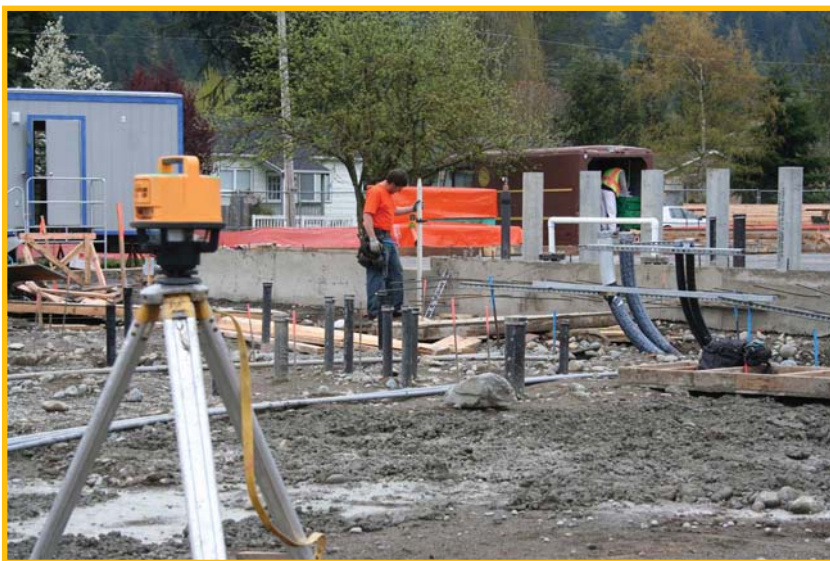
Checking level using a rotary laser.
