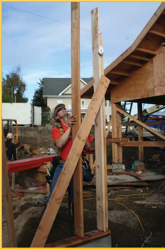
Chalk line at top of wall
