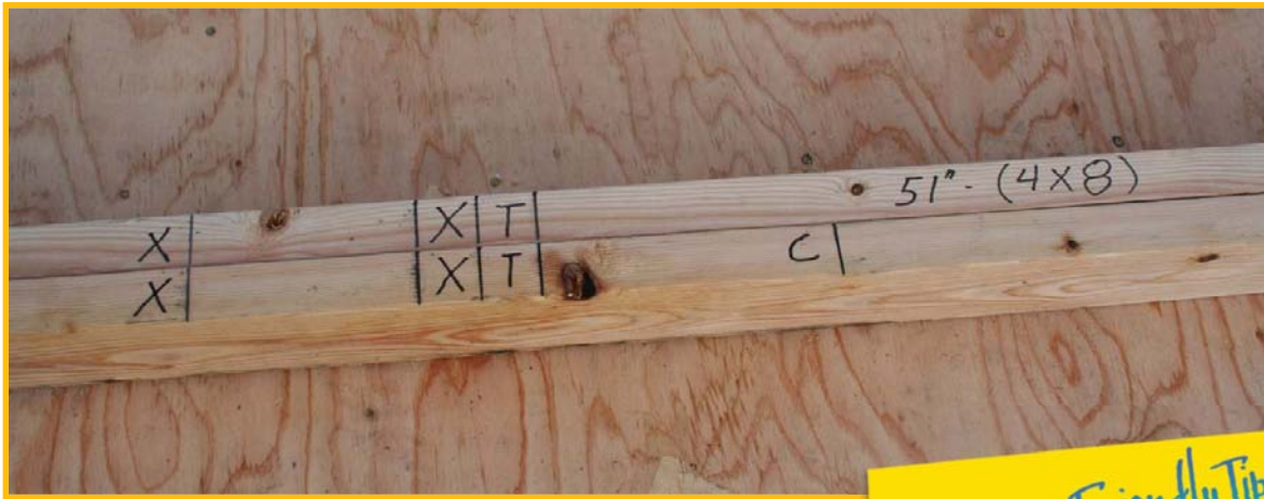
Wall plates positioned vertically for layout
