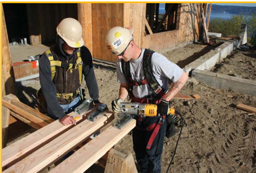
Teaching installing hold-downs after walls are built
