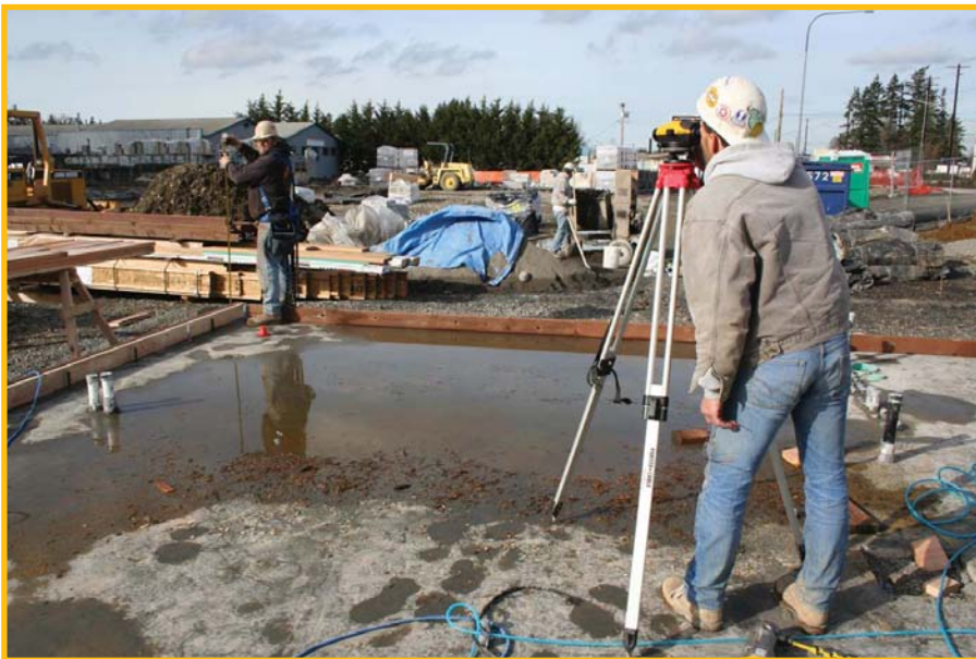
Transit line from concrete
