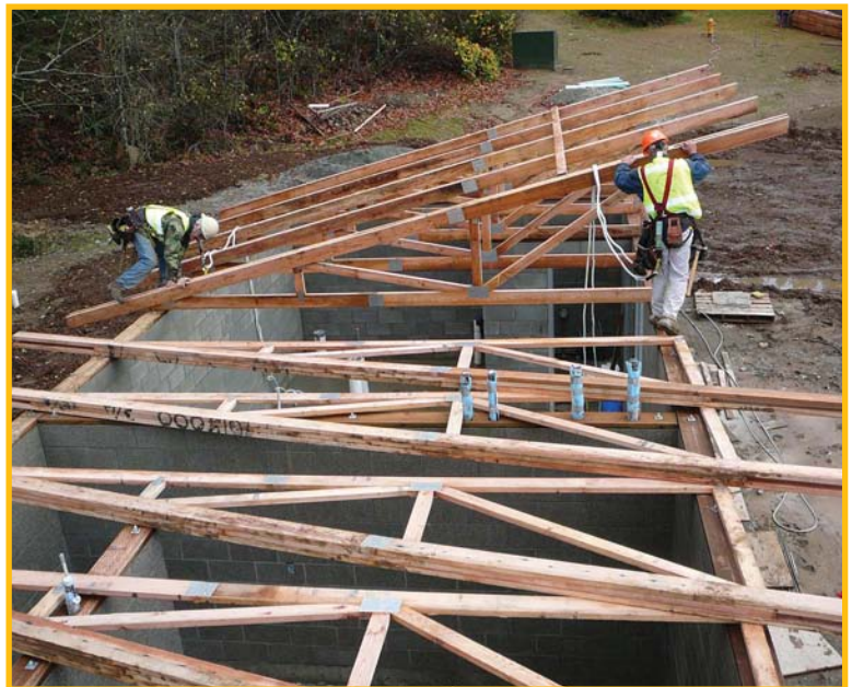
Rolling trusses into position
