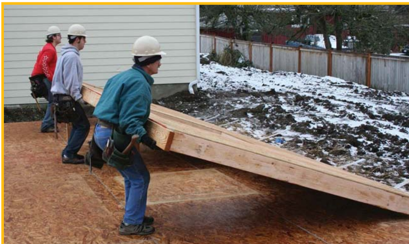
Proper lifting
