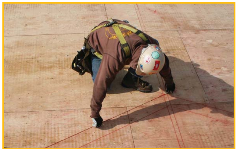
Chalking rafter lines
