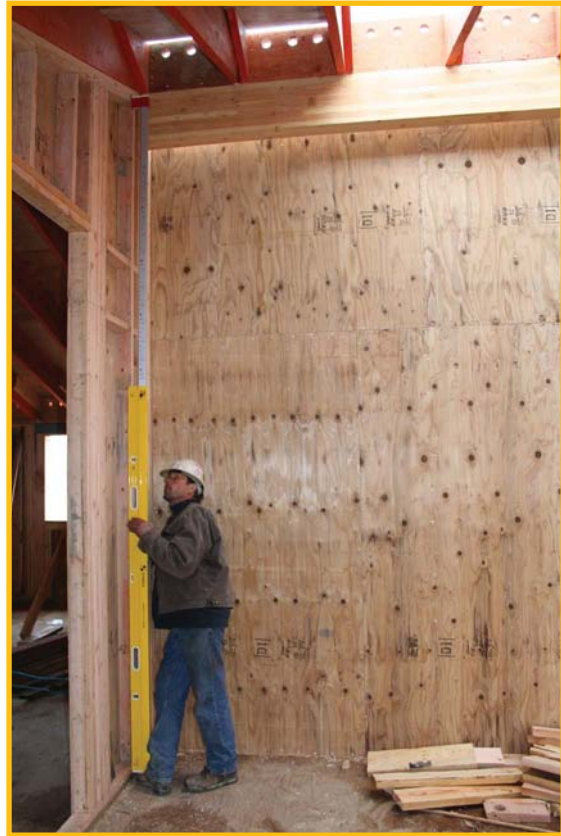
Plumbing tall wall with extending level.
