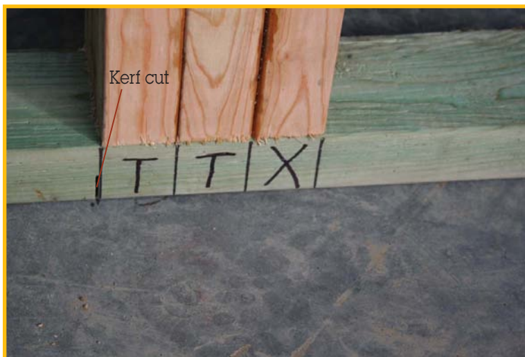
Kerf cut (threshold cut)
