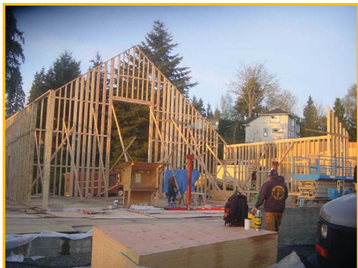
An unsheathed rake wall
