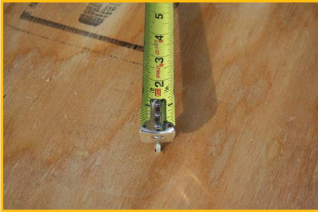
End of tape hooked to a partially set nail
