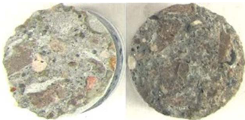
Figure 6.9 Failures of concrete substrate.
