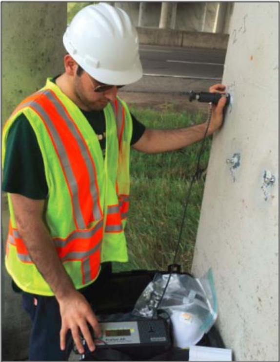
Figure 7.3 Adhesive bond testing on as-built structure.
