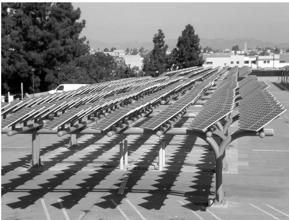
Figure 6.24 Parking space shade structure made of photovoltaic panels
