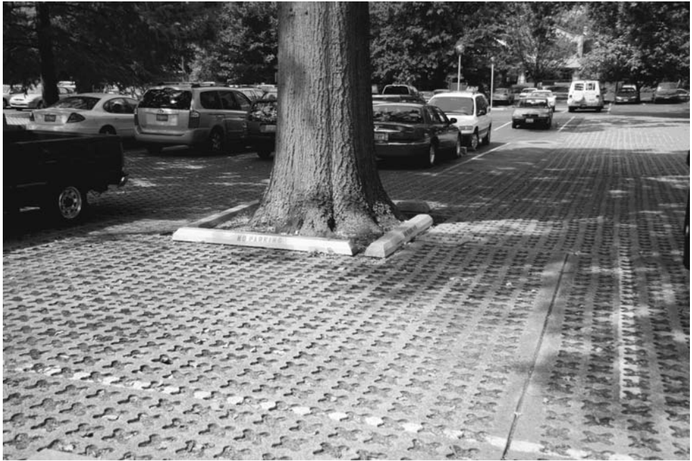
Figure 4.23a Pervious paving, Missouri Botanical Gardens
