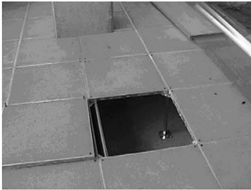
Figure 4.27 Image of a UFAD installation
