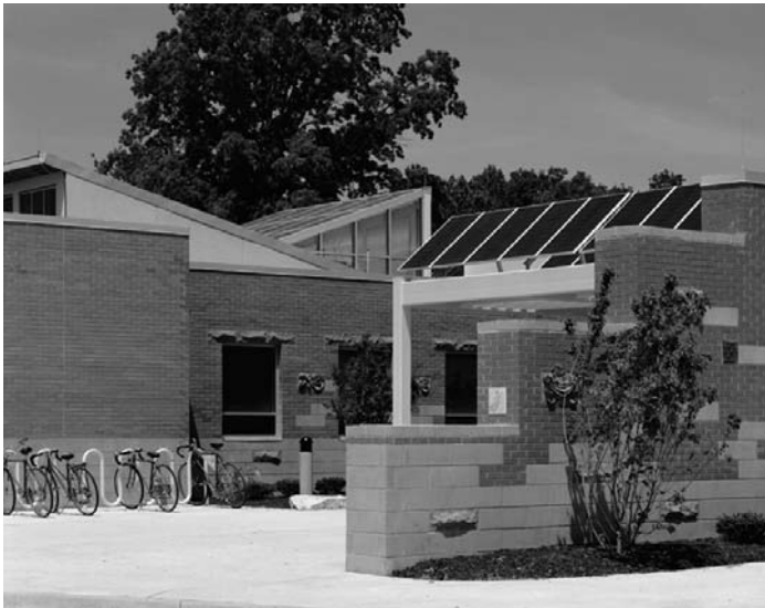
Figure 4.31b Crystalline PV array at Anita B. Gorman Conservation Discovery Center
