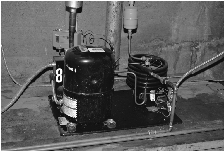
FIGURE 13-1 Hermetically sealed water-cooled compressor.
