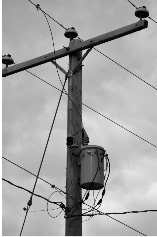
FIGURE 5-3 Single-phase transformer.
