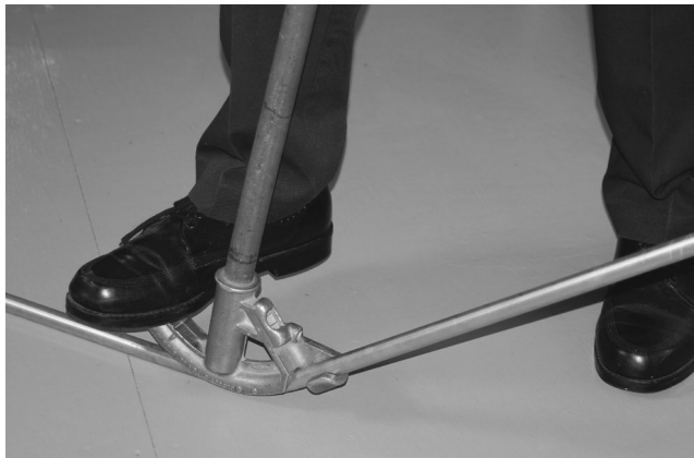
FIGURE 4-1 Bending electrical metallic tubing.
