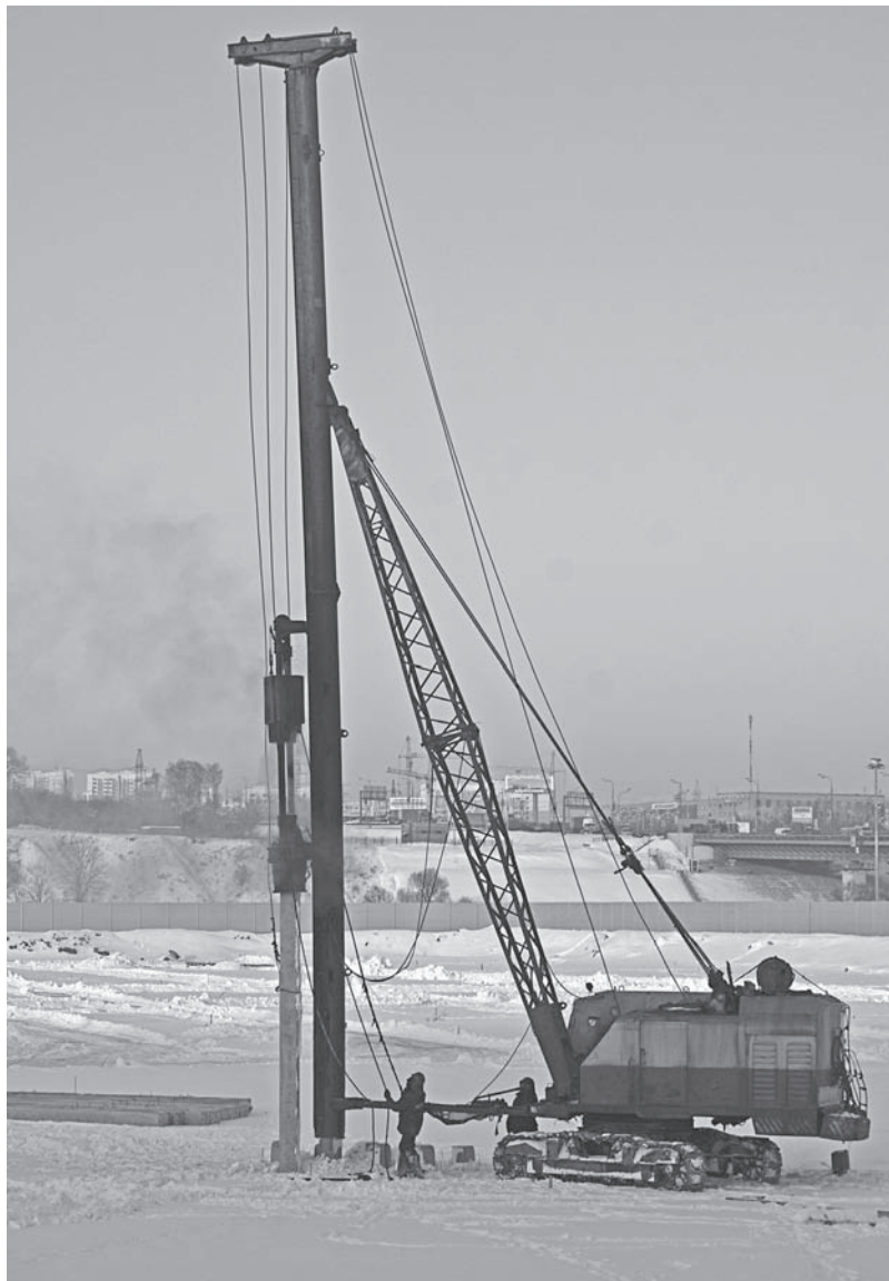
FIGURE 10-23 Pile installation.
