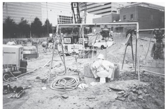
FIGURE 10-33 Setup for a shaft field inspection.
