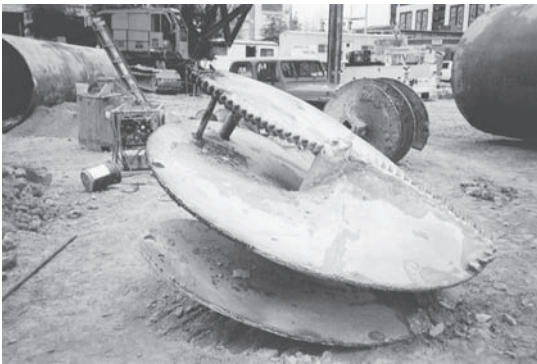
FIGURE 10-30 Large auger used in drilled shaft construction.
