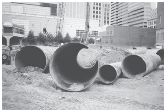
FIGURE 10-31 Steel casing used in drilled shaft construction.
