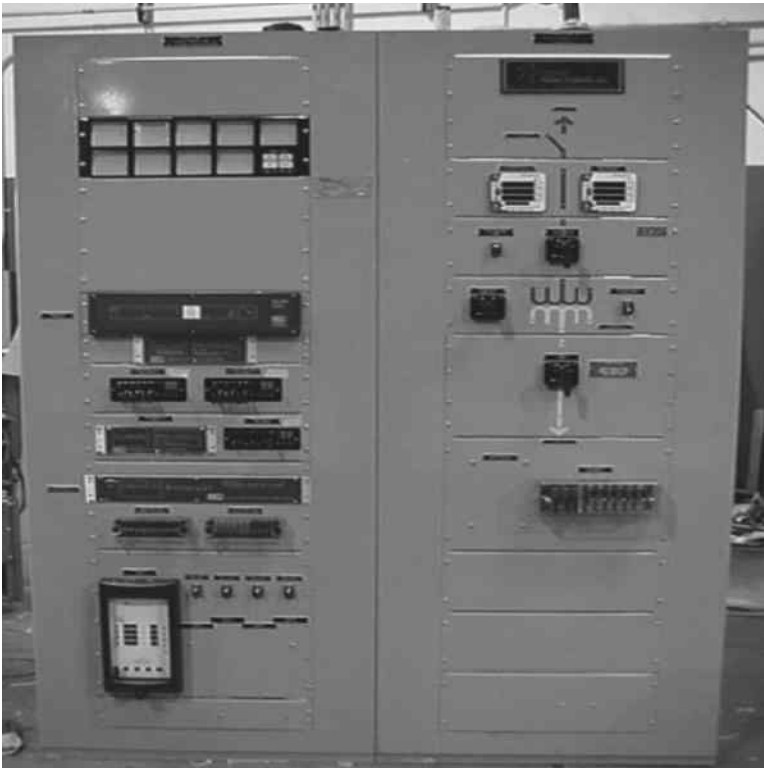
FIGURE 7.12 Generator switchgear (15 kV) in self-contained enclosure. (From Myers Power Products, Inc. With permission.)
