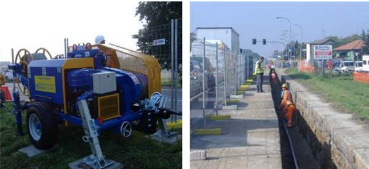
Figure 1.26 (Turbigo–Rho mixed line) Pulling winch and cable laying (Courtesy of TERNA)
