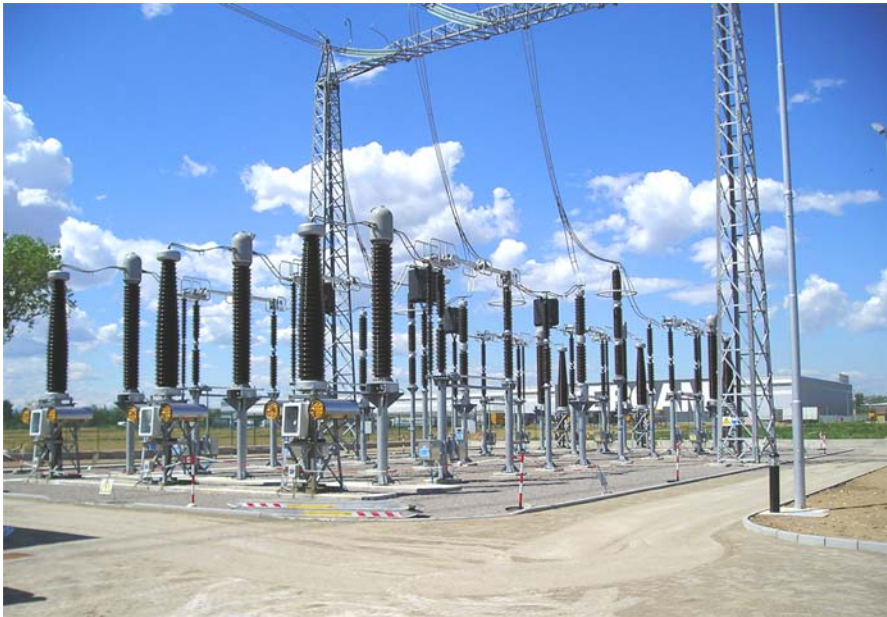
Figure 1.28 (Turbigo–Rho mixed line) Transition compound (Courtesy of TERNA)
