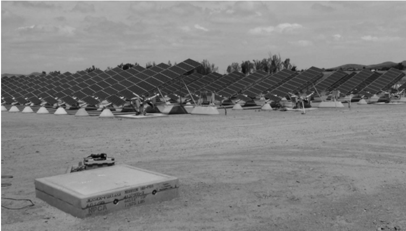
Figure 3.16. A single axis tracking solar power system
