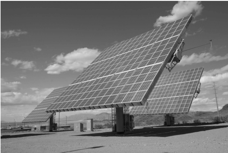
Figure 3.17. A dual axis tracking solar power system. Source: Photo courtesy of AMONIX
