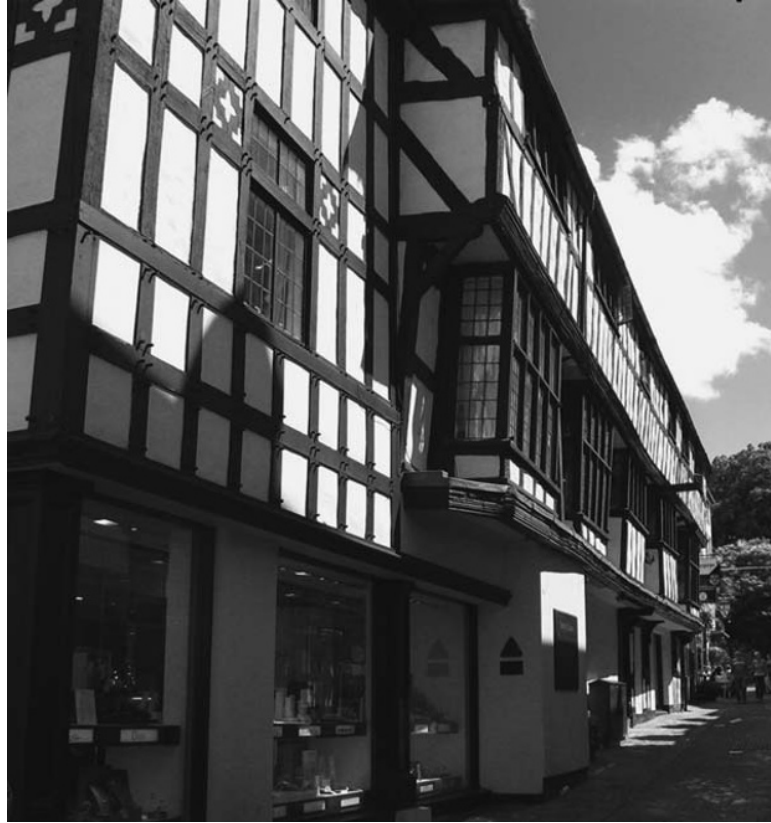
Figure 3.19: Photograph showing the jetty floor of a timber frame building in Shrewsbury.
