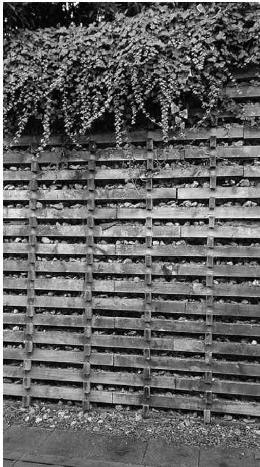
Figure 16.6: Photograph showing a typical crib wall construction.
