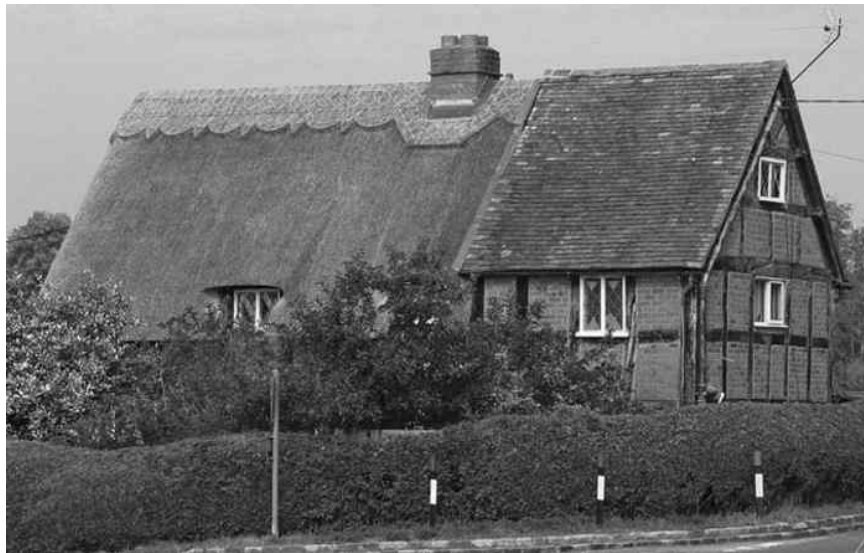
Figure 10.10: Photograph showing a house with a part thatched and part tiled roof.
