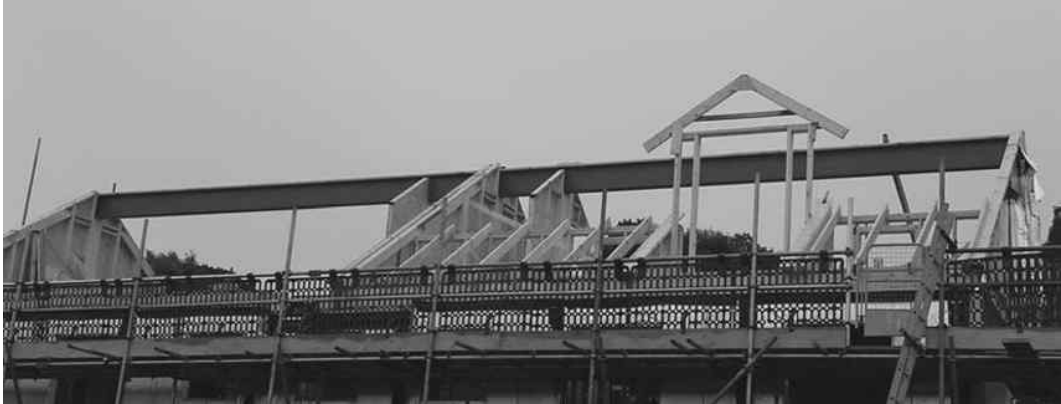
Figure 10.9: Photograph of a steel ridge beam.
