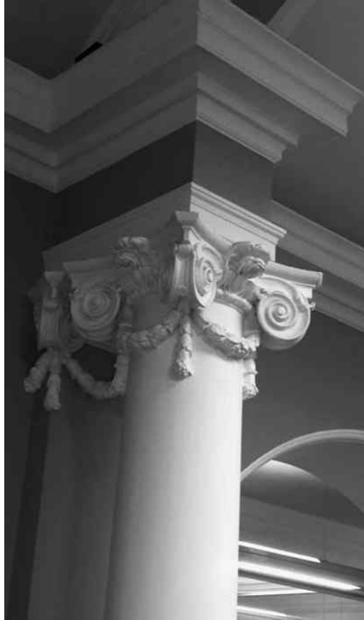
Figure 11.10: Photograph showing a Corinthian column.
