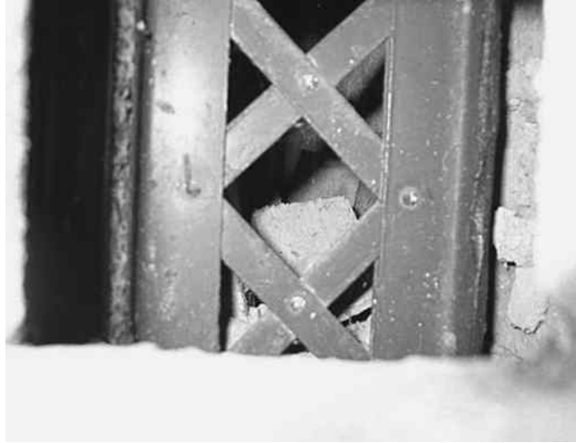
Figure 3.29: Photograph showing exposed frame of a steel frame house.
