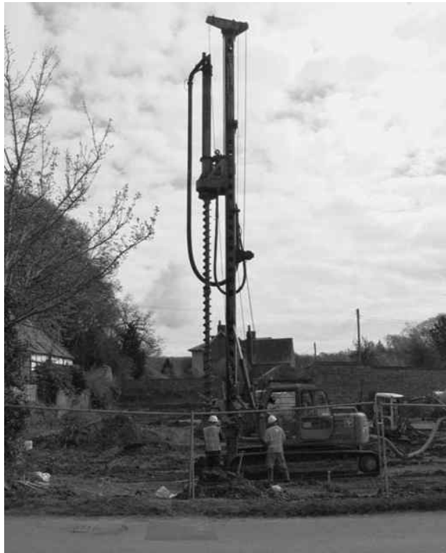
Figure 7.6: Photograph showing a bored pile foundation activity.
