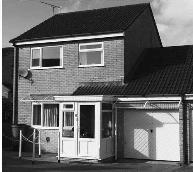
Figure 1.14: A typical 1980s house on a residential estate using calcium silicate bricks.
