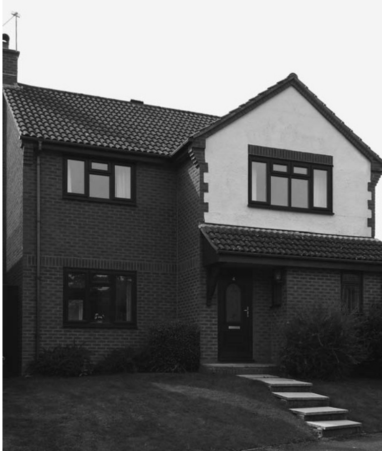
Figure 1.13: A typical 1980s house on a residential estate using clay bricks with a rendered gable.
