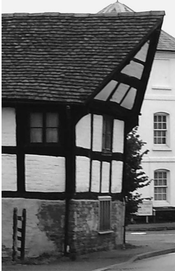
Figure 3.16: Photograph of raked gable wall of a house in Herefordshire.
