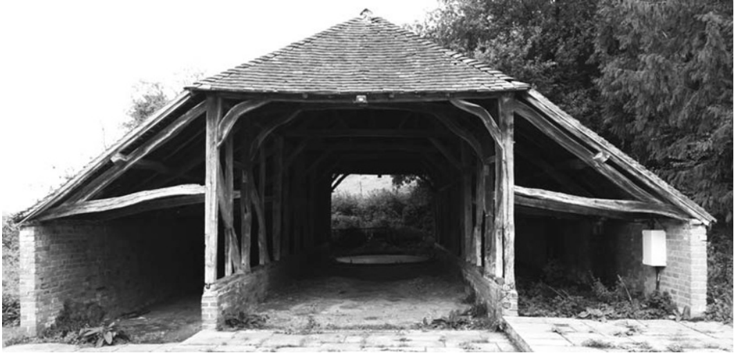
Figure 3.20: An aisled barn construction.
