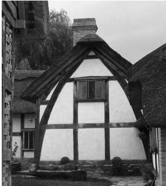
Figure 1.1: Photograph of typical cruck construction in Herefordshire.
