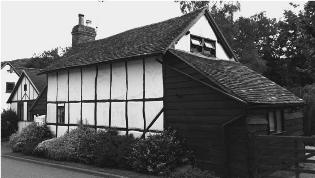
Figure 3.11: A traditional timber frame from the 1700s.
