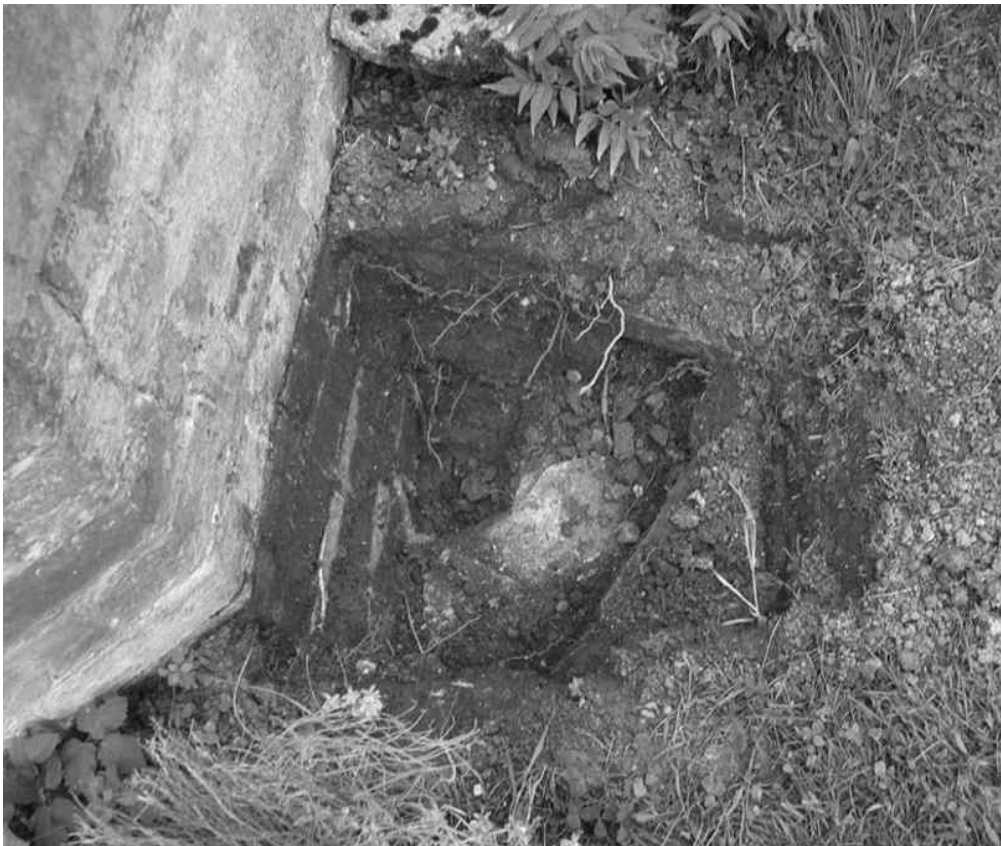
Figure 7.3: Photograph showing a stepped brick foundation in a Georgian property.
