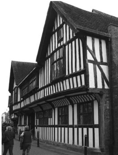
Figure 3.7: A building in Greyfriars, Worcester dating to 1480.
