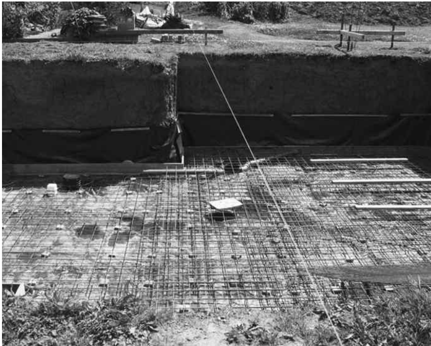
Figure 16.8: Showing the commencement of a basement structure.
