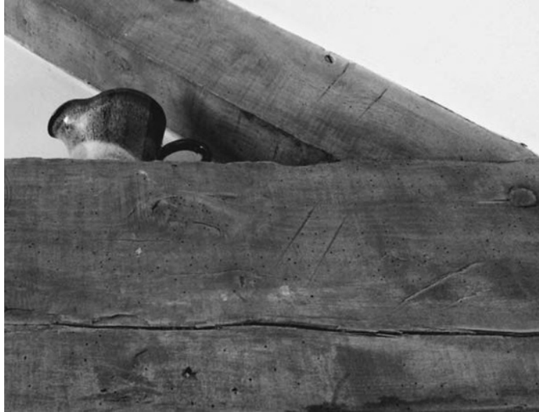
Figure 3.18: Photograph showing roman numbering of joint on a timber truss.
