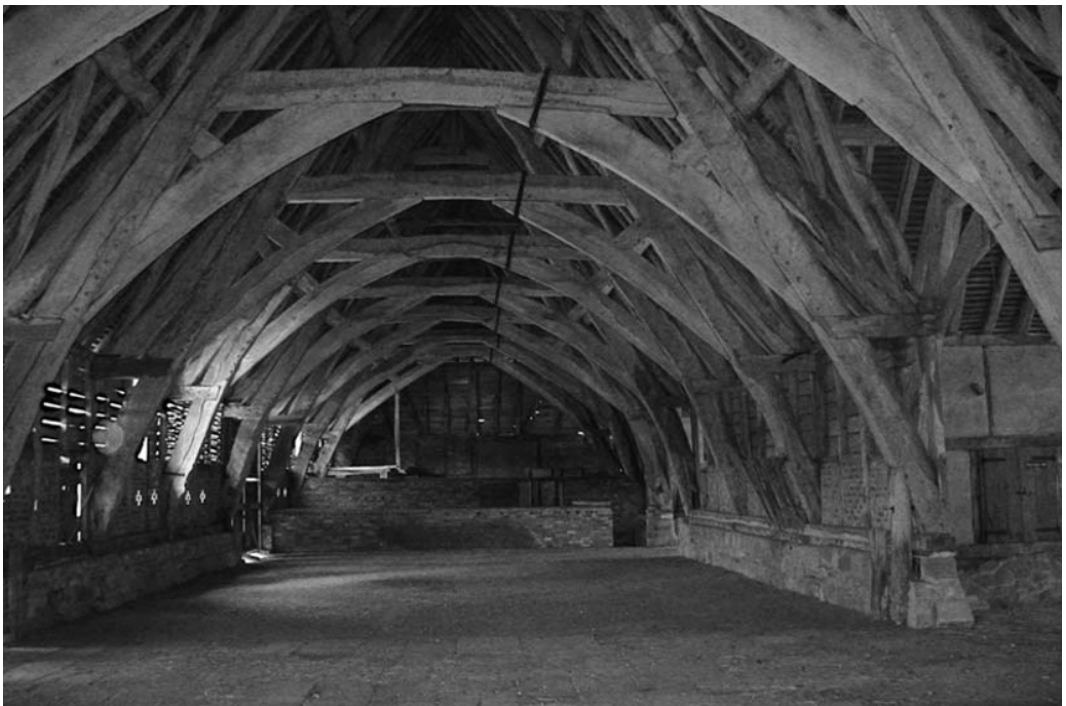
Figure 3.6: Internal cruck frame of Leigh Court Barn in Worcestershire, dated 1300.
