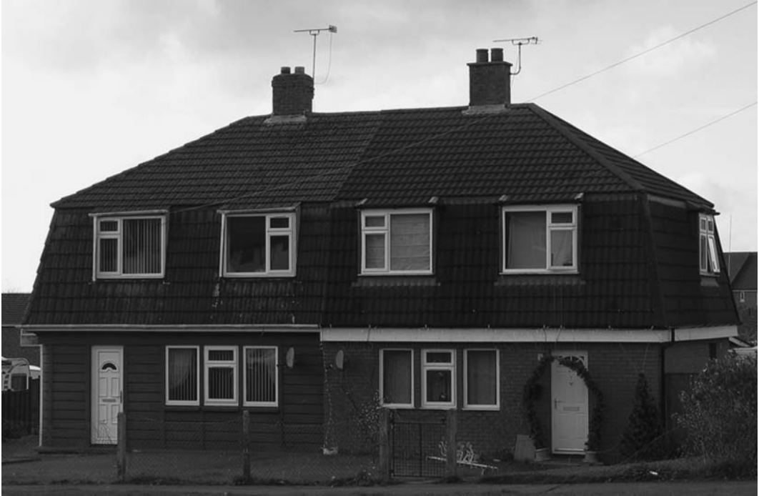
Figure 1.10: Photograph of a Cornish dwelling which was a particular type of prefabricated concrete house.
