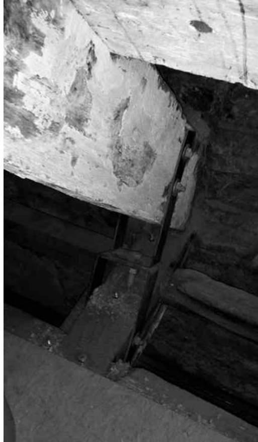
Figure 17.2: Showing steel plate to strengthen a truss connection.
