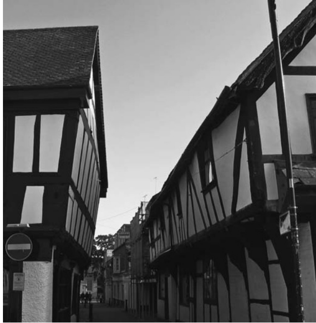
Figure 1.2: Photograph showing the close proximity of timber frame housing in Leominster, increasing the risk of fire.
