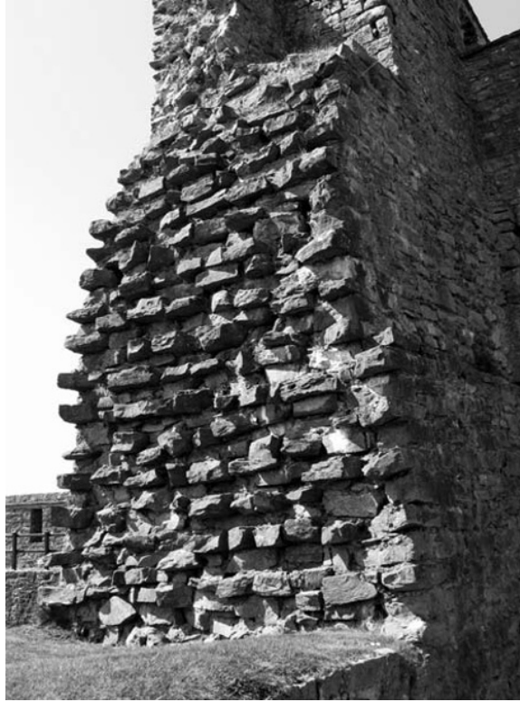
Figure 3.21: Photograph of a large rubble wall in cross-section at Pembroke Castle.
