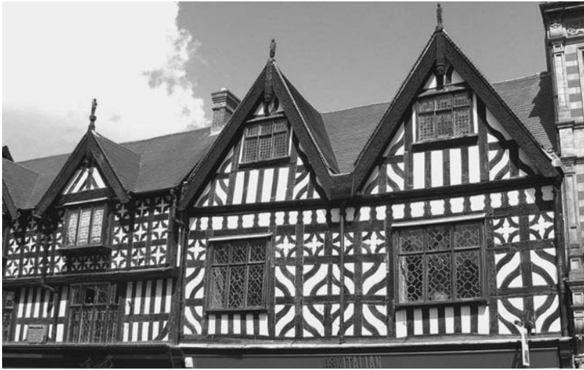
Figure 3.9: A timber frame construction in Shrewsbury circa 1500s with decorative timber panelling.
