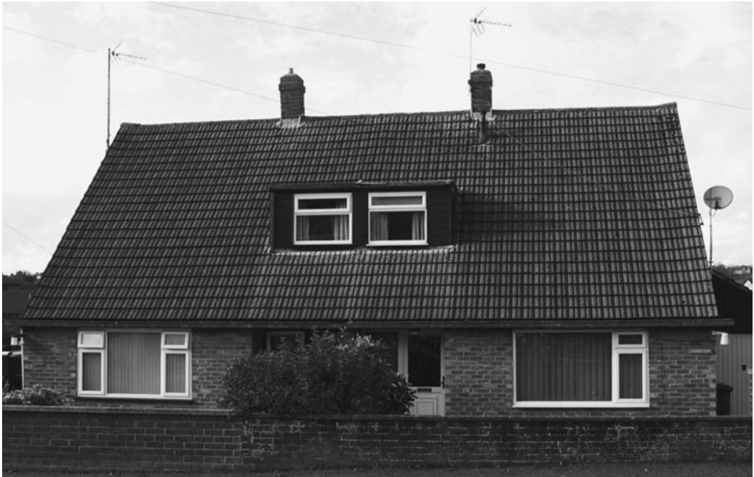
Figure 1.12: Photograph of a typical 1960s bungalow.
