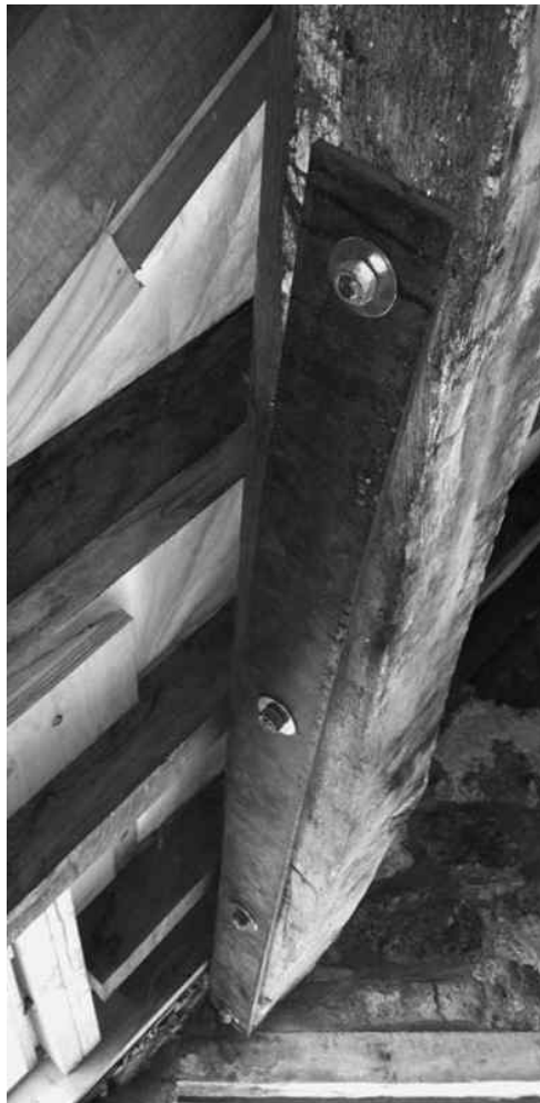
Figure 17.1: Showing steel plate to strengthen purlin.
