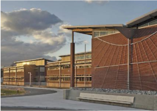
Figure 3.3 A butterfly roof offers an aesthetically pleasing and convenient catchment point for rainwater. To educate students about the environment, a sculpture at Poquoson Elementary School uses rainwater to wash a sundial during wet weather. (©Prakash Patell/Poquoson Elementary School—VMDO Architects)
