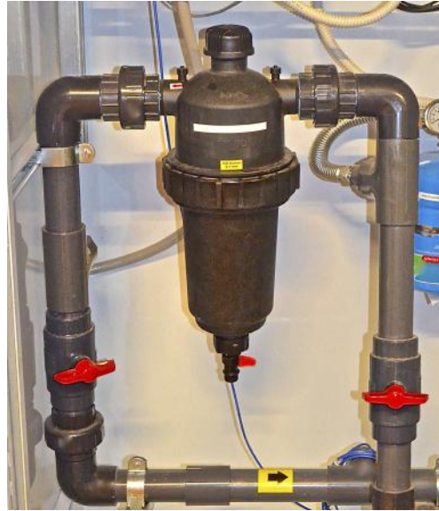
Figure 5.10a Inline filtration units are chosen for desired size of filtration screen as well as flow rate. (Eddie Van Giesen)
