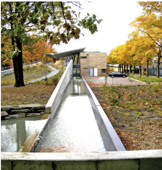
Figure 1.1 Queens Botanical Garden Visitor and Administration Center is an example of integrated rainwater harvesting system design.
