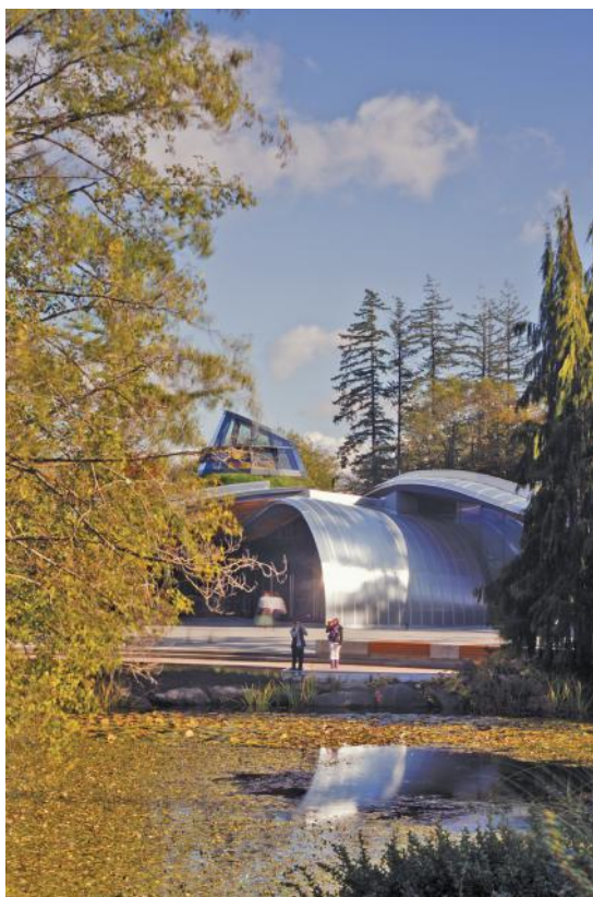
Figure 2.10 Design goals were set at an early stage of planning for the VanDusen Botanical Gardens in Vancouver, Canada. This project was designed by Perkins+Will to be in harmony with nature, and is currently targeting the Living Building Challenge™ and LEED®-Canada NC Platinum. Rainwater is filtered and used for the building’s water requirements and various integrated stormwater drainage systems designed to meet local and stringent best management practices for the community. (Nic Lehoux/Courtesy: Perkins+Will)
