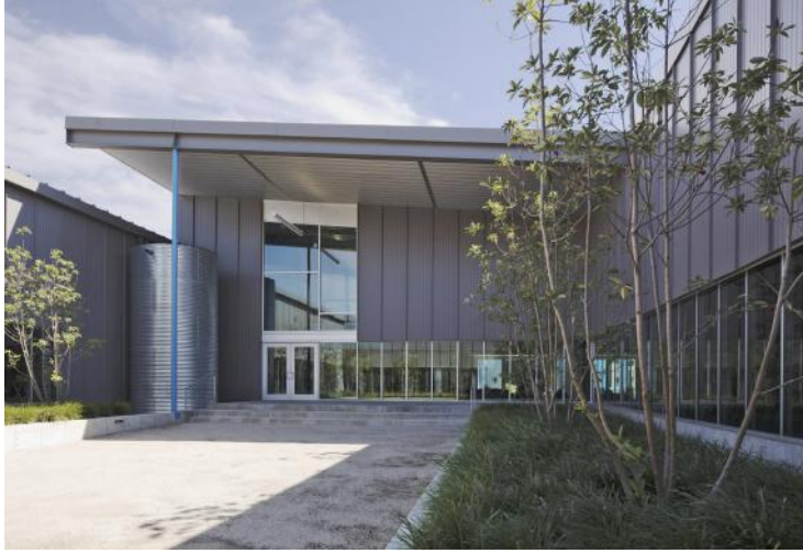
Figure 4.25 Aboveground tanks at Posty Cards Manufacturing Plant in Kansas City, Missouri (Aaron Daugherty Photography)
