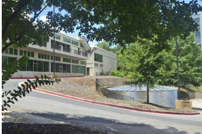
Figure 4.3 An integrated system provides water for toilet flushing and cooling towers at the University of Georgia Visual Arts Building. (Viviane Van Giesen)
