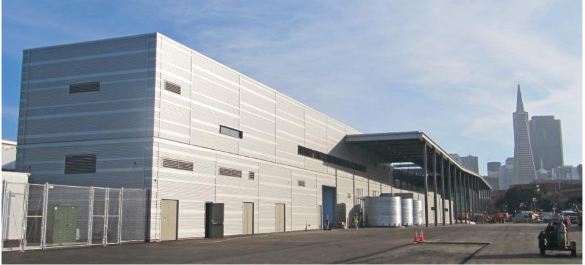
Figure C.5 Three aboveground rainwater collection tanks are sized to meet both the monthly demand for toilet flushing and for irrigation. ( KMD ARCHITECTS & PFAU LONG ARCHITECTURE, a Joint Venture )
