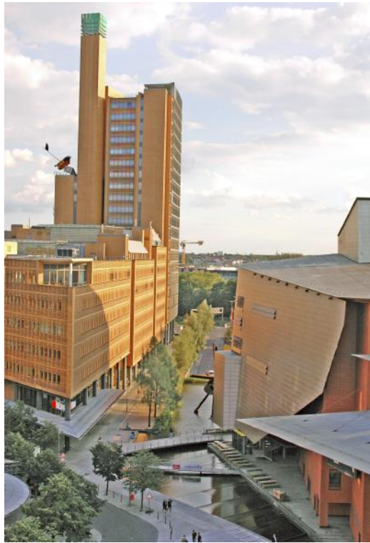
Figure 1.11 Potsdamer Platz integrates various water system designs to create a vibrant natural area in the heart of Berlin. ( Judy Leel/Atelier Dreiseitl )
