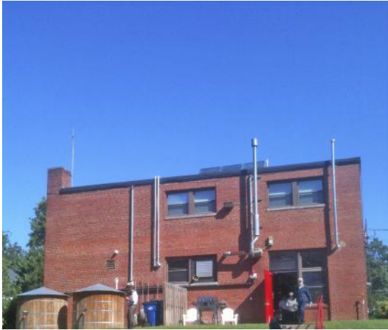
Figure 3.6 The rainwater collection system for Fire Station Number 6 in Raleigh, North Carolina, provides water for toilet flushing. (Celeste Allen Novak, Architect)
