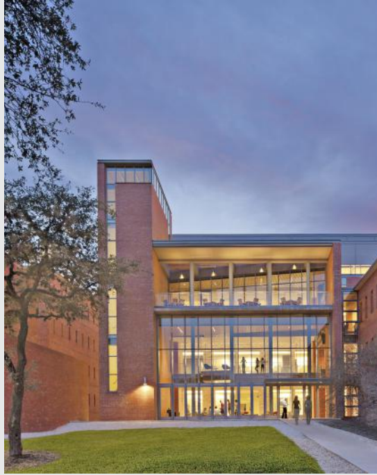
Figure 3.11 Center for the Sciences and Innovation at Trinity University, San Antonio, Texas, designed by EYP Architecture & Engineering and RVK Architects. The reclaimed water system using condensate collection earned 6 points in the Water Efficiency category toward LEED® Gold. ( Robert Benson Photography )
