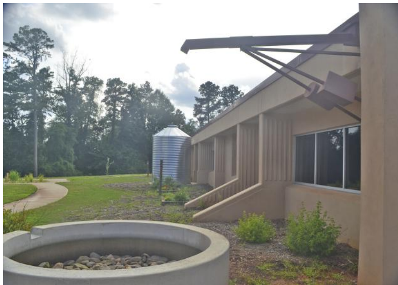
Figure 4.14 Exaggerated conveyance provides educational opportunities in a rain garden/rainwater harvesting system for the Fowler Drive Elementary School, Athens, Georgia. ( Viviane Van Giesen )
