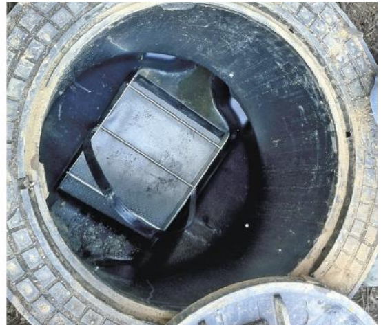
Figures 5.9a and b An example of a cascading type filter when dirty (a) and then after cleaning (b). (Eddie Van Giesen)
