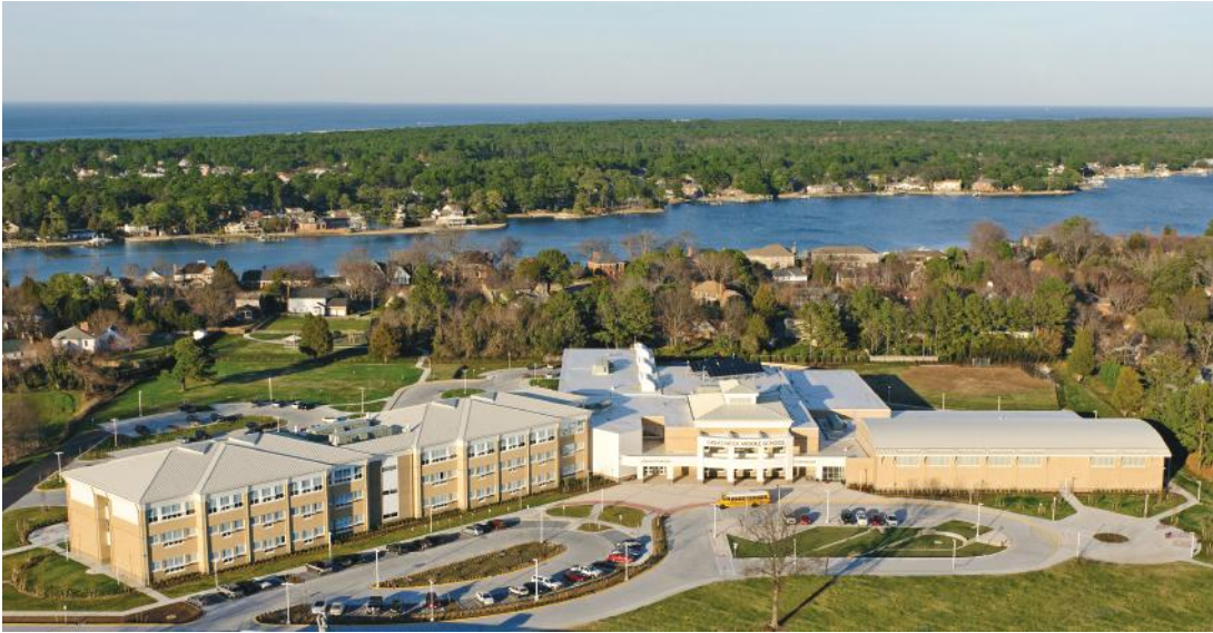
Figure C.10 Great Neck Middle School in Virginia Beach is one of several Virginia schools that collects rainwater for toilet flushing and irrigation. (Photographed by Steve Budman Photography, Courtesy of Waller, Todd & Sadler Architects, Inc)
