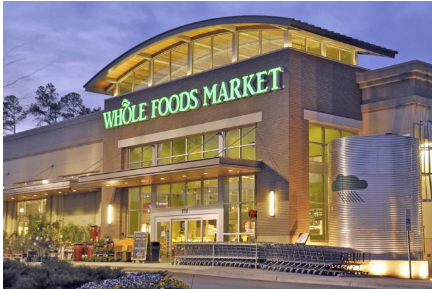
Figure 1.19 Project sustainability is showcased by this exterior rainwater harvesting cistern that stores water for toilet flushing in store restrooms. ( Regency Centers )
