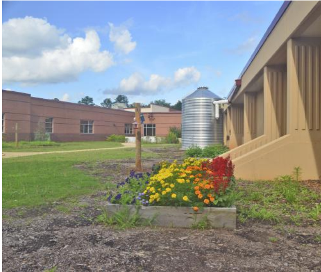
Figure 3.9 Rainwater collection tanks are visible from an outdoor classroom that incorporates a demonstration rain garden at Fowler Drive Elementary School. (Eddie Van Giesen)
