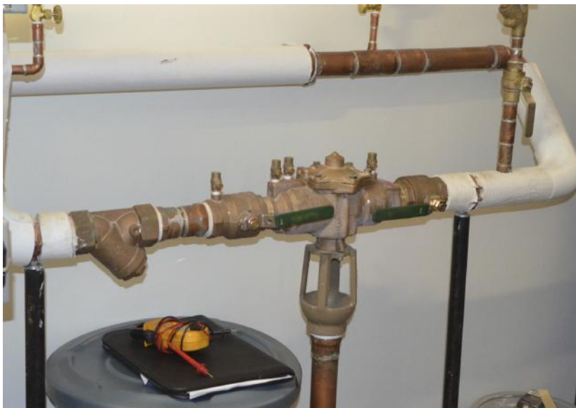
Figure 5.12 Reduced pressure zone principle backflow preventer. (Eddie Van Giesen)
