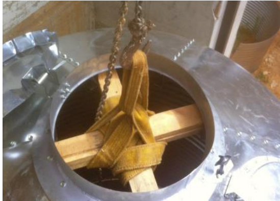
Figure 4.23 Corrugated tank with access opening is attached to the top section of the tank. (Eddie Van Giesen)
