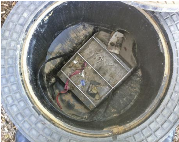
Figures 5.9a and b An example of a cascading type filter when dirty (a) and then after cleaning (b). (Eddie Van Giesen)
