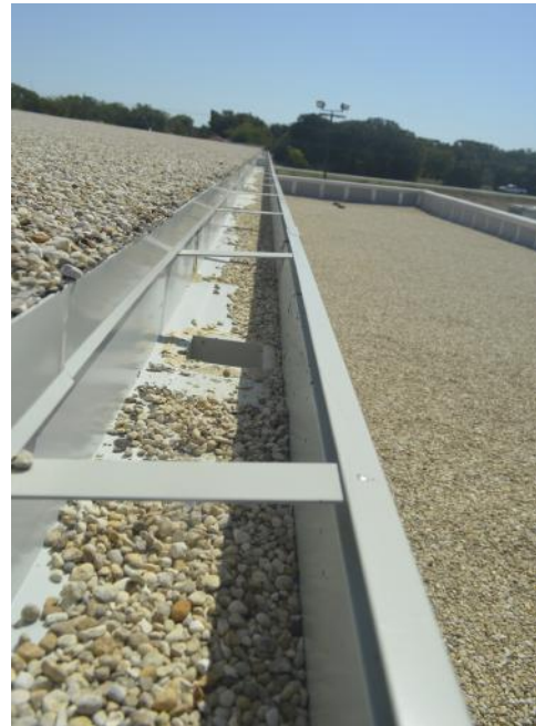
Figure 5.3 Accumulation of gravel in a commercial gutter and built-up gravel roof. (Eddie Van Giesen)
