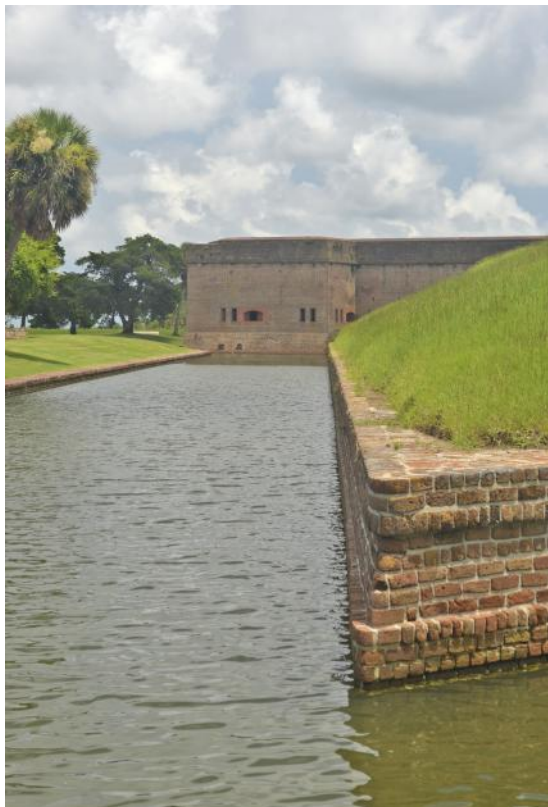
Figure 1.6 Fort Pulaski National Monument in Georgia provides an example of a historic rainwater collection system. Ten brick subterranean cisterns incorporated into the structure of the fort were capable of storing 200,000 gallons of fresh water. After the capture of the Fort, in 1862, Union soldiers supplemented the natural supply with a steam condenser which converted the moat's saltwater into freshwater. ( Eddie Van Giesen )
