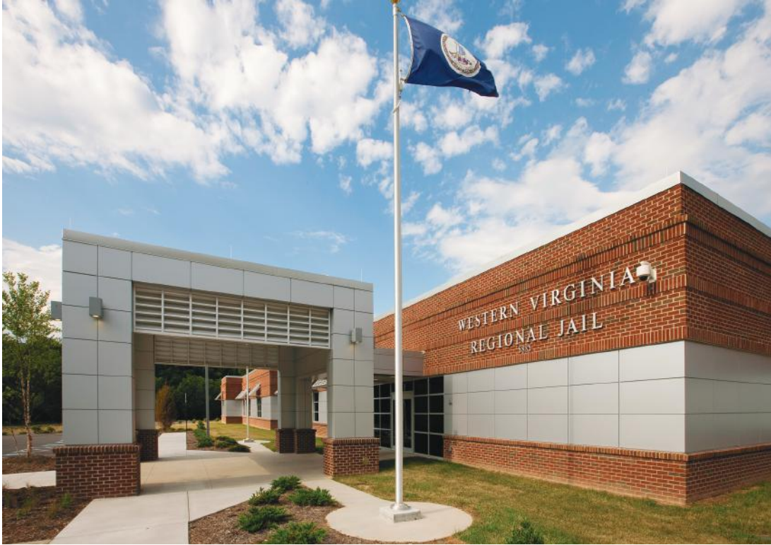
Figure C.4 The West Virginia Regional Jail designed by AECOM uses rainwater for toilet flushing, washing, and irrigation. ( Richard Boyd Photography )
