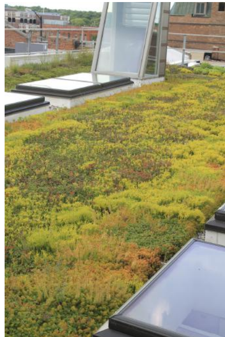
Figure 4.7 Example of a green roof installed by Ann Arbor Architects Collaborative that included rainwater collection for roof irrigation in Michigan. ( Celeste Allen Novak, Architect )
