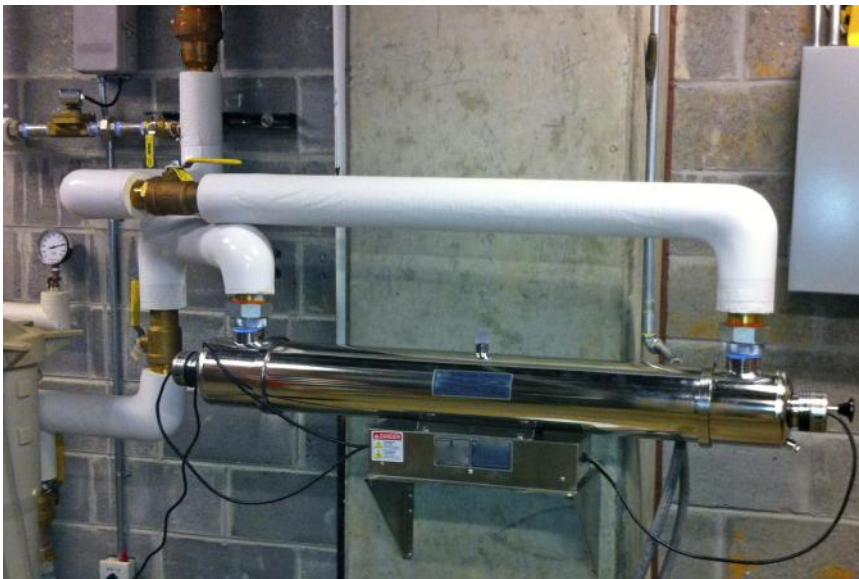
Figure 5.10b Water flow rates and intensity of UV light are matched to achieve disinfection. (Eddie Van Giesen)
