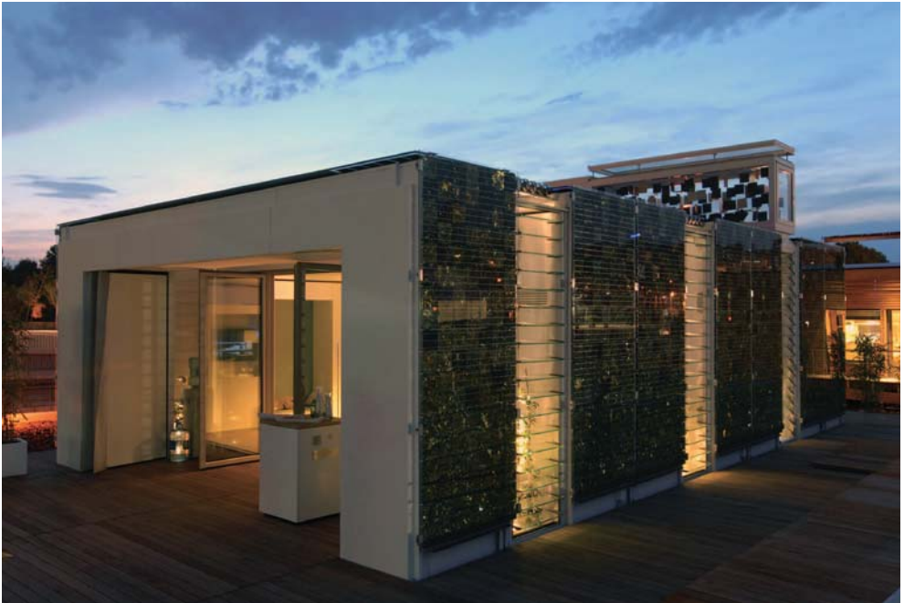
Figure 9.2 Stuttgart Solar Decathlon building home+ with a mono crystalline PVT roof and coloured poly crystalline PV facade elements (photo: Jan Cremers, HFT Stuttgart).
