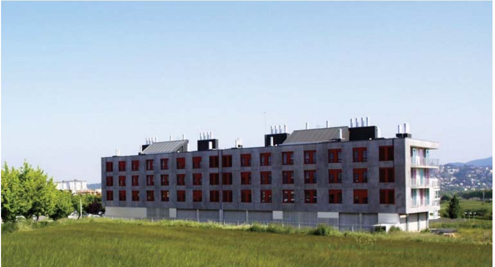
Figure 2.47 The Cerdanyola residential building near Barcelona, Spain under construction (Photo: POLYCITY).
