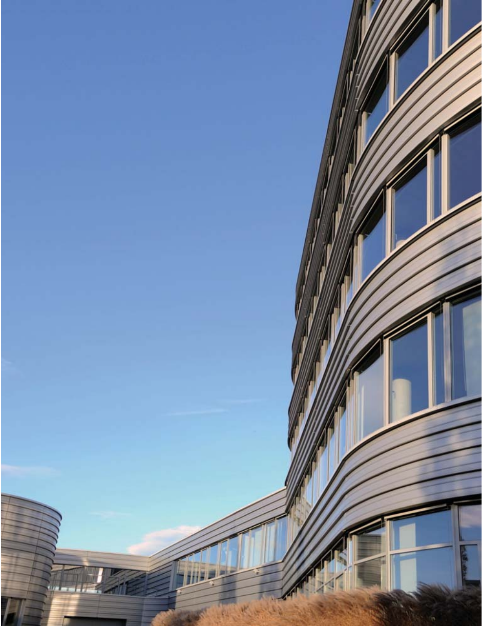
Figure 2.2 Elektror building in Scharnhäuser Park near Stuttgart, Germany with a concrete core activation for an efficient heat and cold distribution (Photo: M. Seubert).
