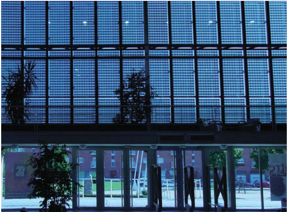
Figure 9.6 Back-ventilated cavity photovoltaic facade of a public library in Mataró (photo: Ursula Eicker).
