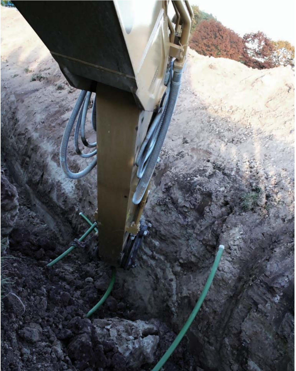
Figure 6.2 Installation of a horizontal low depth heat exchanger in Wüstenrot (Photo: Ursula Pietzsch).
