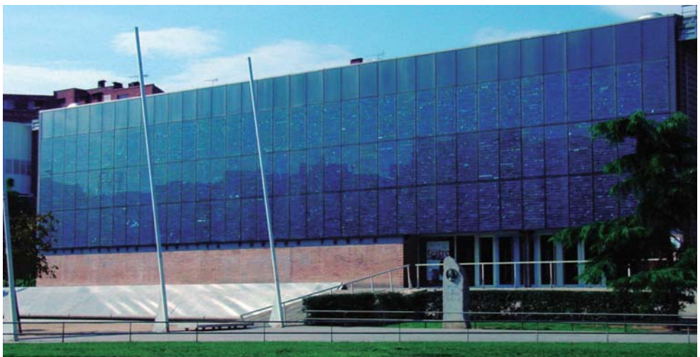
Figure 9.7 Back-ventilated cavity photovoltaic facade of a public library in Mataró (photo: Ursula Eicker).
