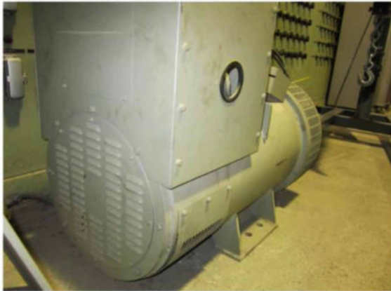
Figure 58. A synchronous generator
