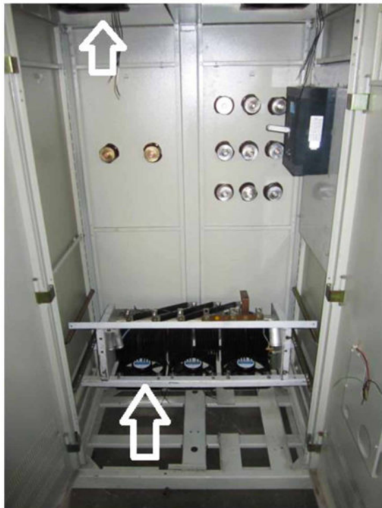
Figure 22. Direction of Fans in a cabinet
