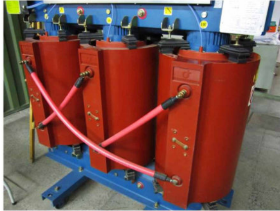
Figure 77. A transformer with resin as insulator
