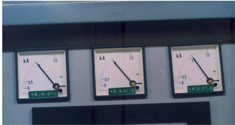
Figure 42. unbalance 3-phase currents
