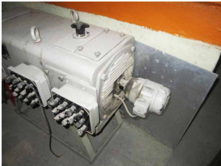
Figure 116. Tachogenerator of a generator
