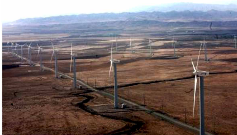
Figure 71. Induction generators used in a wind farm, Source: IRAN SANA (with permission)
