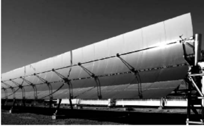
Figure 5.8 Parabolic trough collector of a concentrating solar thermal power plant
