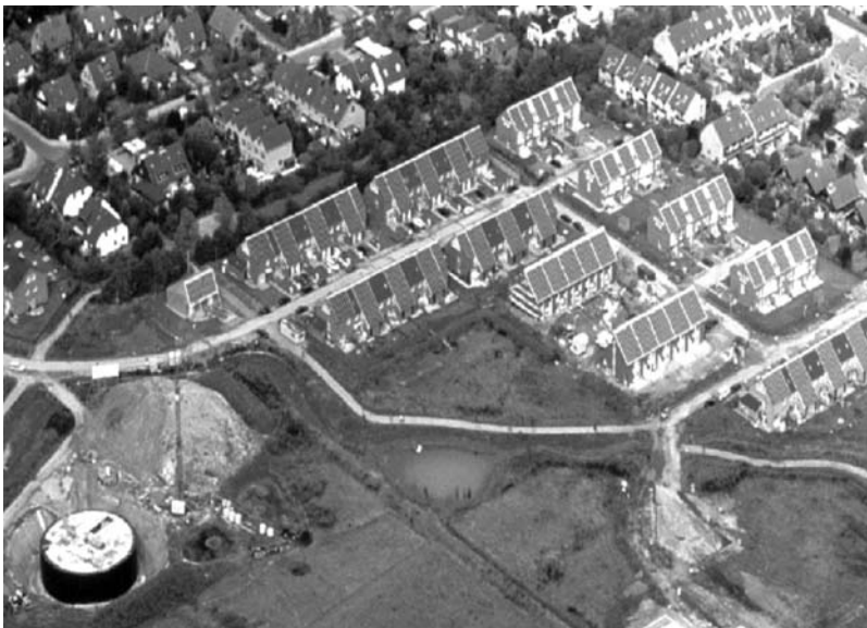
Figure 5.11 Solar-supported local heating network with seasonal storage, for a solar fraction of 50% (the storage system under construction at the lower left corner) (source: Institute of Thermodynamics and Thermal Engineering (ITW), University of Stuttgart, Germany.)
