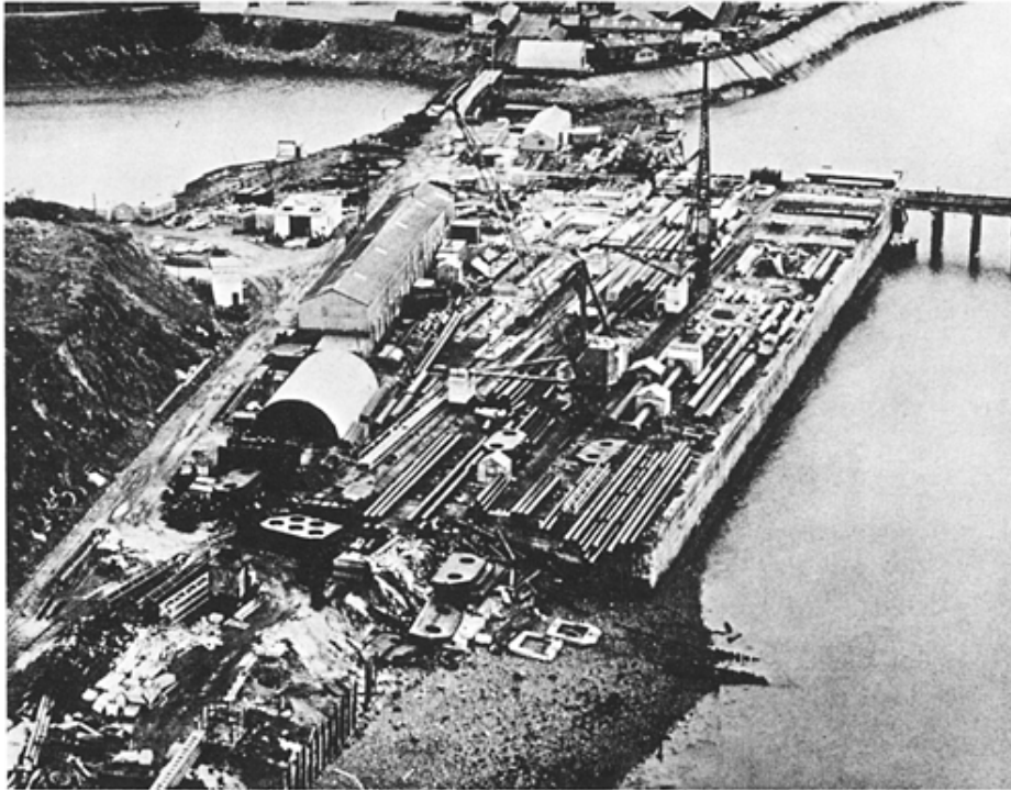
Fig. 2.15 Fabrication yard for steel tubular piles at Milford Haven
