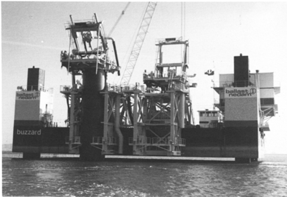
Fig. 9.24 Drilling equipment for sinking 3.50m OD precast concrete cylinder piles, Saudi Arabia-Bahrain Causeway
