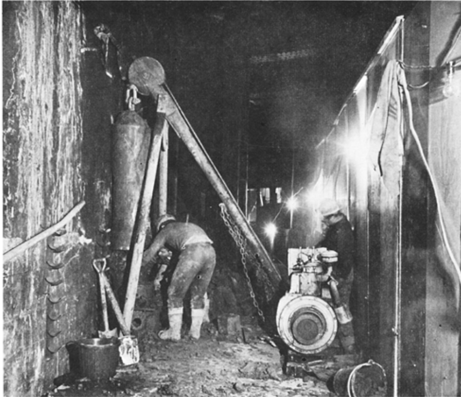
Fig. 3.34 Tripod piling rig installing bored piles under low headroom conditions
