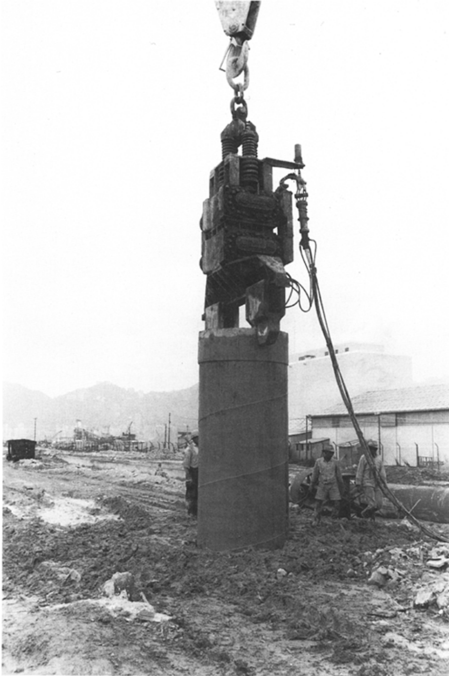
Fig. 3.17 Driving pile casing with Muller vibrator.
