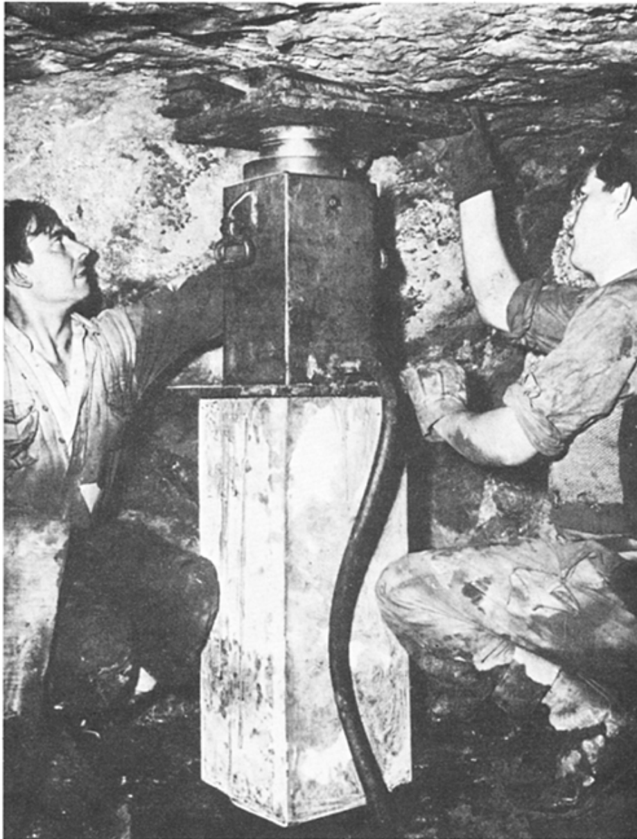
Fig. 9.6 Jacking down Franki Miga pile
