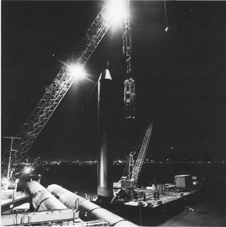
Fig. 3.15 BSP International Foundations Ltd. 40-tonne hydraulic hammer
