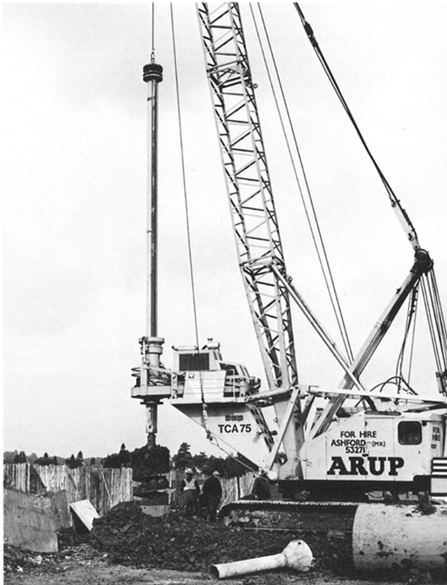
Fig. 3.27 BSP International Foundations Ltd. 'Terradrill' Model TSA75 mounted on standard crawler base machine
