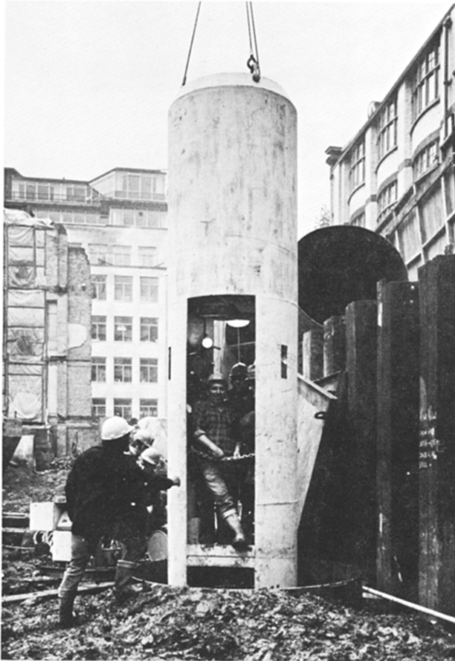
Fig. 11.7 Safety cage used for inspection of pile boreholes
