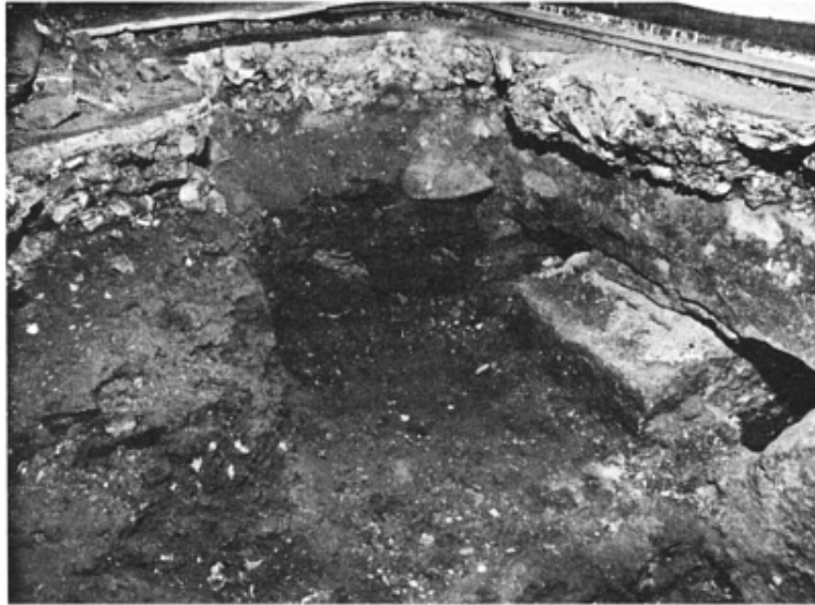
(a) Cavities left by complete decay of piles and timber capping sills
