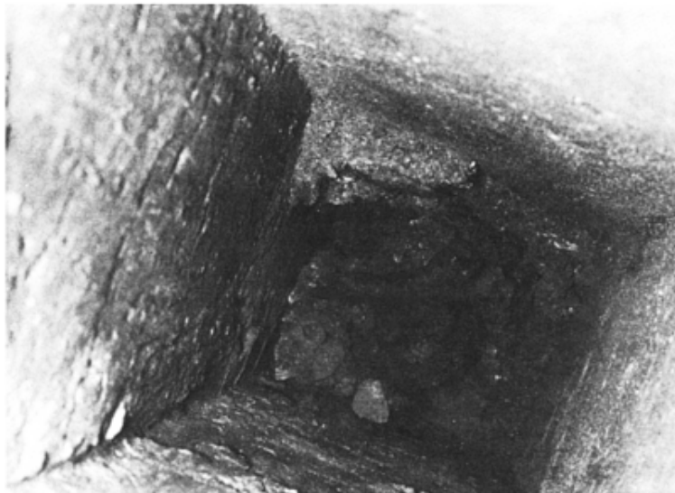
(b) View down cavity left in clay after complete decay of timber pile
