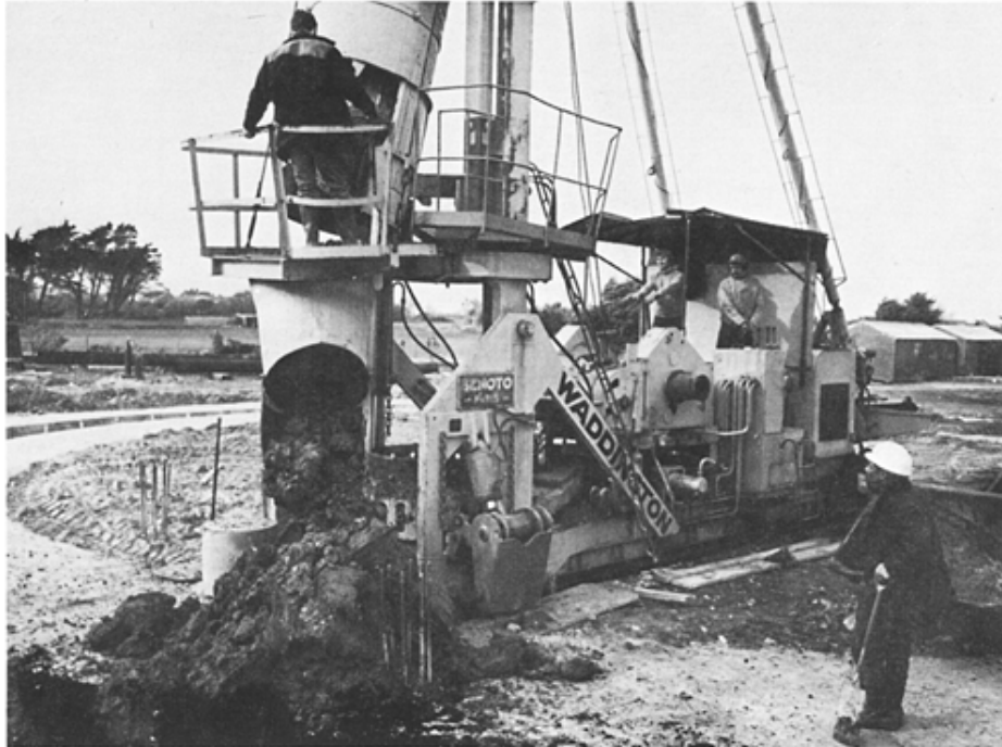
Fig. 3.31 Benoto piling rig showing discharge chute for spoil and casing oscillator at base of machine
