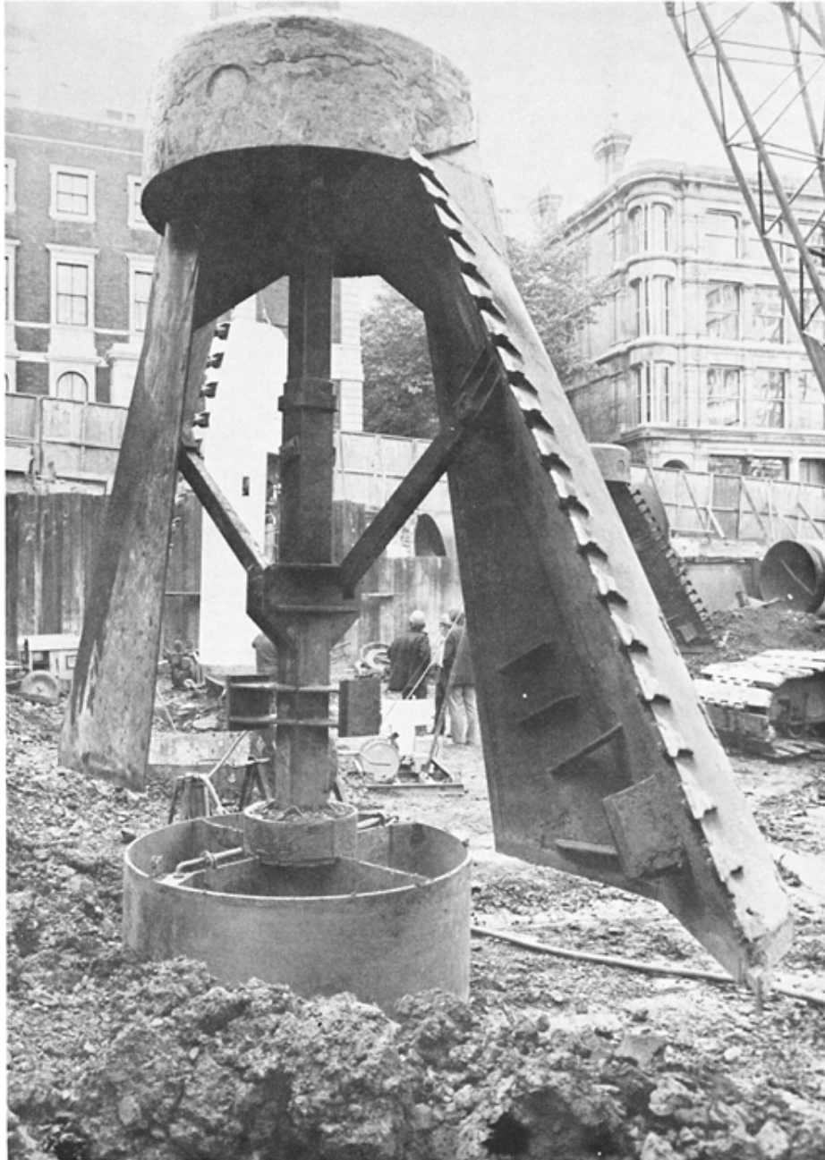
Fig. 3.30 Top-hinged under-reaming bucket
