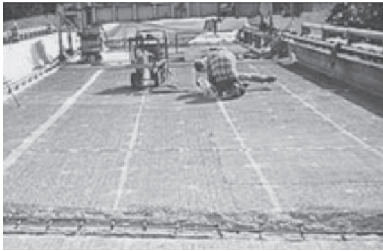
FIGURE 7.15a Fixing an anode on a bridge deck.
