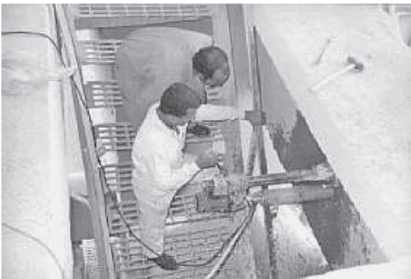
FIGURE 4.5 How to take a core sample.
