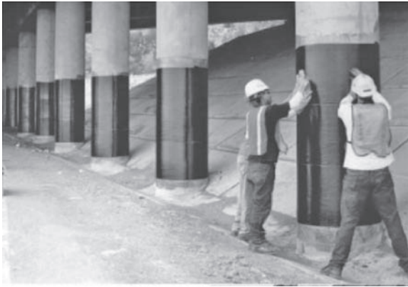
FIGURE 8.27 Column repair.
