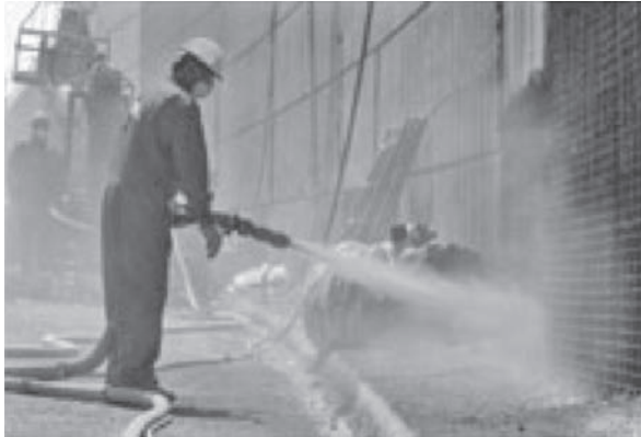
FIGURE 8.16 Using shotcrete.
