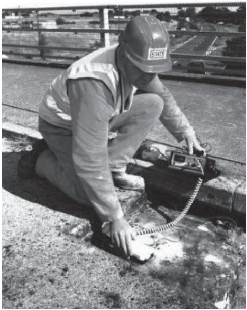
FIGURE 4.22 Concrete cover measurement to a bridge deck.
