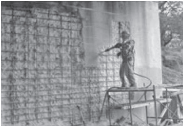
FIGURE 8.3 Using a pneumatic hammer to remove wall concrete cover.
