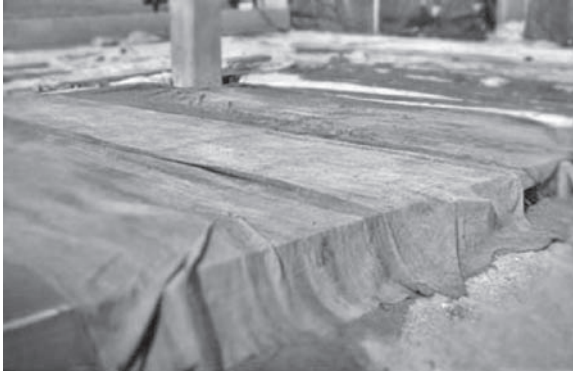
FIGURE 6.16 Curing by using textiles.
