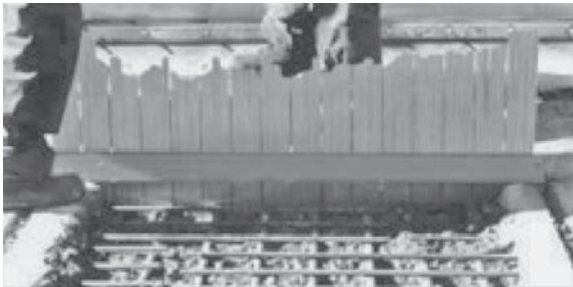
FIGURE 8.6 Surface after using a water jet.
