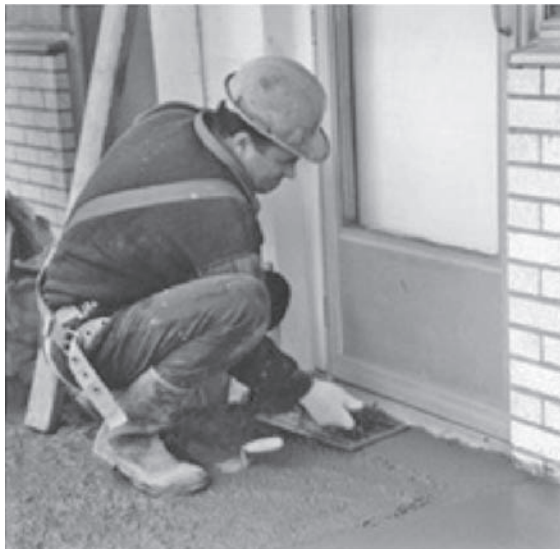
FIGURE 8.13 Manual method for repair.
