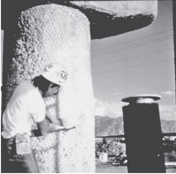
FIGURE 7.11 Fixing titanium on a concrete column.
