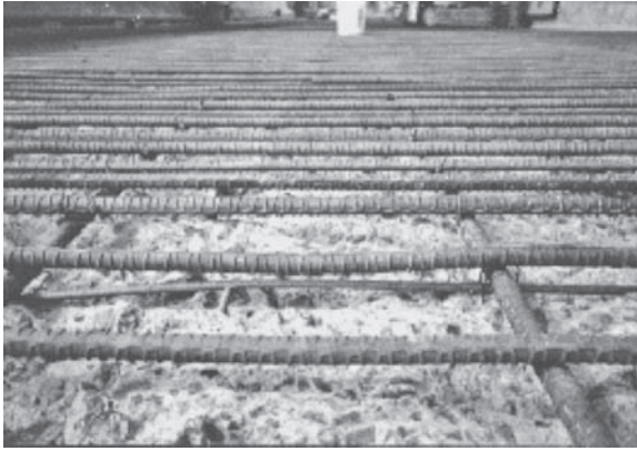
FIGURE 8.5 Concrete surface after using a water jet.
