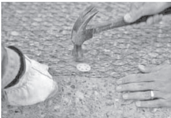
FIGURE 7.15b Fixing titanium mesh by plastic binder.
