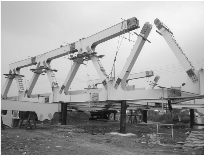
Figure 10.35 Floor beams and bottom lateral bracings of Shang Xin Bridge.
