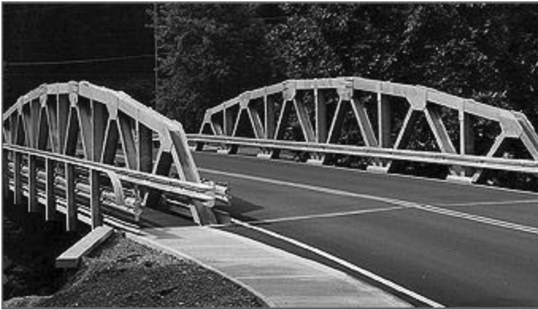
Figure 14.8 Pony truss bridge.
