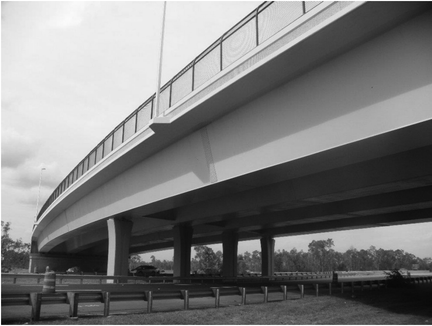
Figure 8.23 Estero Parkway Bridge opened to traffic as a two-span continuous bridge.
