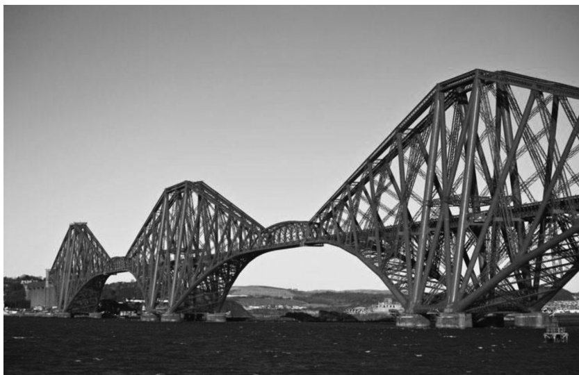
Figure 10.7 Forth Rail Bridge, Queensferry, Scotland.
