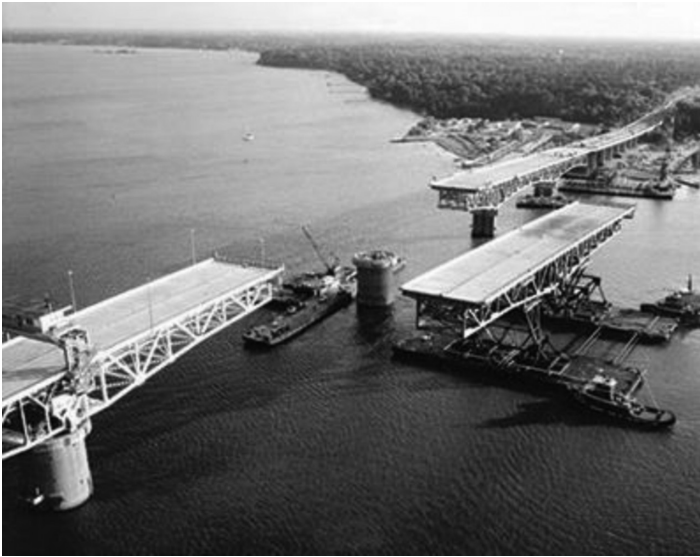
Figure 10.3 Construction of George P. Coleman Bridge in segment. (Courtesy of VDOT, Virginia.)
