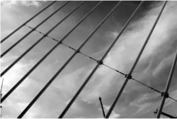
Figure 11.7 Crosstie of cables.
