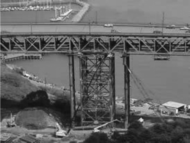
Figure 10.6 The Golden Gate Marin (north) approach viaduct under construction.
