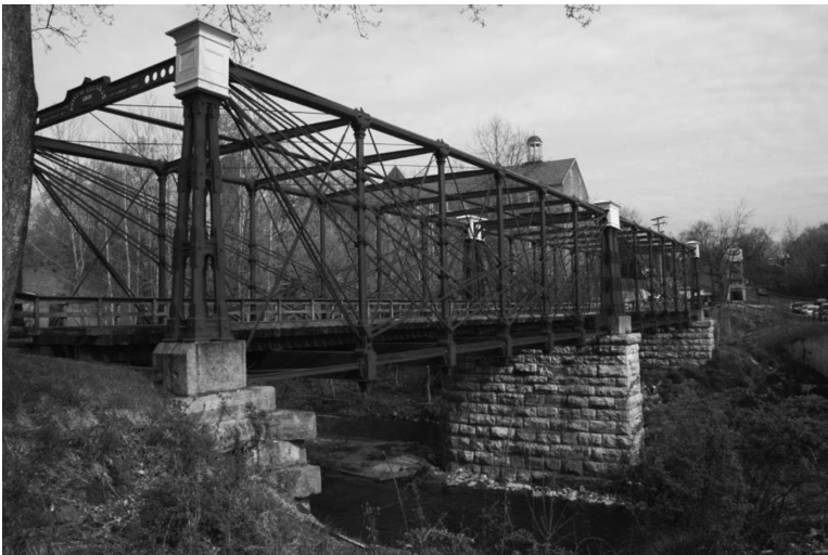
Figure 10.2 Bollman truss bridge.
