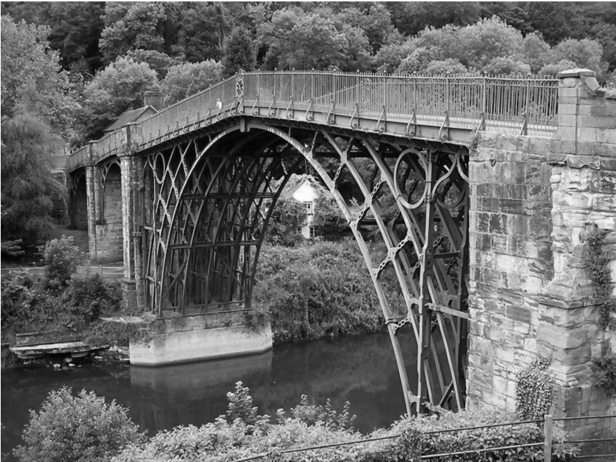
Figure 1.2 The first cast iron truss bridge at Coalbrookdale, Telford, England. (Courtesy of Tata Steel European Limited.)
