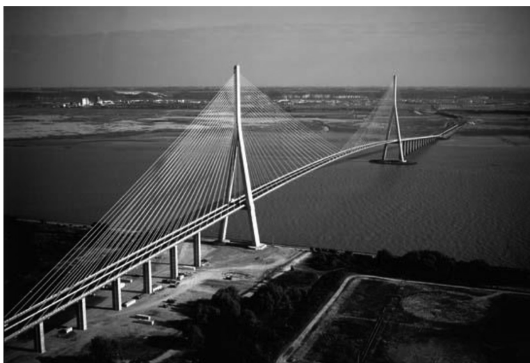
Figure 11.3 A cable-stayed bridge with auxiliary piers.
