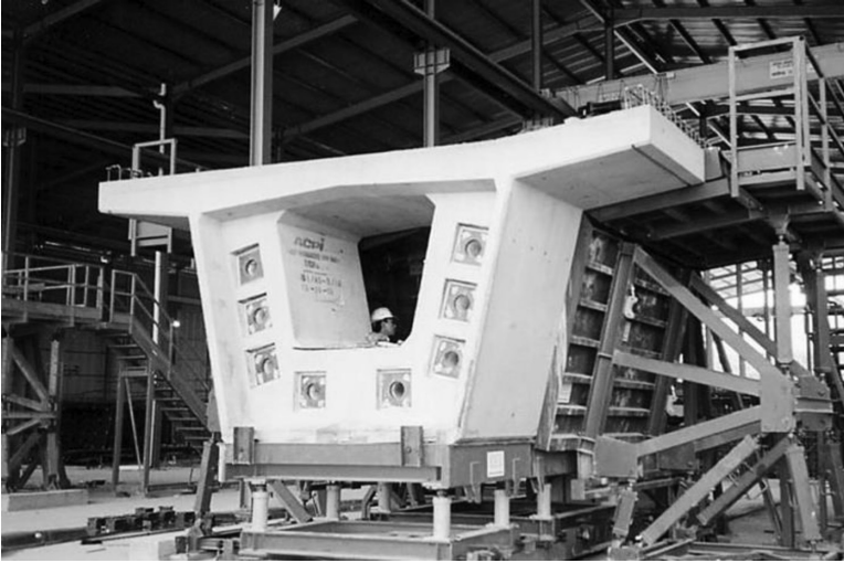
Figure 18.18 Adjustment of match segment and formworks for casting segment. (Courtesy of Ninive™ CASSEFORME, http://www.ninive.it/bridge-formwork/segmental-box-girder-forms/ .)
