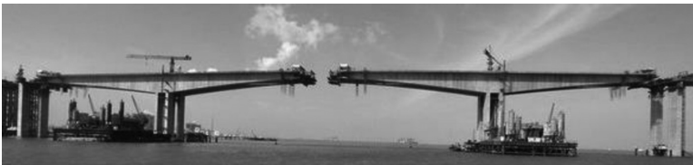
Figure 5.47 Construction of the continuous rigid frame of Sutong Bridge approach spans.
