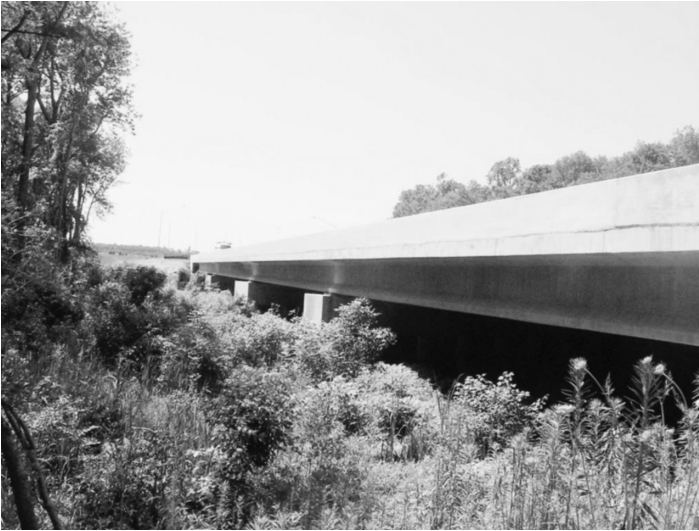
Figure 5.32 US23043 Bridge, Maryland.
