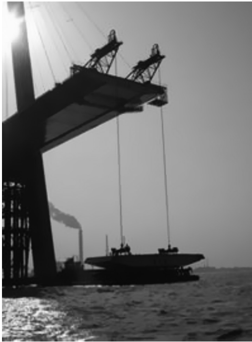
Figure 11.11 Lifting and erecting of one segment.
