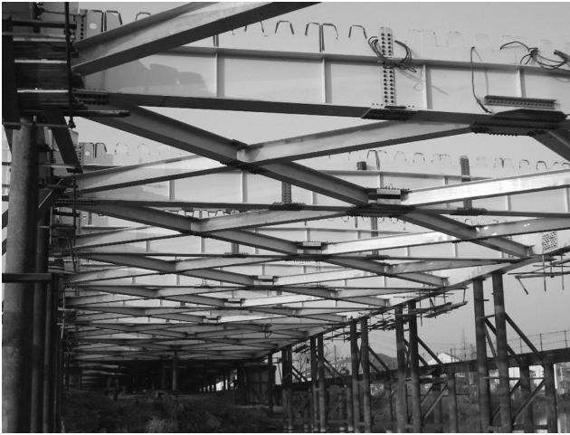
Figure 10.36 Rigid connections of Shang Xin Bridge.
