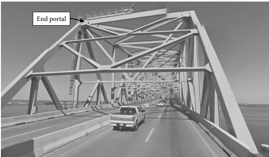
Figure 10.27 End portal of Francis Scott Key Bridge.
