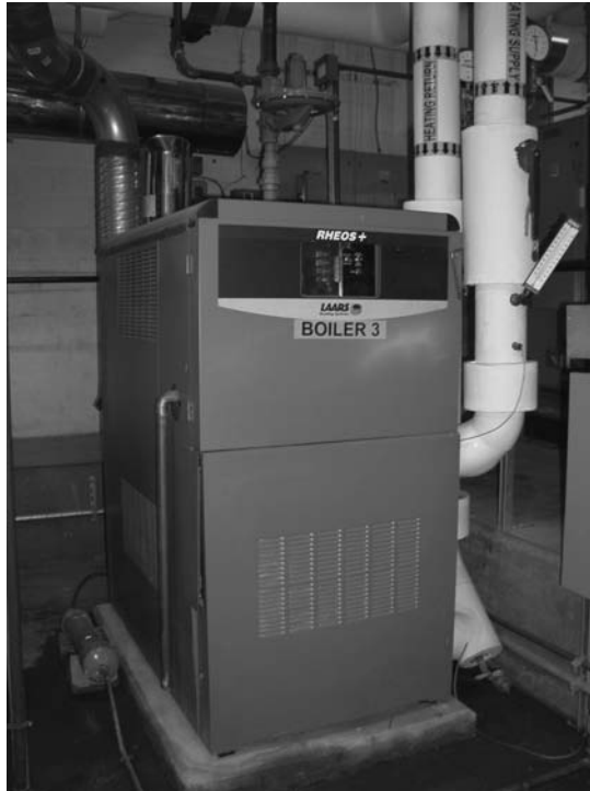
FIGURE 4-2 Photograph of a hot water boiler.
