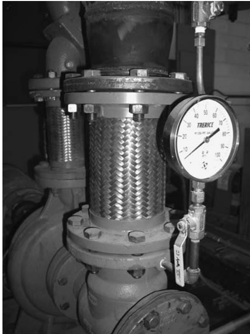
FIGURE 3-38 Photograph of a stainless steel hose and braid flexible pipe connector.
