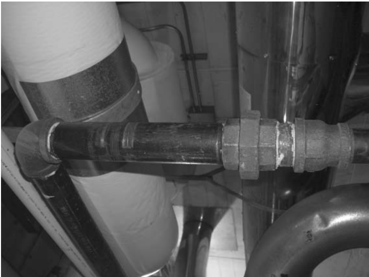
FIGURE 3-2 Photograph of a malleable iron union with threaded ends.
