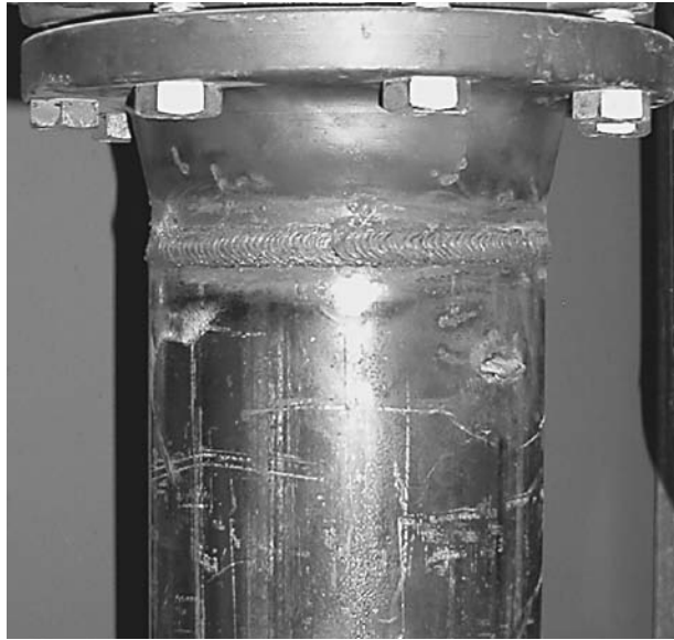
FIGURE 3-3 Photograph of a wrought steel flange with butt welding ends.
