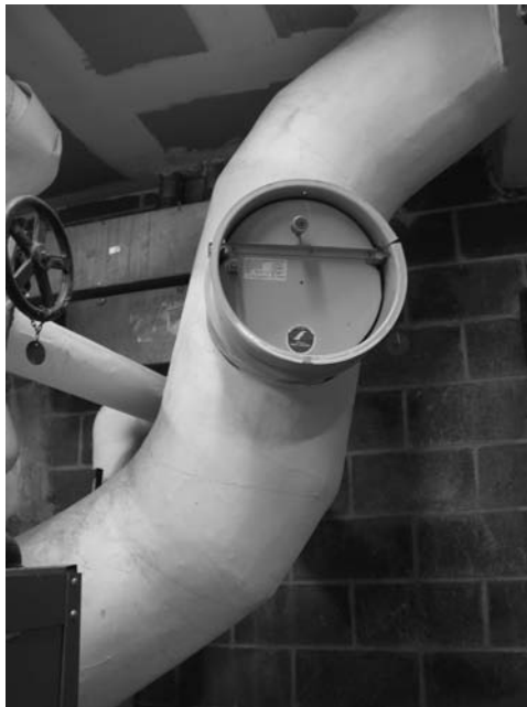
FIGURE 4-5 Photograph of a barometric draft regulator.
