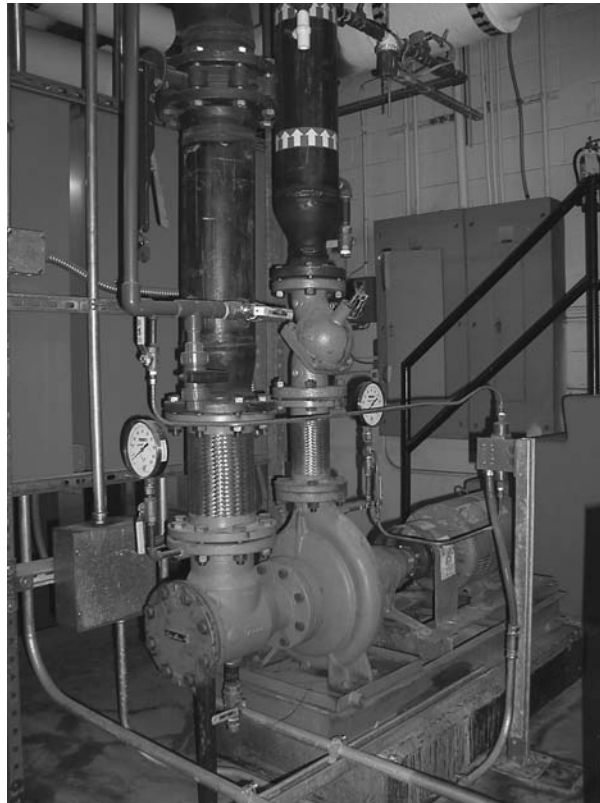
FIGURE 4-31 Photograph of an end-suction pump.
