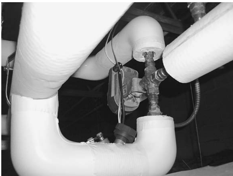
FIGURE 9-5 Photograph of a 3-way globe valve.
