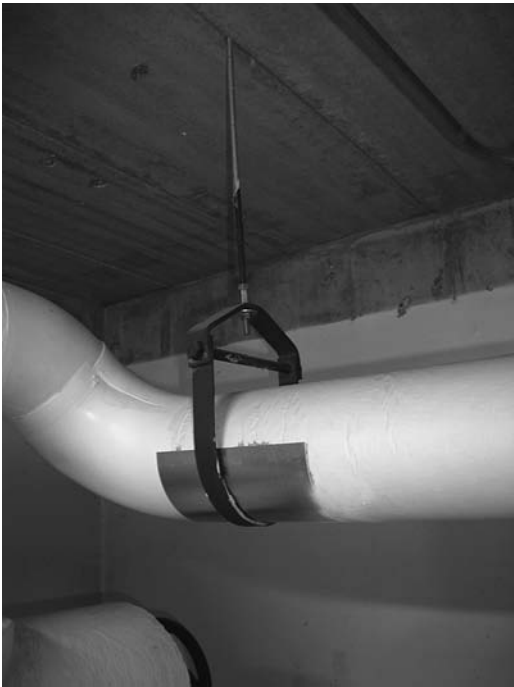
FIGURE 6-2 Photograph of a clevis pipe hanger.
