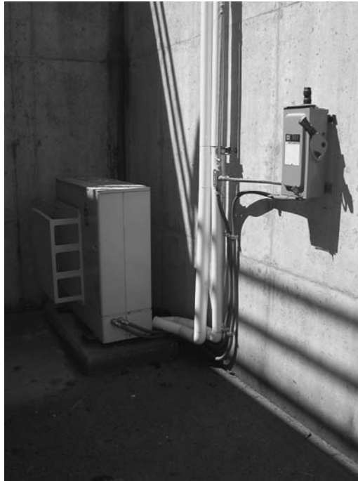
FIGURE 7-12 Photograph of a ductless split-system outdoor unit.
