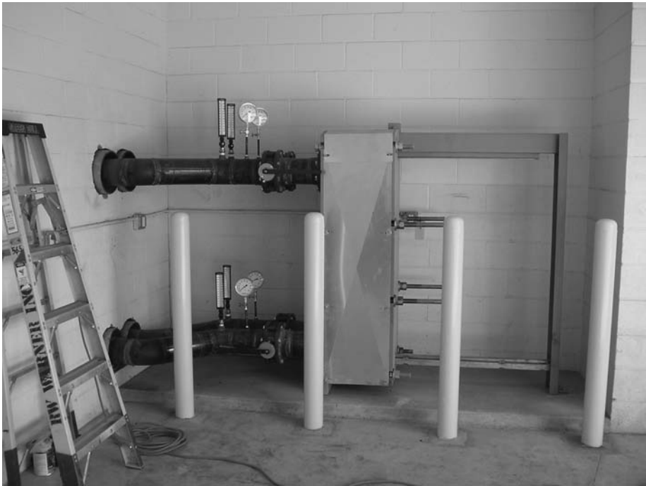
FIGURE 4-8 Photograph of a plate and frame heat exchanger.
