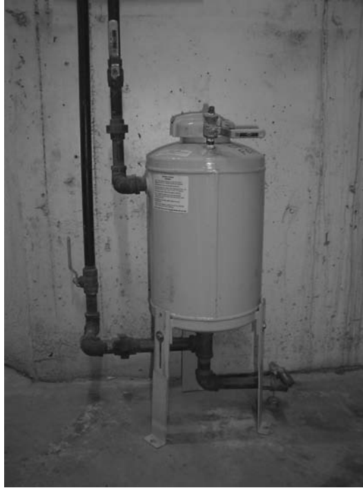
FIGURE 4-23 Photograph of a 5-gal shot feeder.
