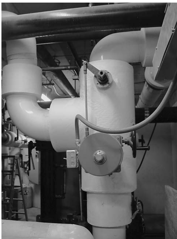
FIGURE 9-6 Photograph of a 3-way butterfly valve.
