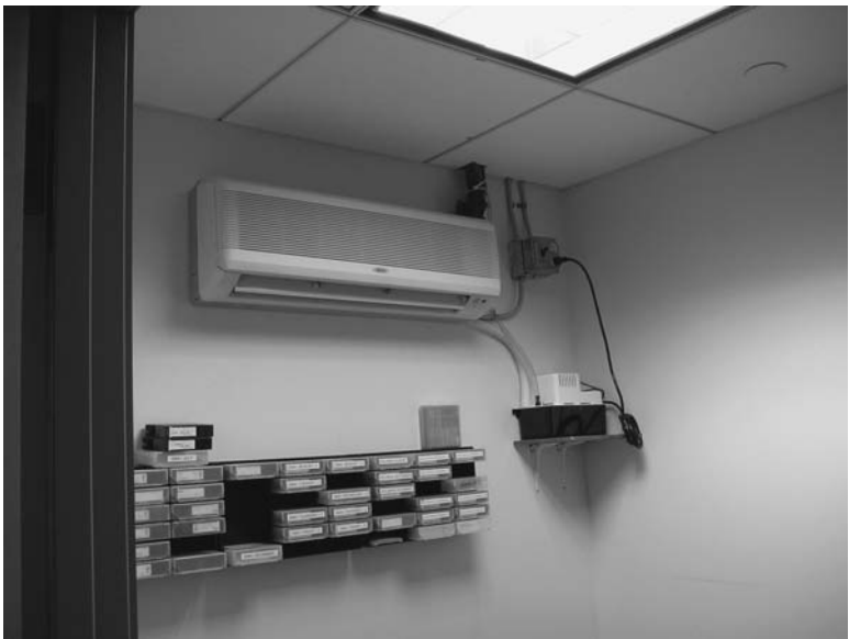
FIGURE 7-11 Photograph of a ductless split-system indoor unit.
