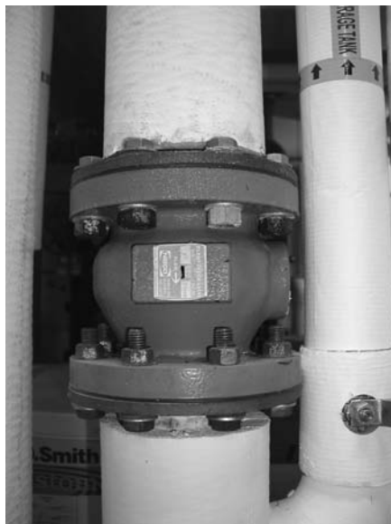
FIGURE 3-23 Photograph of a center-guided check valve with flanged ends.
