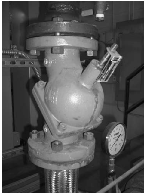
FIGURE 3-24 Photograph of a multi-purpose valve with flanged ends.
