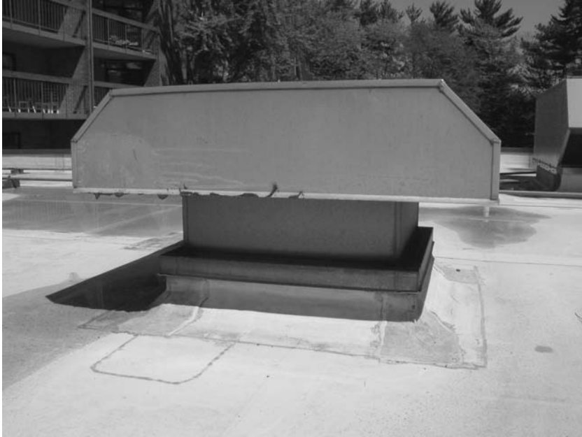
FIGURE 2-9 Typical intake/exhaust/relief air hood.
