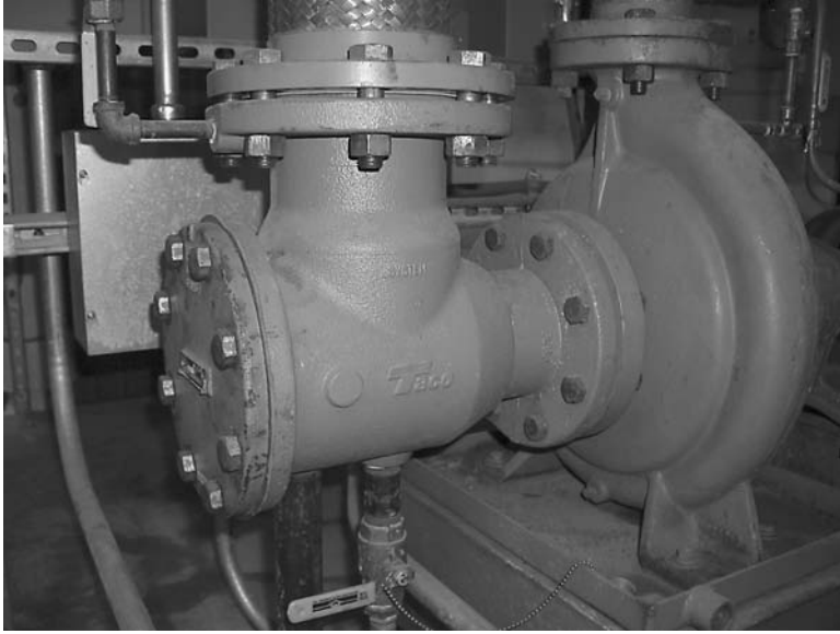
FIGURE 3-36 Photograph of a suction diffuser.
