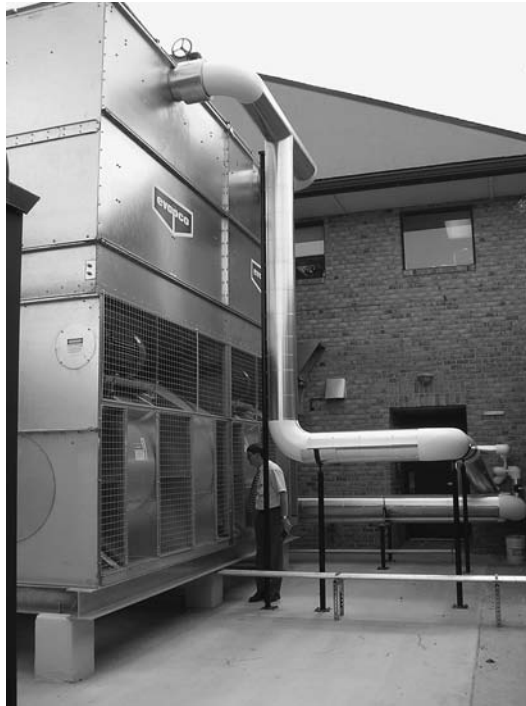
FIGURE 4-17 Photograph of a forced draft counterflow cooling tower.
