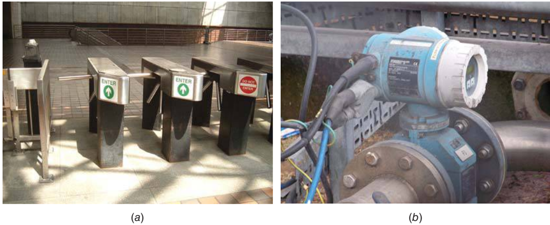
Figure 24.2 Monitoring the Use of Systems: (a) Monitoring the frequency of use: Turnstiles at transit terminals help transit agencies to keep accurate counts on the extent of use of their systems. (b) A magnetic flow meter at the Tetley's brewery in Leeds, West Yorkshire, as seen from Crown Point Road. The meter is manufactured by 'Endress + Hauser' and is tagged 'F1' ('F' denoting flow). The meter used HART Protocol. Taken on the afternoon of Monday the 10th of May 2010. [Courtesy: (a). Arnold Reinhold/Wikimedia Commons and (b). Mtaylor848/Wikimedia Commons].
