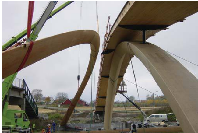
Bridge under construction, 2001, Vebjorn Sand, Norway.
