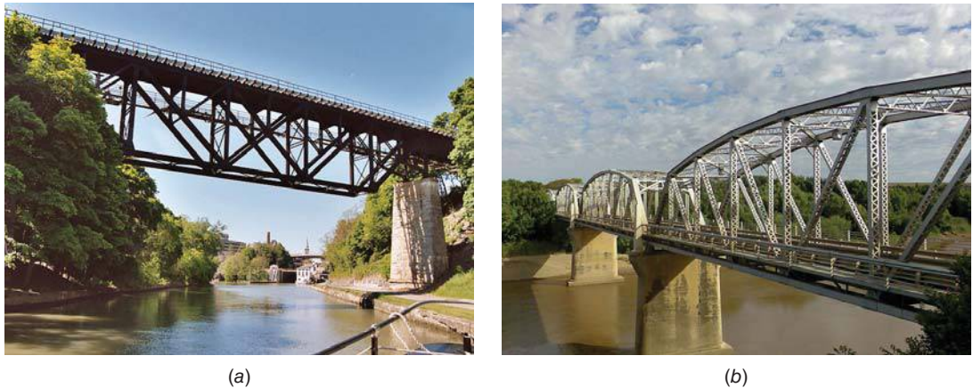
Figure 21.1 Different configurations in design: illustration using bridge truss example: (a) truss located beneath bridge and (b) truss located above bridge (a. Courtesy of Leonard G./Wikimedia Commons; b. Gregory David Harington/Wikimedia Commons).
