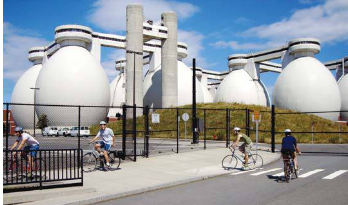
Figure 1.11 Digesters at the wastewater treatment plant Deer Island, MA (Source: Frank Hebbert/Wiki Commons).
