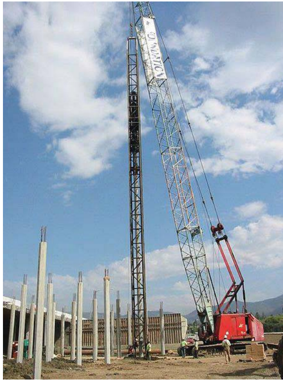
Figure 19.5 Special geotechnical systems are needed in areas of weak soils. Pile driving for a bridge in California (Courtesy of Argyriou/Wikimedia Commons).
