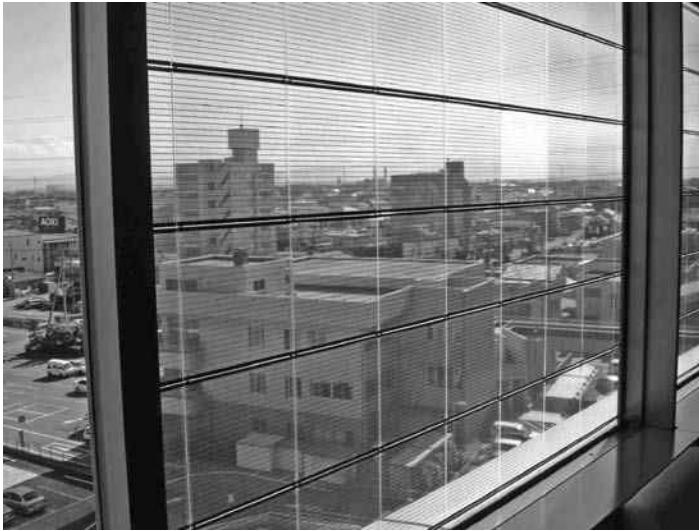
FIGURE 8.11 Building integrated see-through PV modules (Sanyo) at the Ohta City government office complex.
