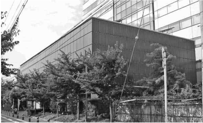
FIGURE 8.14 Sanyo corporate headquarters in Tokyo with BIPV on the south, east, and west sides of this office complex.
