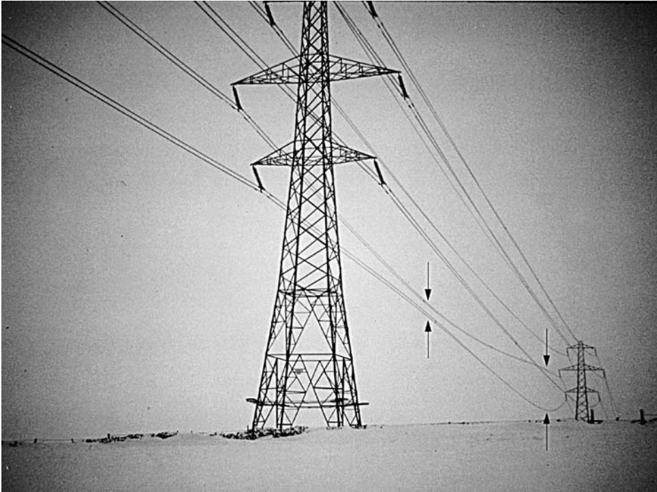
Figure 3.40 Galloping lines. The arrows indicate the minimum distance (when there is a risk of a short-circuit) and the maximum distance between the conductors. Reproduced by permission of M. Tunstall.
