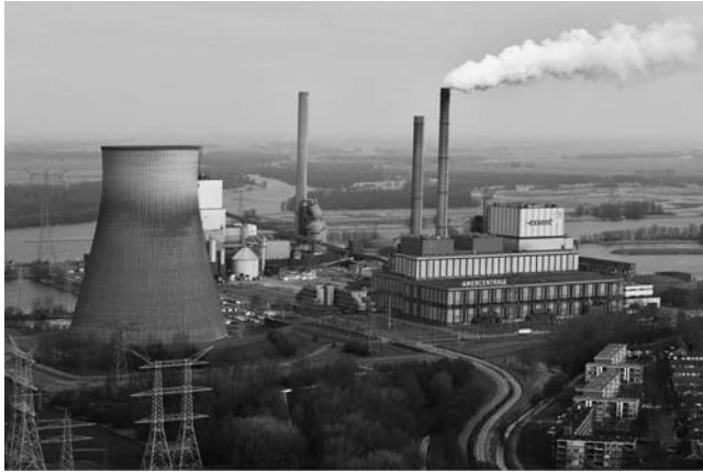
Figure 2.1 A thermal power plant. Reproduced by permission of TenneT TSO B.V.
