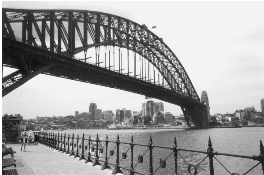
Fig. 2.51 Sydney Harbour Bridge.
